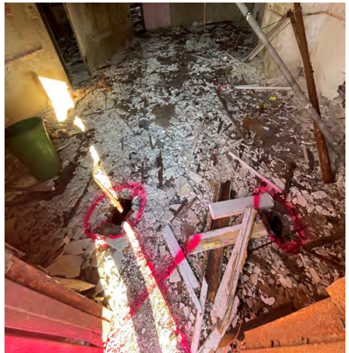
Photo 8: 1st floor punch through under inspector's weight.
