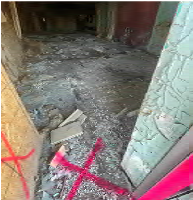
Photo 7: Front Door (Inaccessible). Floor flex under inspector's weight.
