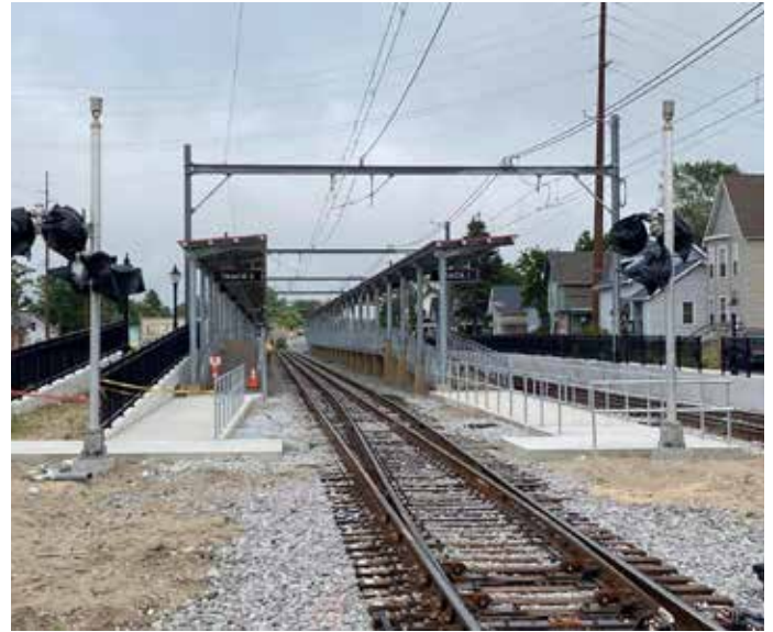
Construction of South Shore Double Track Project in Michigan City
