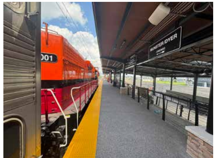
New West Lake Corridor Station
