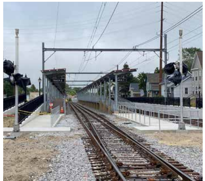
Construction in Progress at Michigan City 11th Street Station
