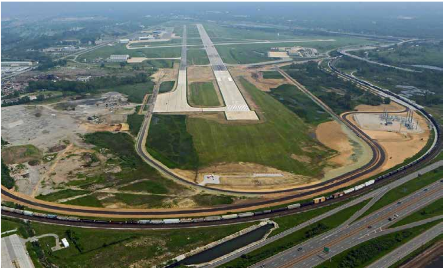
Runway Expansion Project at Gary/Chicago International Airport
