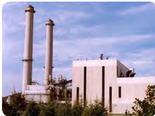
Power boiler natural gas conversions are currently an attractive and economical option.
