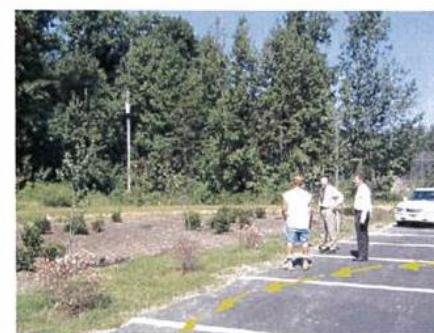
Some site runoff by-passes bioretention because of inadequate slope of filter strip.
