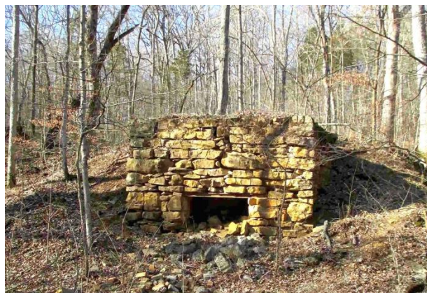
Image 26 . This is one of the two surviving lime kilns on a hillside in Spring Mill State Park between the lake and the railroad.
