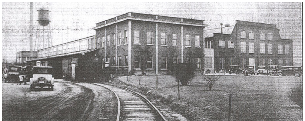
The Guide Plant No. 1 in Anderson, Indiana
