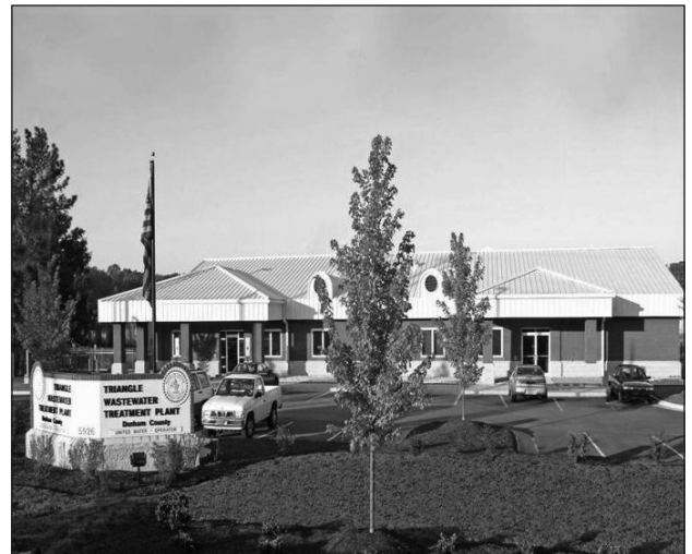
Triangle Wastewater Treatment Plant Photo courtesy of Durham County Engineering Department
