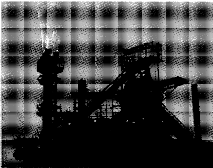
Prior to the installation of the energy recovery boiler, 46 billion cubic feet of BFG was flared into the atmosphere each year. Photo courtesy of ArcelorMittal
