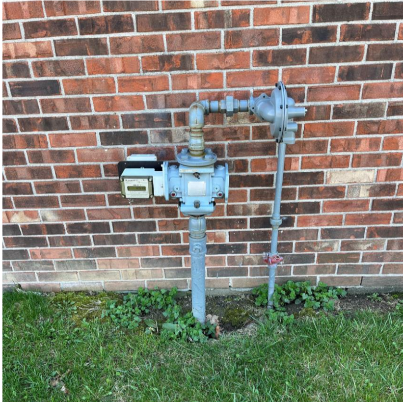
Master meter served from the gas supplier.
