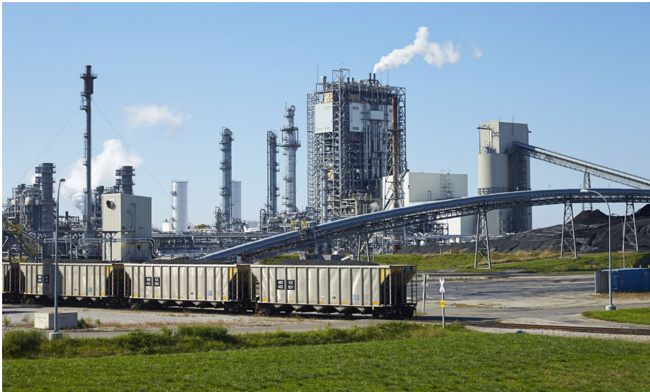
Edwardsport Generating Station
