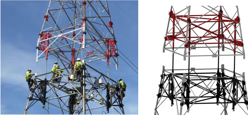
Figure 17: AMPJACK lift system.
