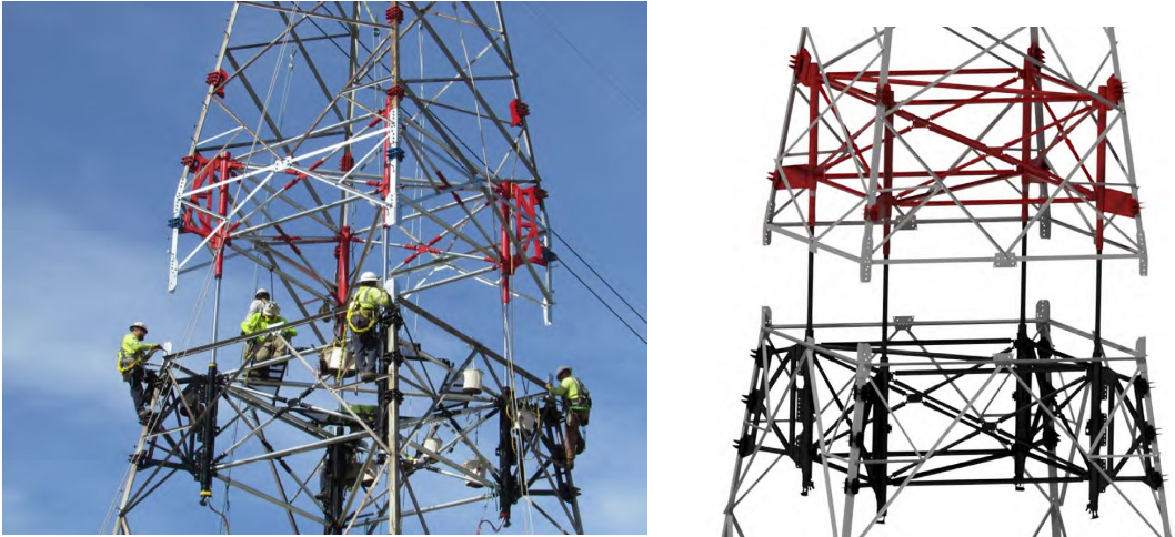
Figure 17: AMPJACK lift system.
