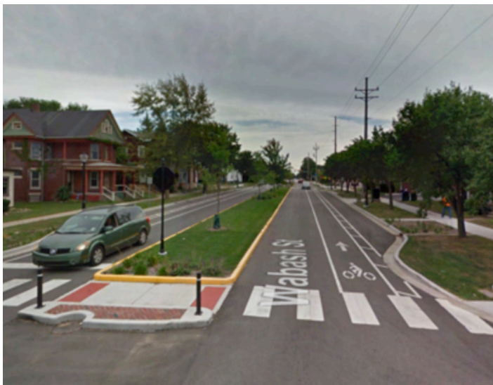
Bike lanes, green medians and native plantings were added during the Michigan City Wabash Street Improvements project.
