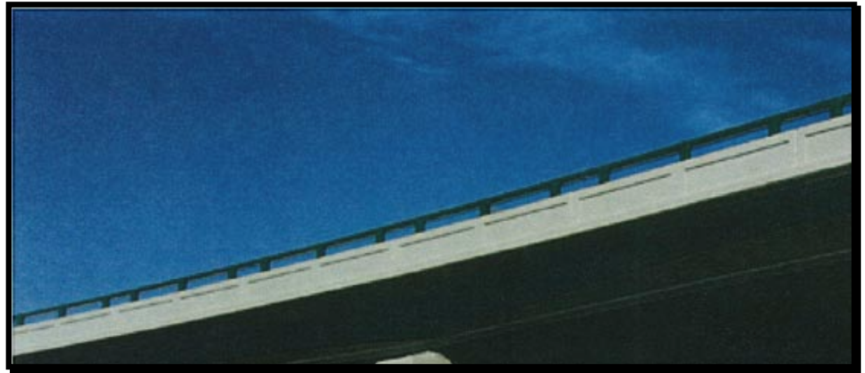
Type of Bridge Railing
