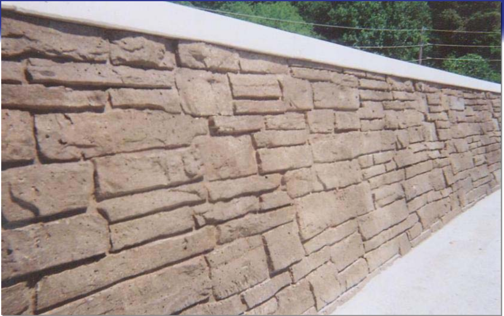
Texture of the Retaining Walls & Bridge Piers
