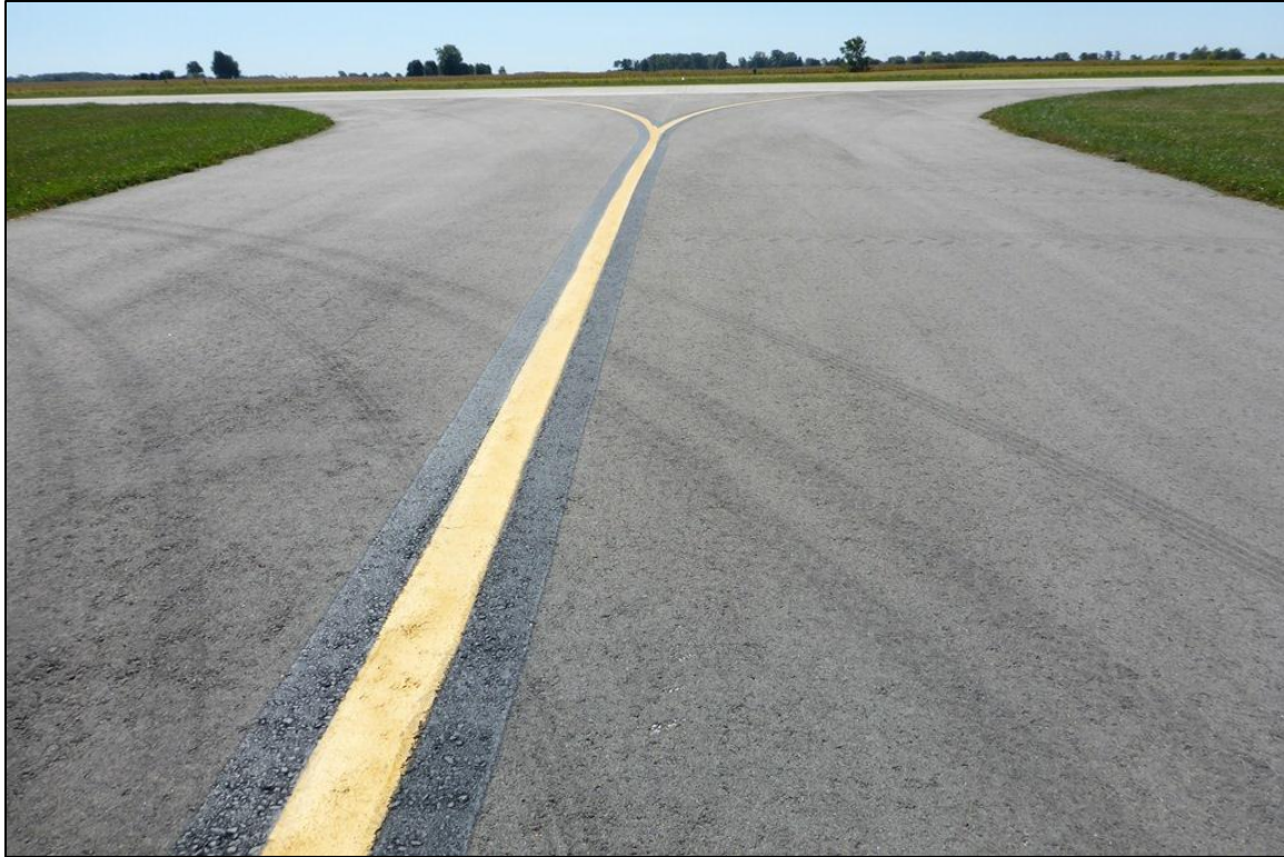
Figure 2-4. Typical AC Pavement in Good Condition (Feature 165)
