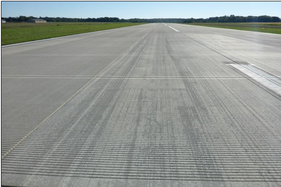
Figure 2-3. Typical PCC Pavement in Good Condition (Feature 6105)
