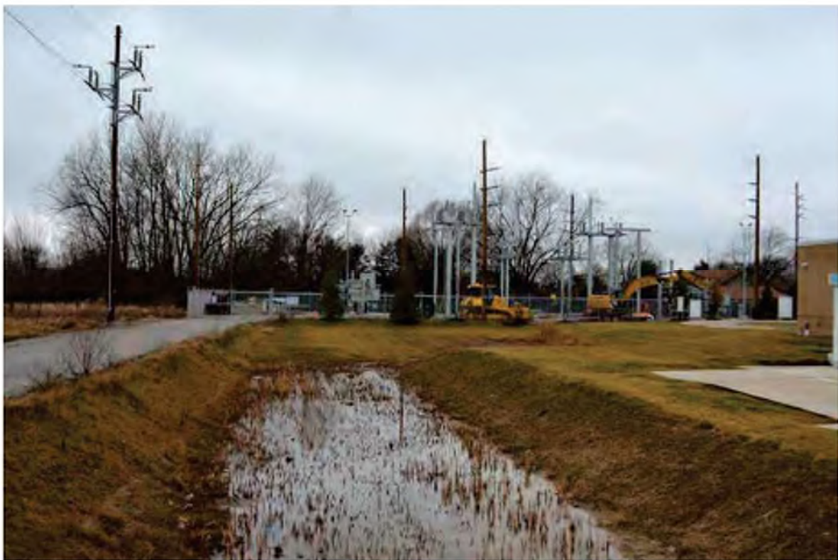
12. The Northern Indiana Public Service substation has had an additional entrance added along Parrish Avenue at the south end of the APE, looking west.
