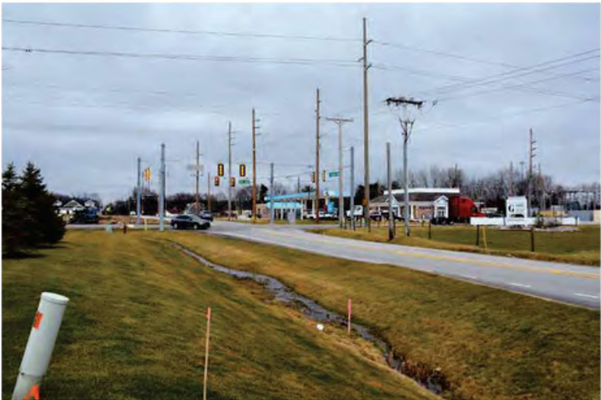
4. This view looks south at the intersection of US 231/109th Avenue and Parrish Avenue.
