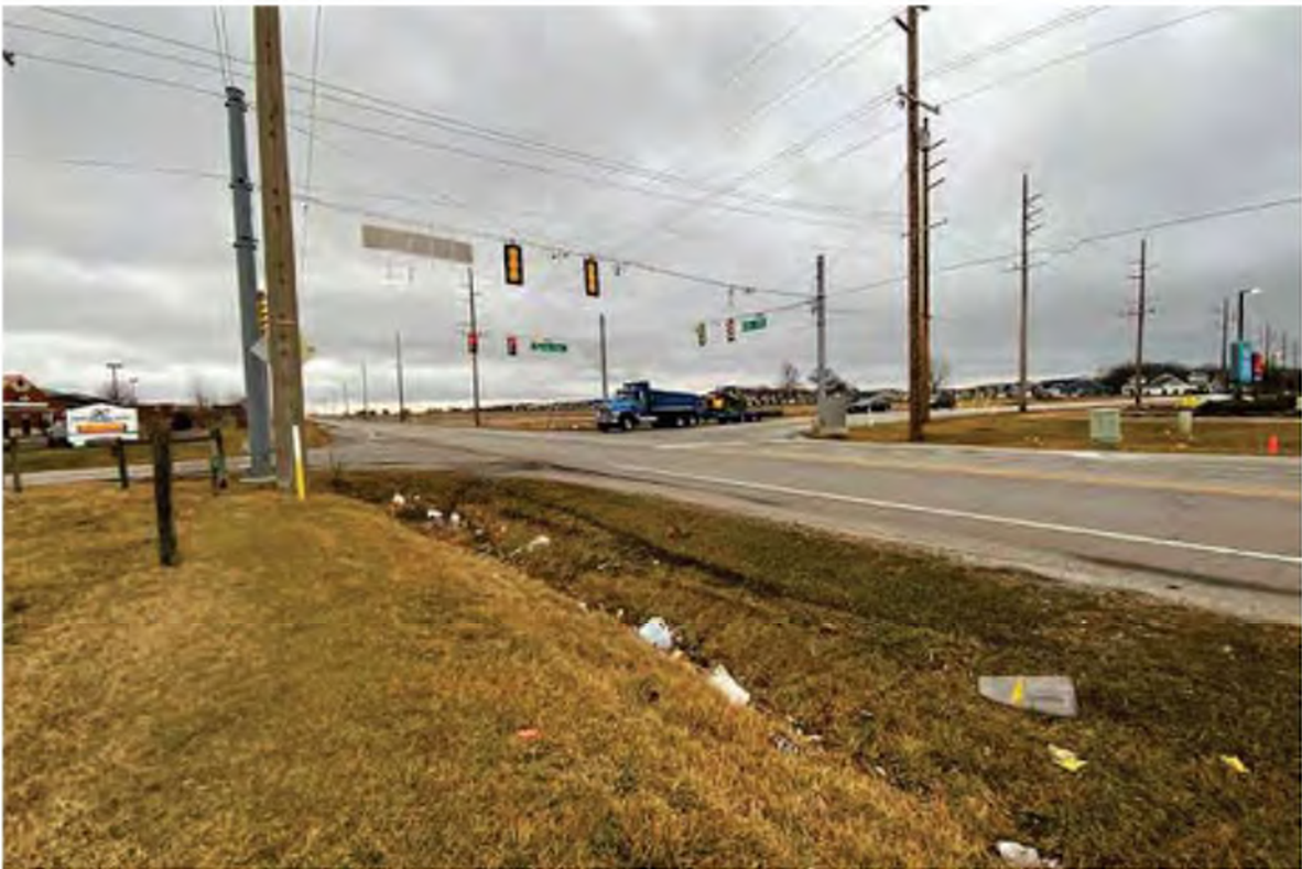
7. The project would replace the current signalized intersection of US 231/109th Avenue and Parrish Avenue with a roundabout, looking southeast.
