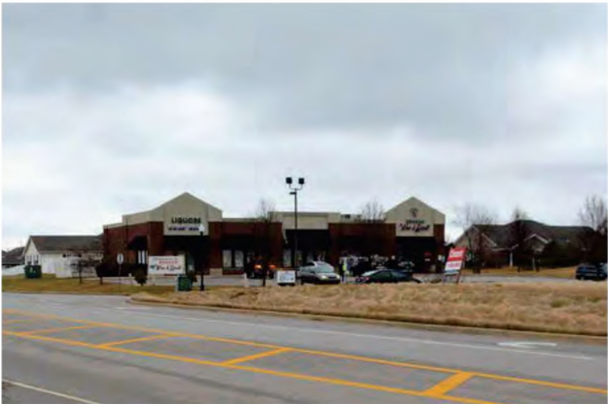
3. Commercial properties have developed within the APE, including the liquor store located at 9540 Poplar Place, looking northeast.
