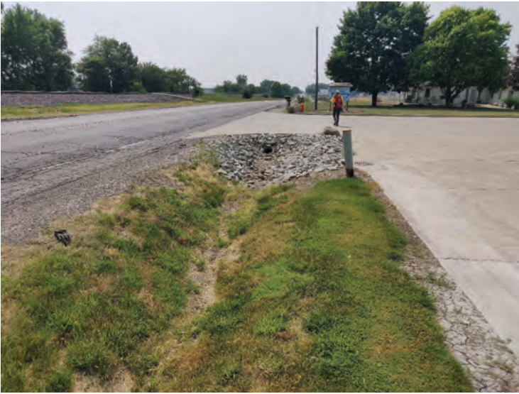
37. Looking west along north side of US 6 toward culvert
