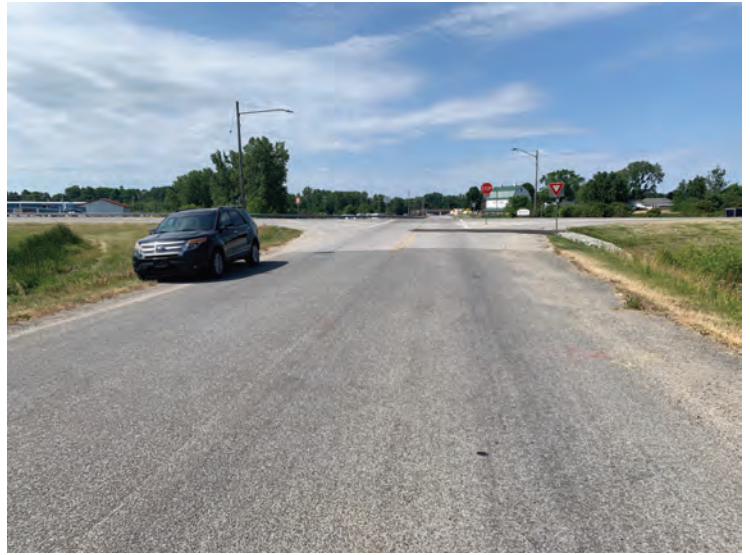
2. Looking southwest along Douglas Rd toward US 6
