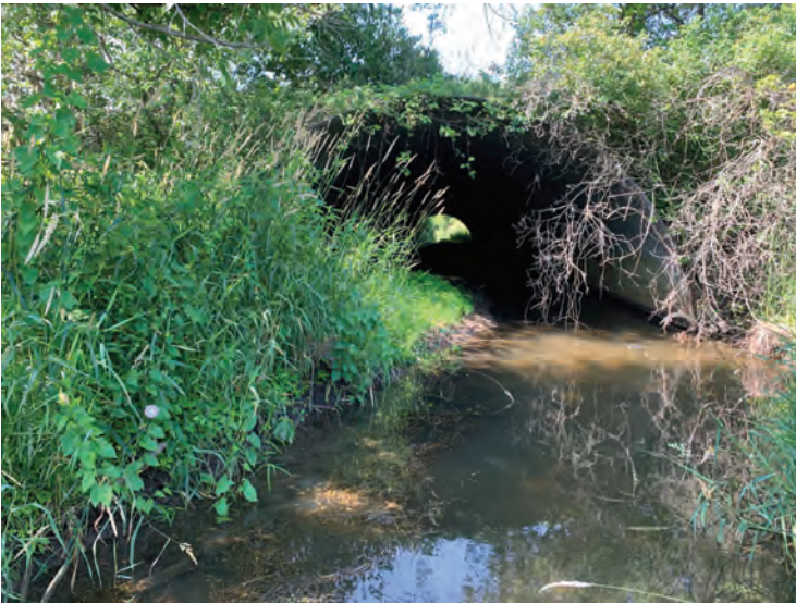
3. Looking south downstream along Albert Zeiger Ditch toward culvert
