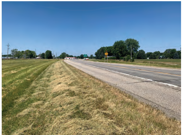
6. Looking northwest along south side of US 6
