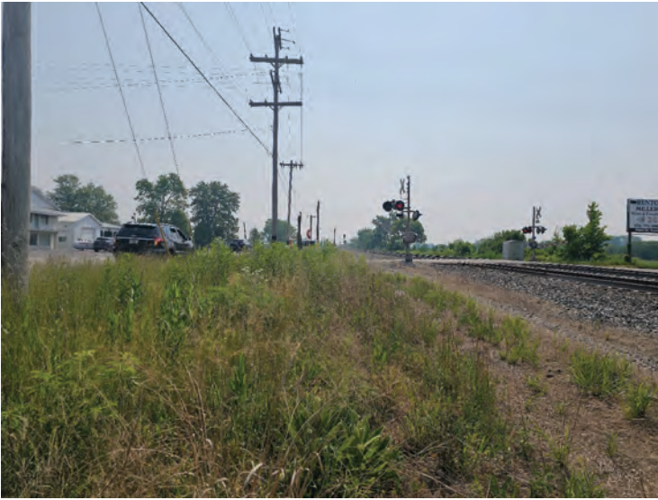
25. Looking east along south side of US 6
