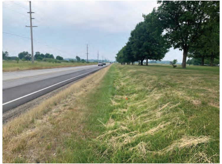
14. Looking west along north side of US 6
