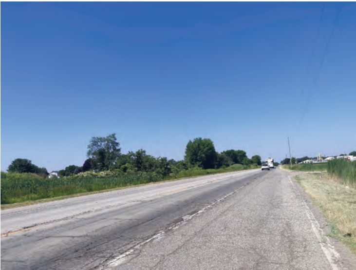
39. Looking west along north side of US 6
