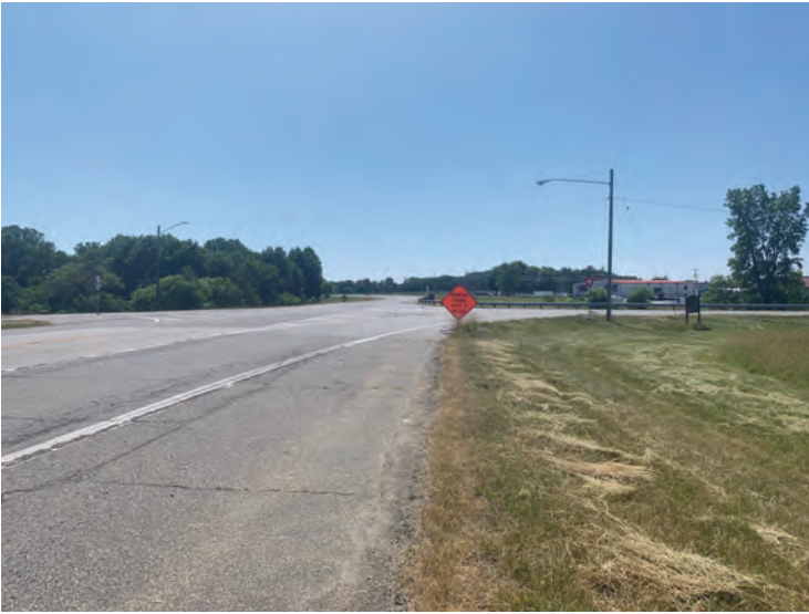
1. Looking southeast along US 6
