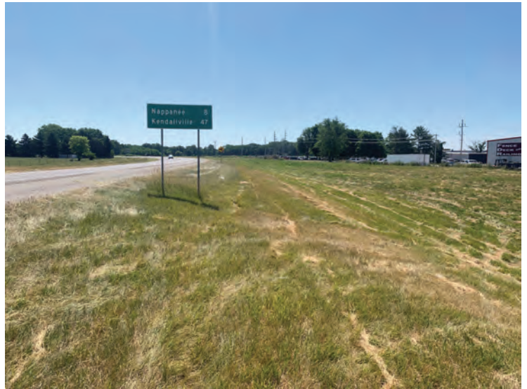
4. Looking southeast along south side of US 6
