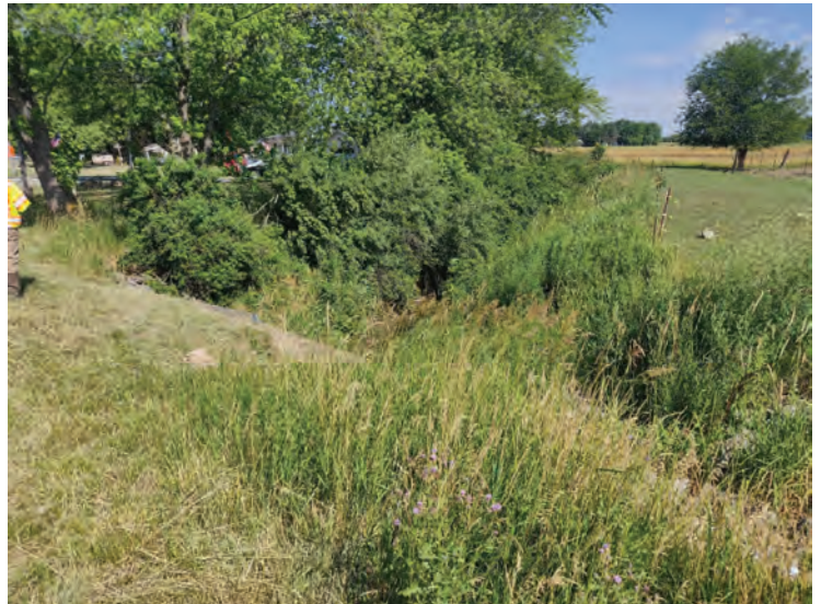
12. Looking northwest downstream along George Marberger Ditch
