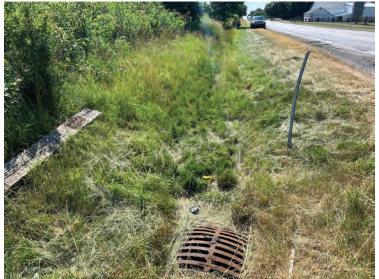
34. Looking west along south side of US 6 at drainage structure
