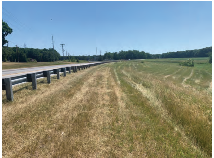
16. Looking east along south side of US 6
