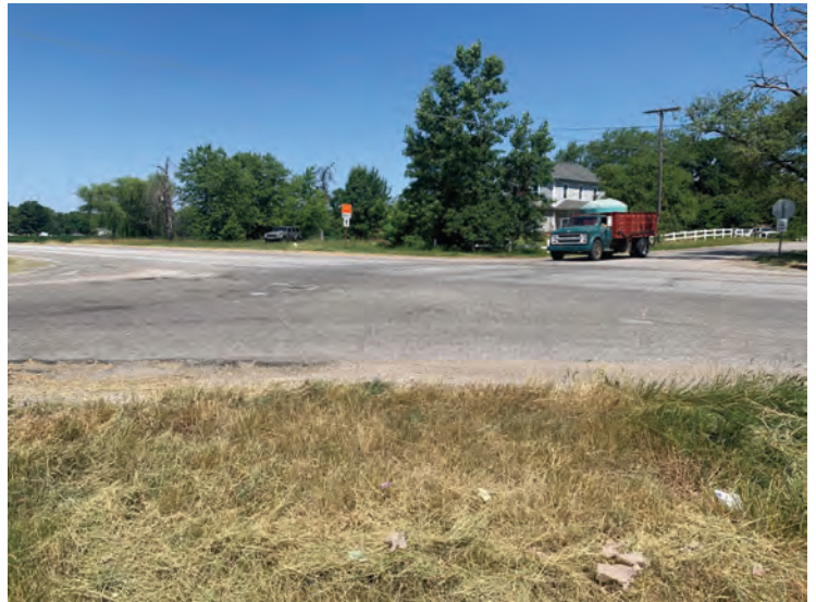
10. Looking northwest at intersection of US 6 and Dogwood RD
