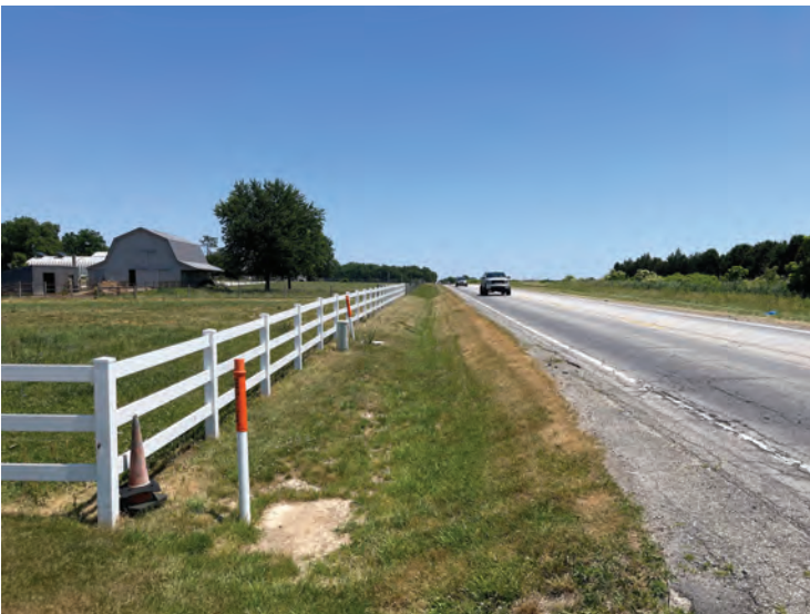
29. Looking east along north side US 6
