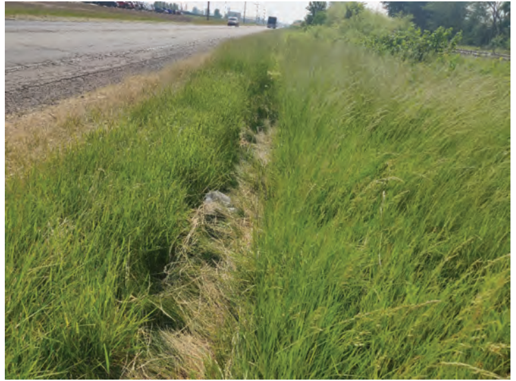
38. Looking east along south side of US 6
