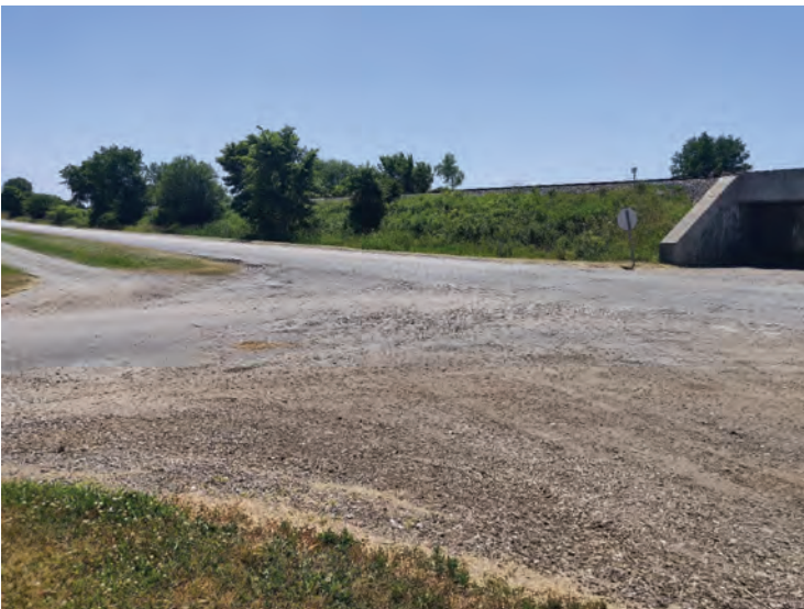
35. Looking southeast at intersection of US 6 and CR 100
