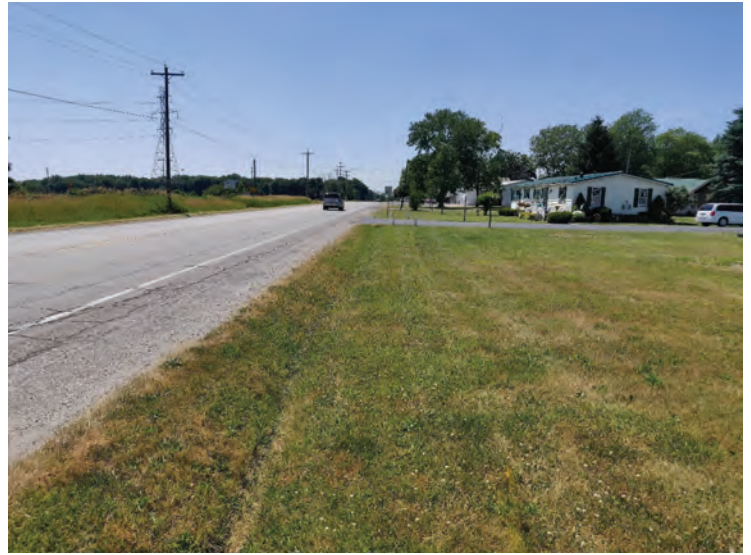
26. Looking west along north side of US 6
