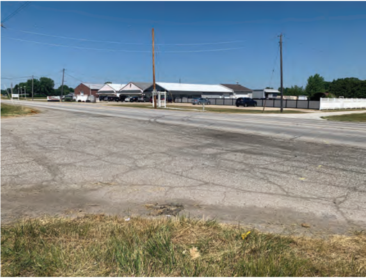
7. Looking northwest at intersection of US 6 and US 6 Access Road
