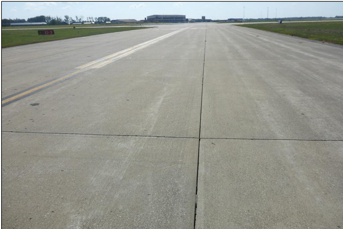
Figure 2-3. Typical PCC Pavement in Good Condition (Feature 106)
