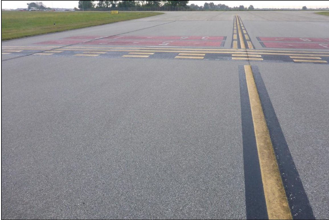
Figure 2-6. Typical AC Pavement in Good Condition (Feature 130)
