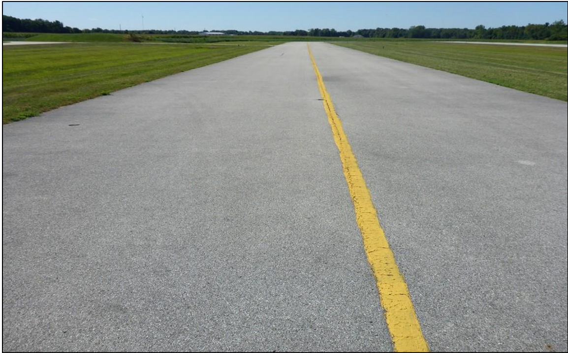
Figure 2-4. Typical AC Pavement in Good Condition (Feature 110)
