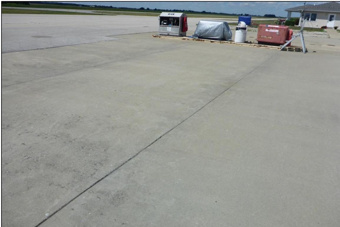
Figure 2-3. Typical PCC Pavement in Good Condition (Feature 3050)
