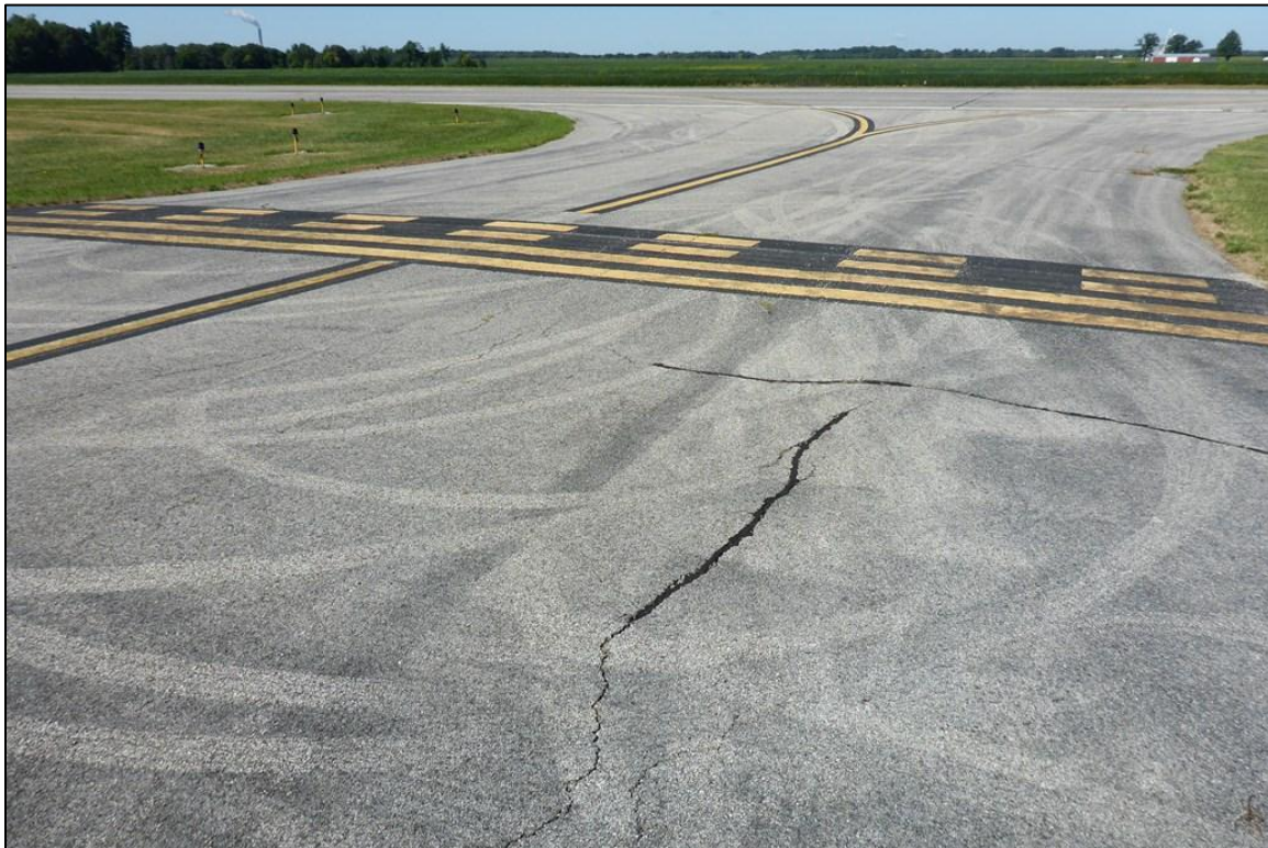
Figure 2-5. Typical AC Pavement in Fair Condition (Feature 405)
