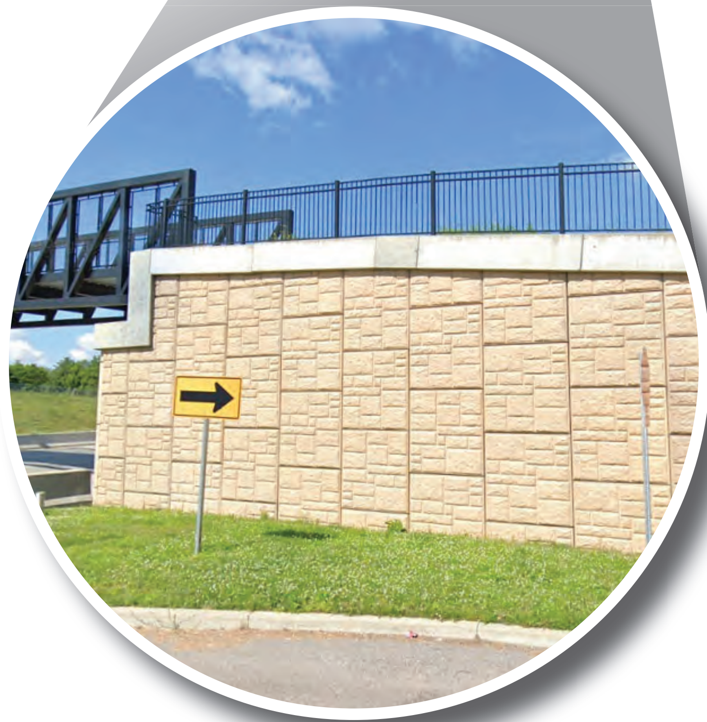
Example of Standard Railing at Llyod Expressway
