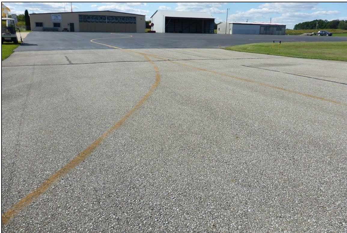
Figure 2-5. Typical AC Pavement in Fair Condition (Feature 115)
