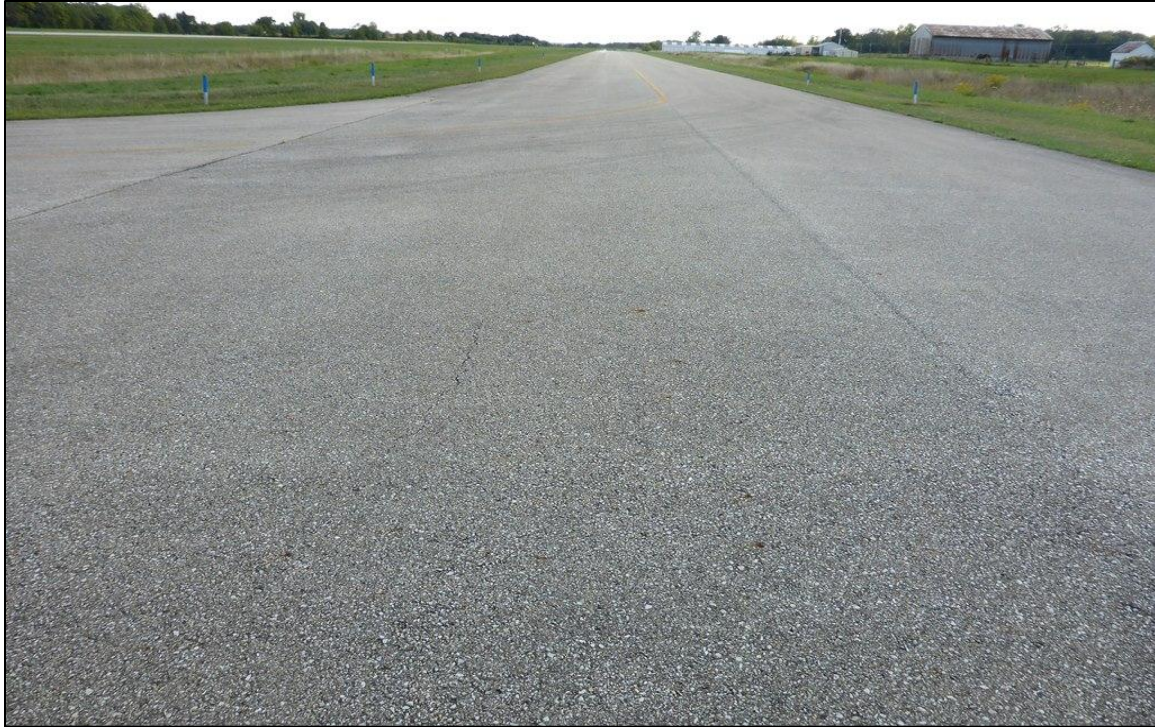
Figure 2-4. Typical AC Pavement in Good Condition (Feature 105)
