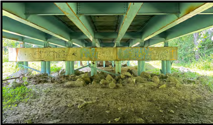
Photo 51: Looking northwest from under the south side of the bridge.
