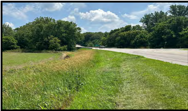
Photo 3: Looking southeast along RSD1, within the northeast quadrant of the investigated area.
