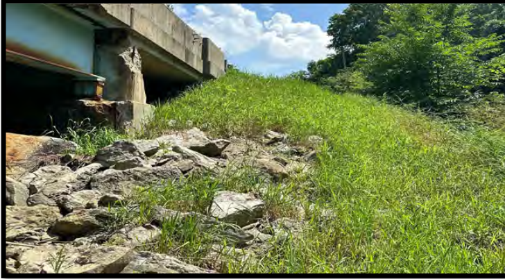
Photo 49: Looking southeast along the southwest side of the bridge.
