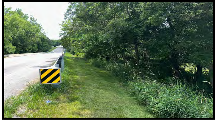
Photo 62: Looking southeast along RSD4 from the northwest approach.
