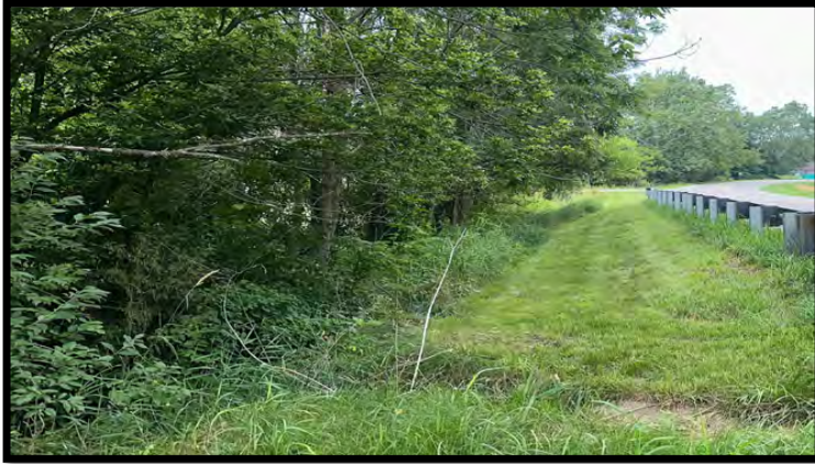
Photo 61: Looking northwest along RSD4 from the northwest corner of the bridge.
