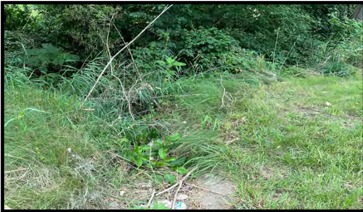
Photo 11: Looking northeast along a short drainage from the northeast corner of the bridge.
