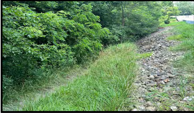
Photo 41: Looking northwest toward the end of the concrete section of RSD3.
