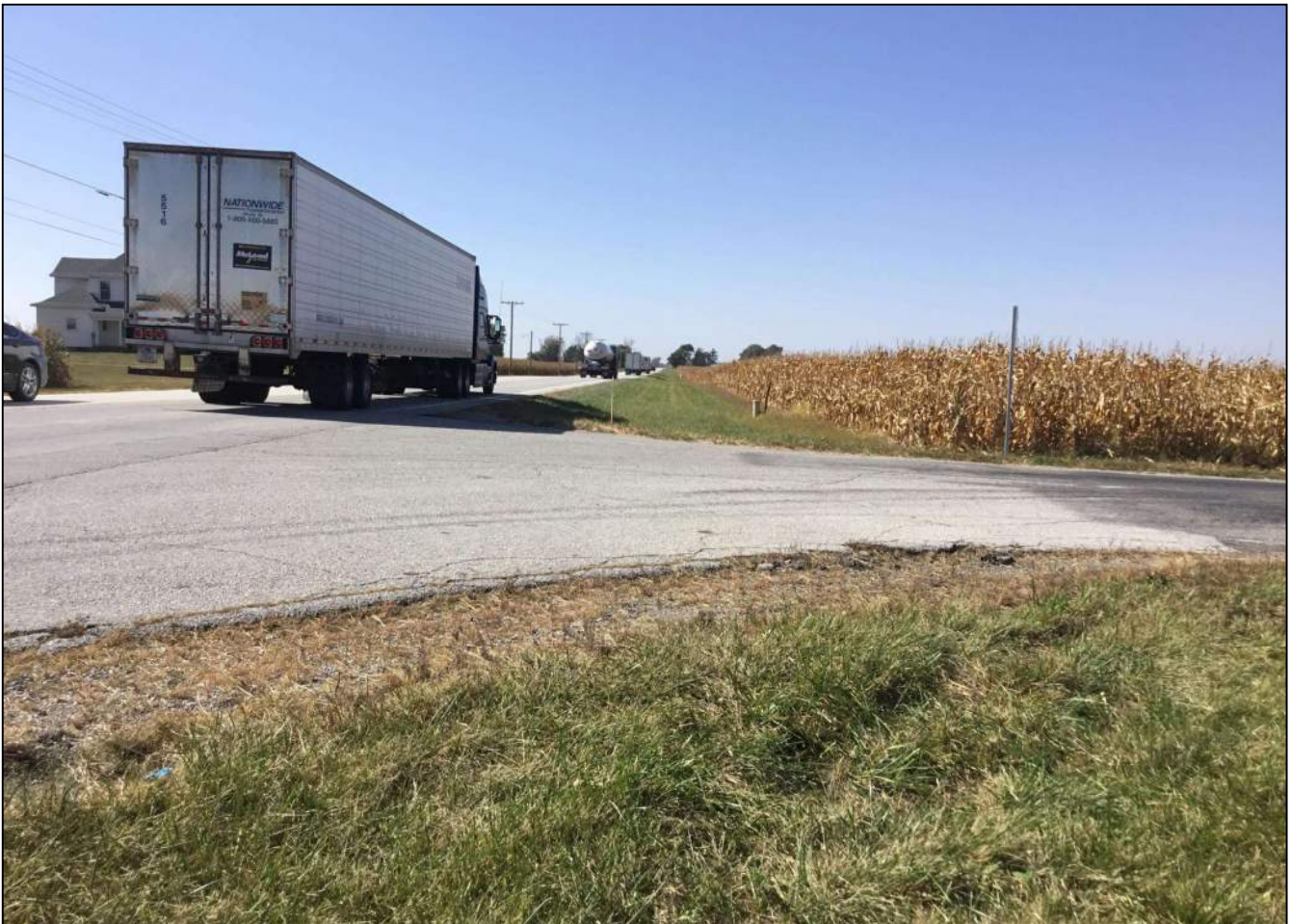
175. Looking west along the north side of SR 32 at the CR 900 W. intersection. Photo taken October 7, 2020.
