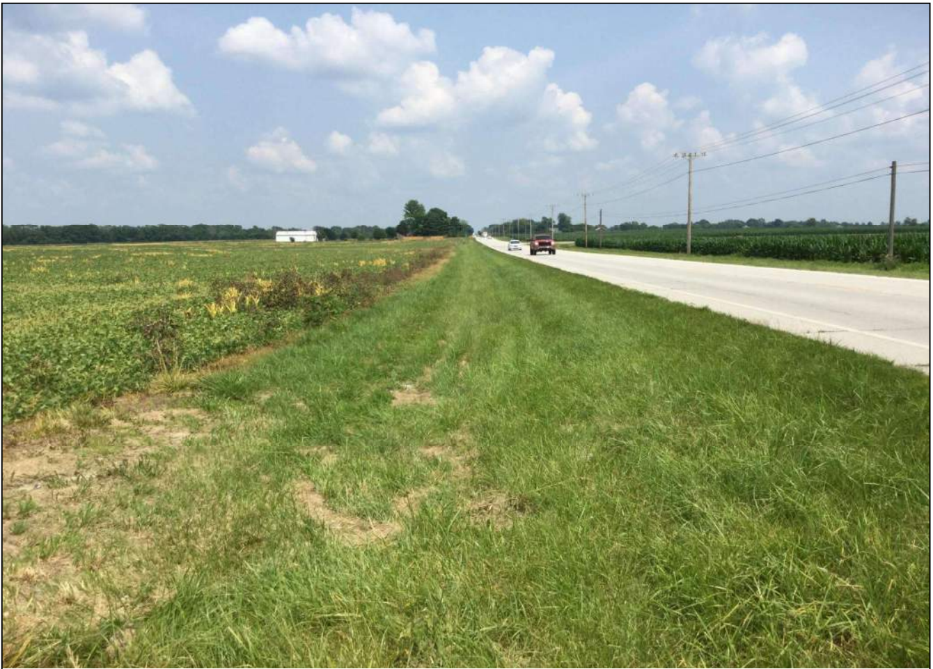
173. Looking east along the north side (WB lane) of SR 32 at the surrounding landscape. Photo taken July 6, 2021.
