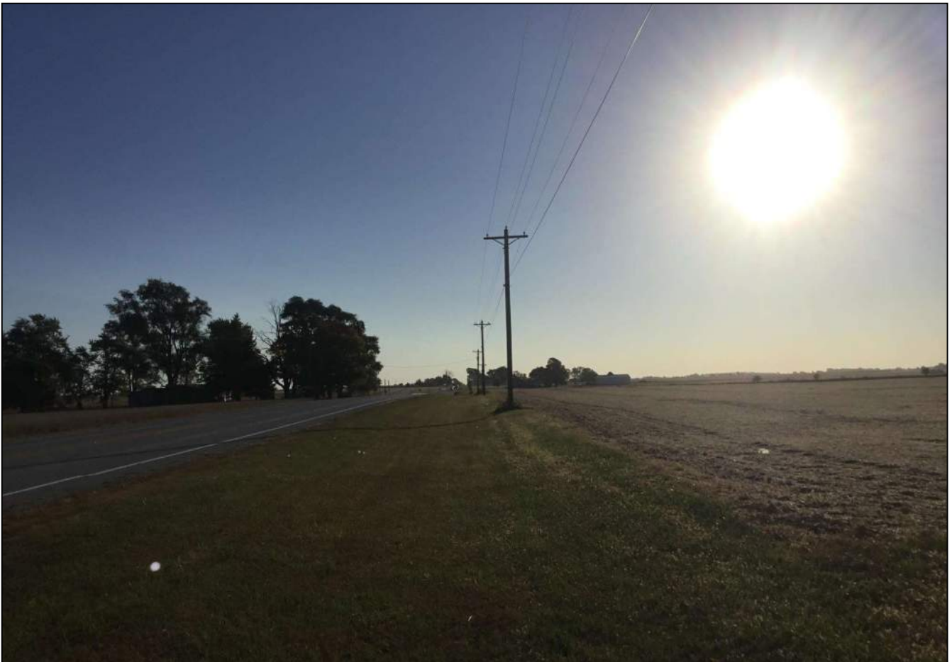
187. Looking east along the south side (EB lane) of SR 32 just east of the CR 1075 W. intersection and Structure No. 104. Photo taken October 8, 2020.
