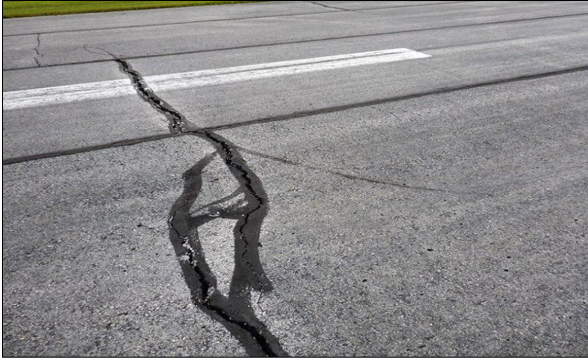
Figure 2-4. Typical AC Pavement in Fair Condition (Feature 6105)
