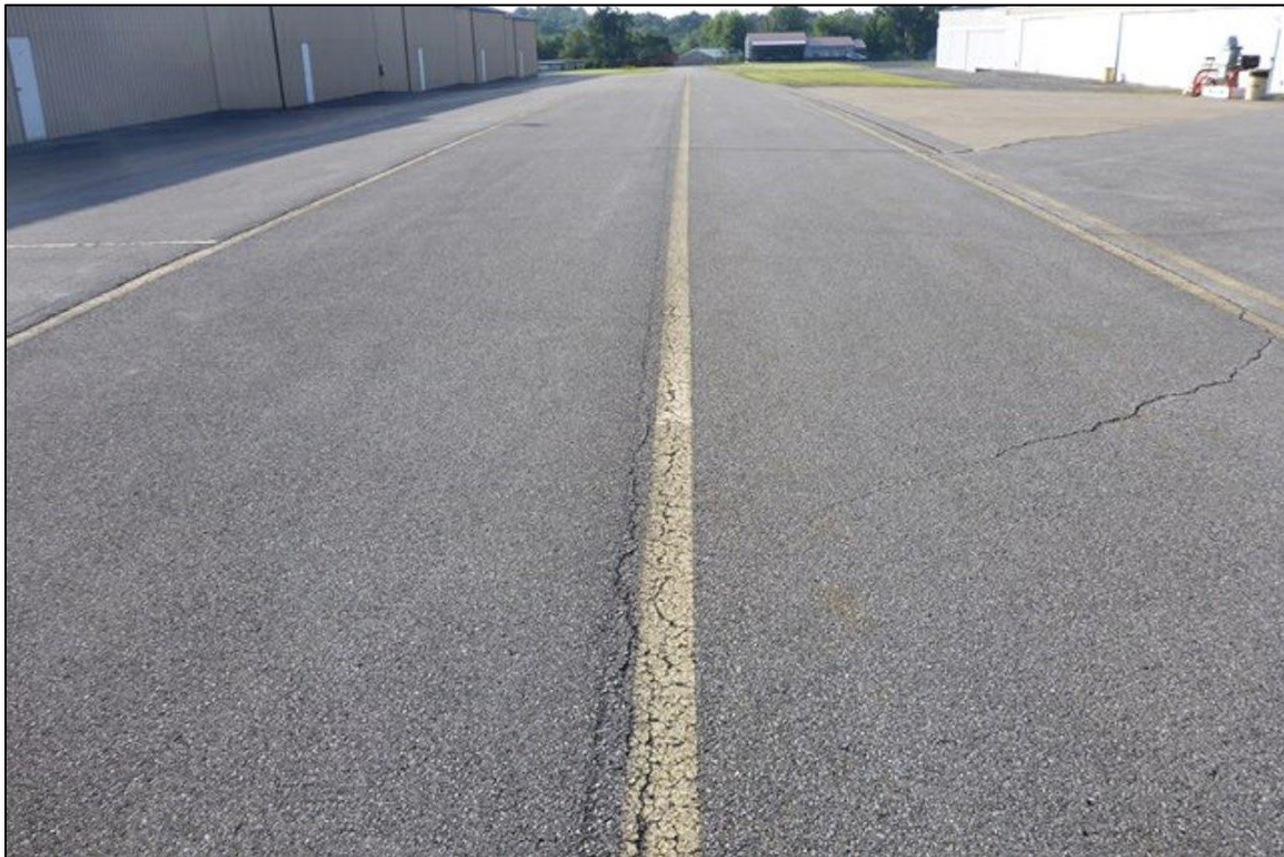
Figure 2-3. Typical AC Pavement in Good Condition (Feature 105)
