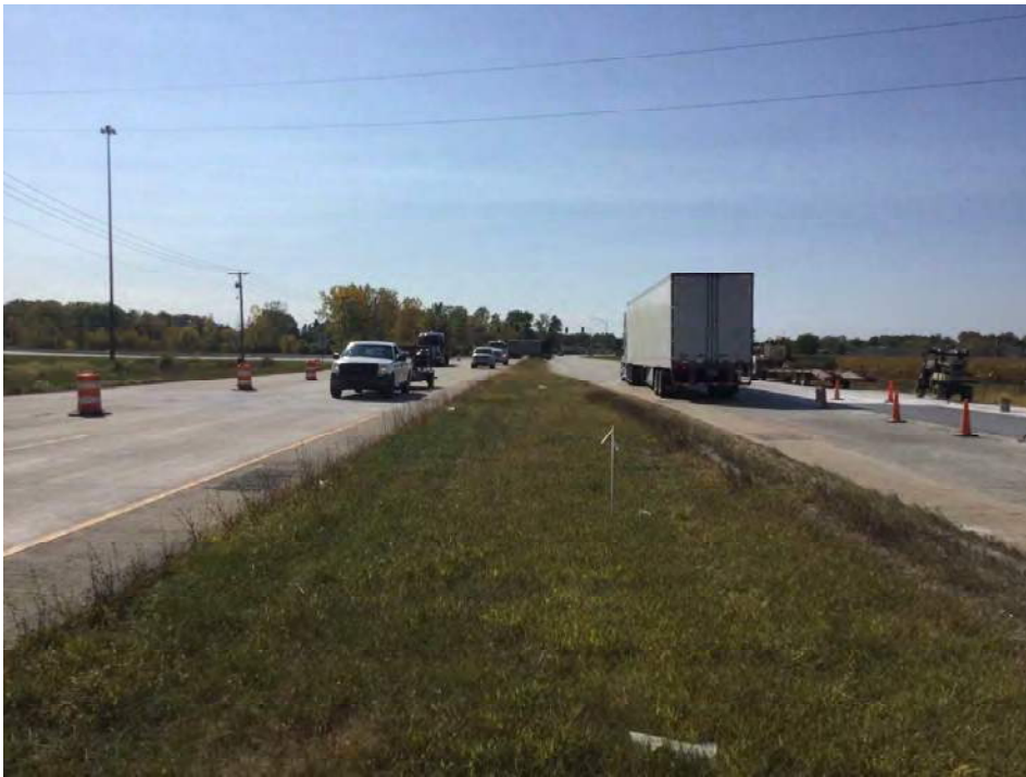
33. Looking southwest along US 24 median
