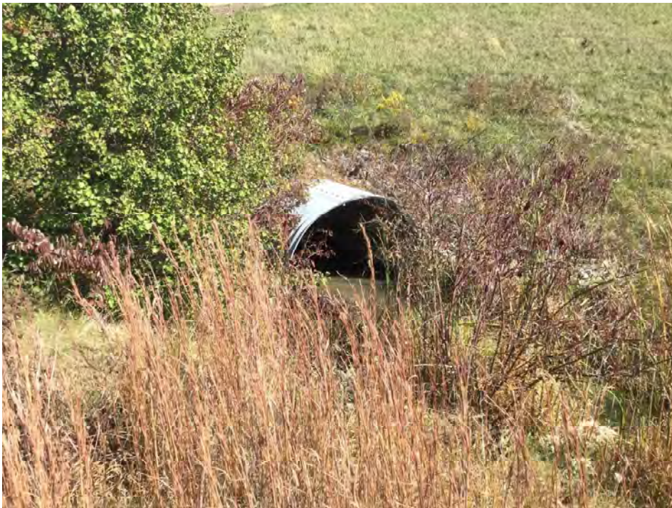
35. Looking east towards Wetland-F culvert Des No 1800092
