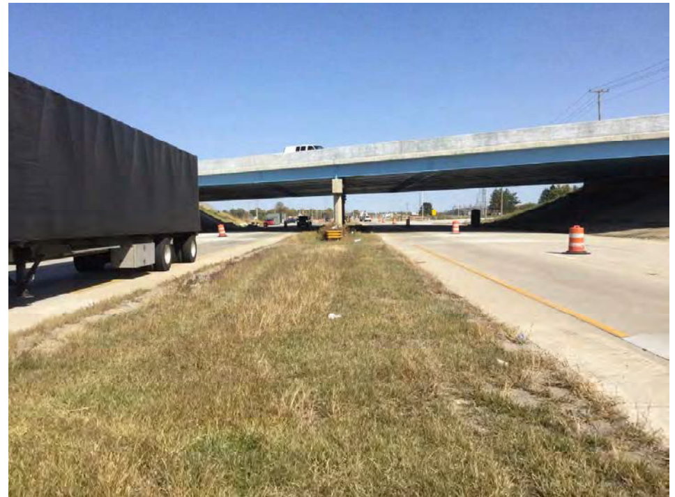
32. Looking northeast in US 24 median
