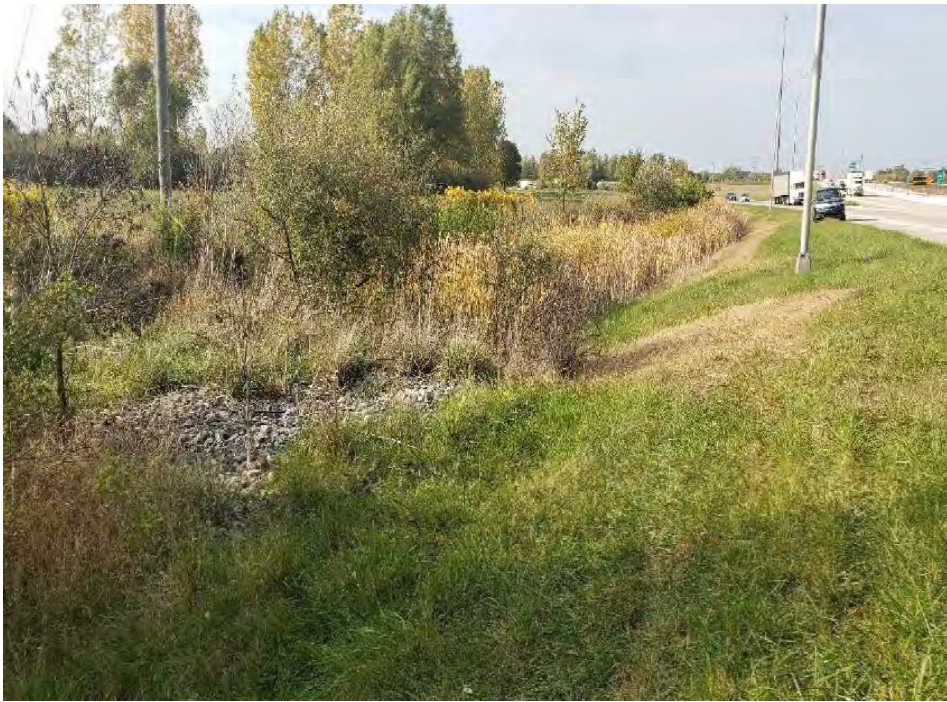
65. Looking northwest at southern end of RSD 3
