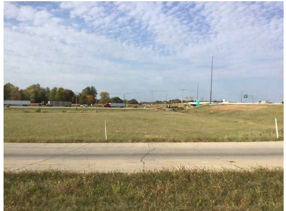
60. Looking north at I-469 interchange median Appendix B, Page 25 of 38
