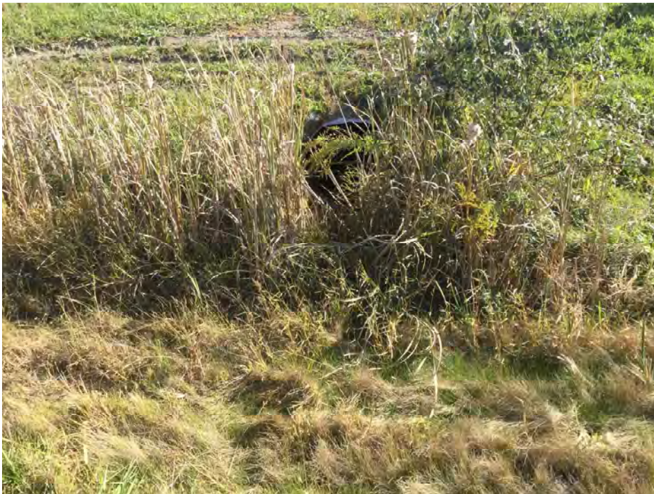
47. Looking south west at culvert
