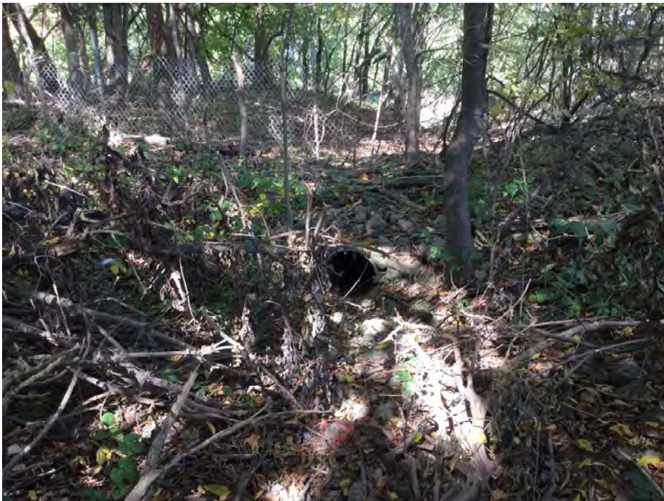
27. Looking north towards culvert note RSD 1 Des No 1800092
