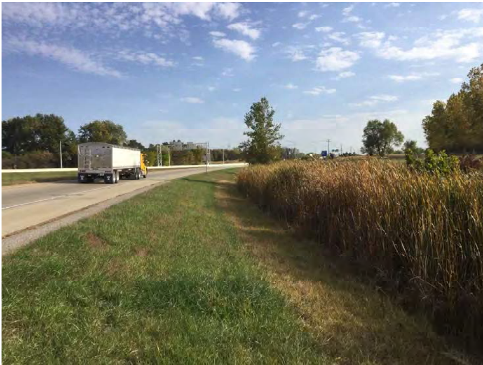
63. Looking south along I-469 on ramp and RSD 3 Des No 1800092
