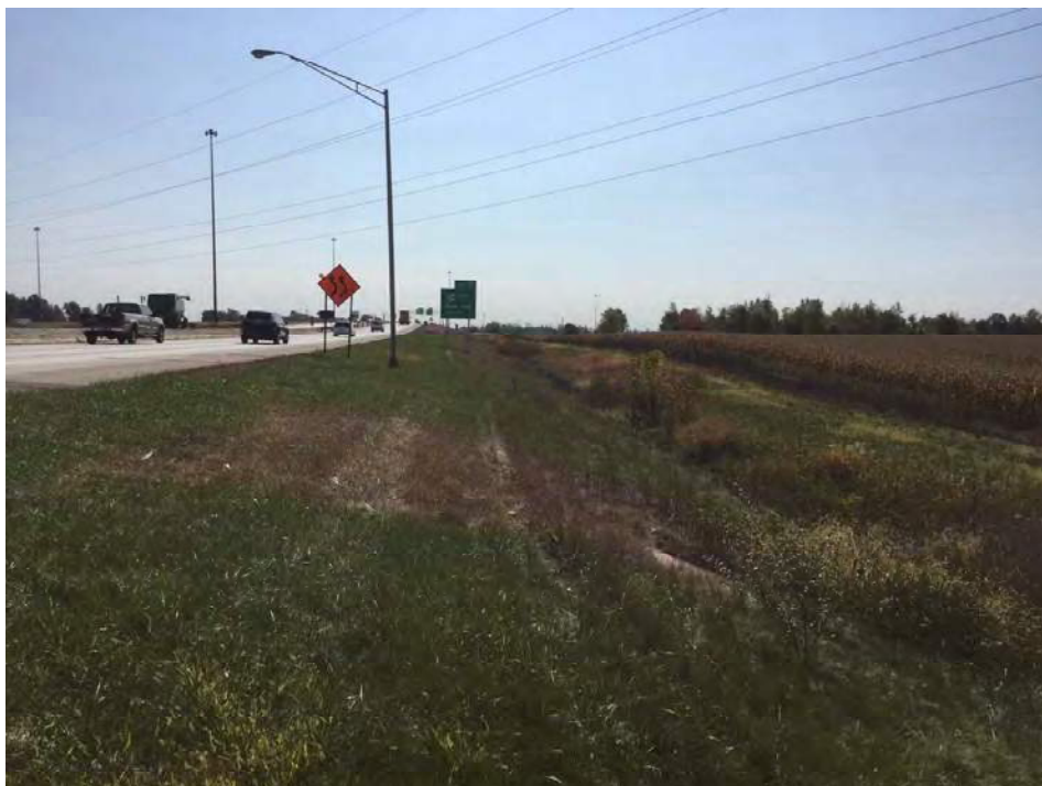
23. Looking south along I-469
