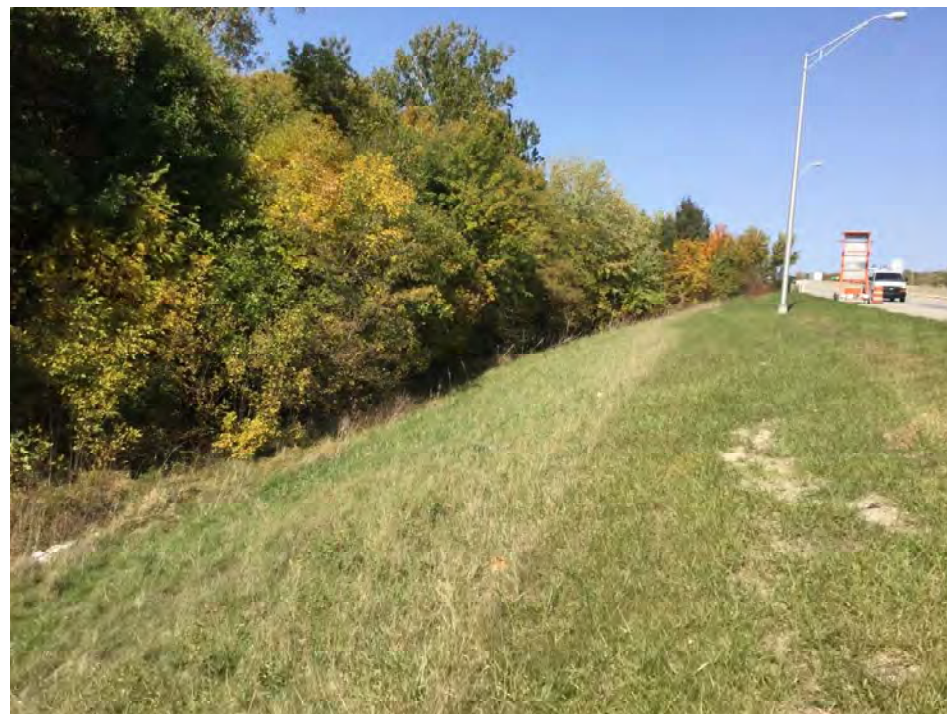
24. Looking north west along I-469
