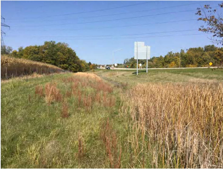
29. Looking north along right of way note RSD 1
