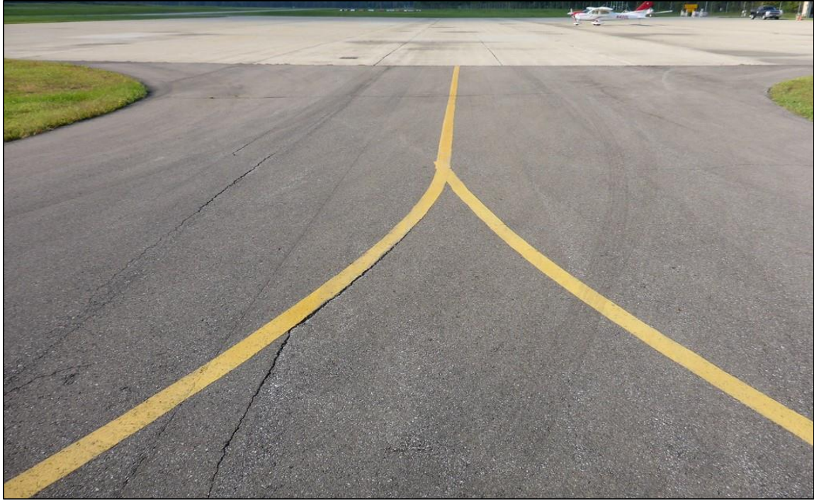
Figure 2-4. Typical AC Pavement in Good Condition (Feature 315)
