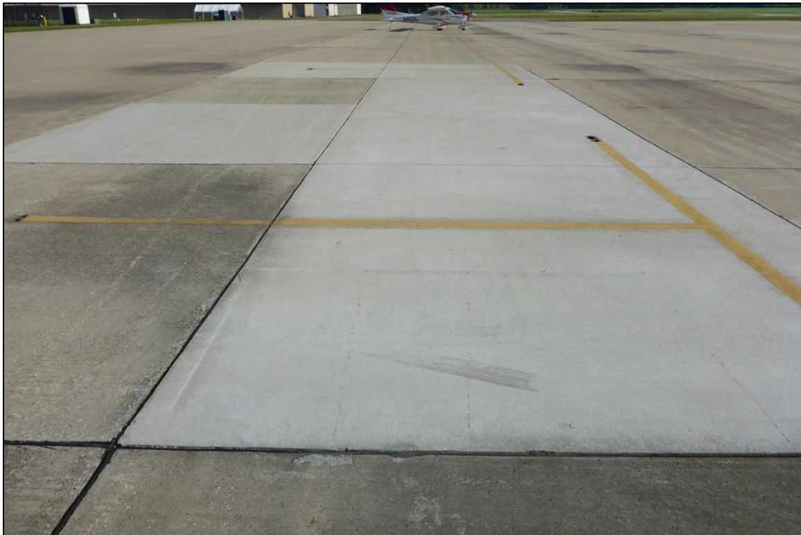
Figure 2-3. Typical PCC Pavement in Good Condition (Feature 3005)
