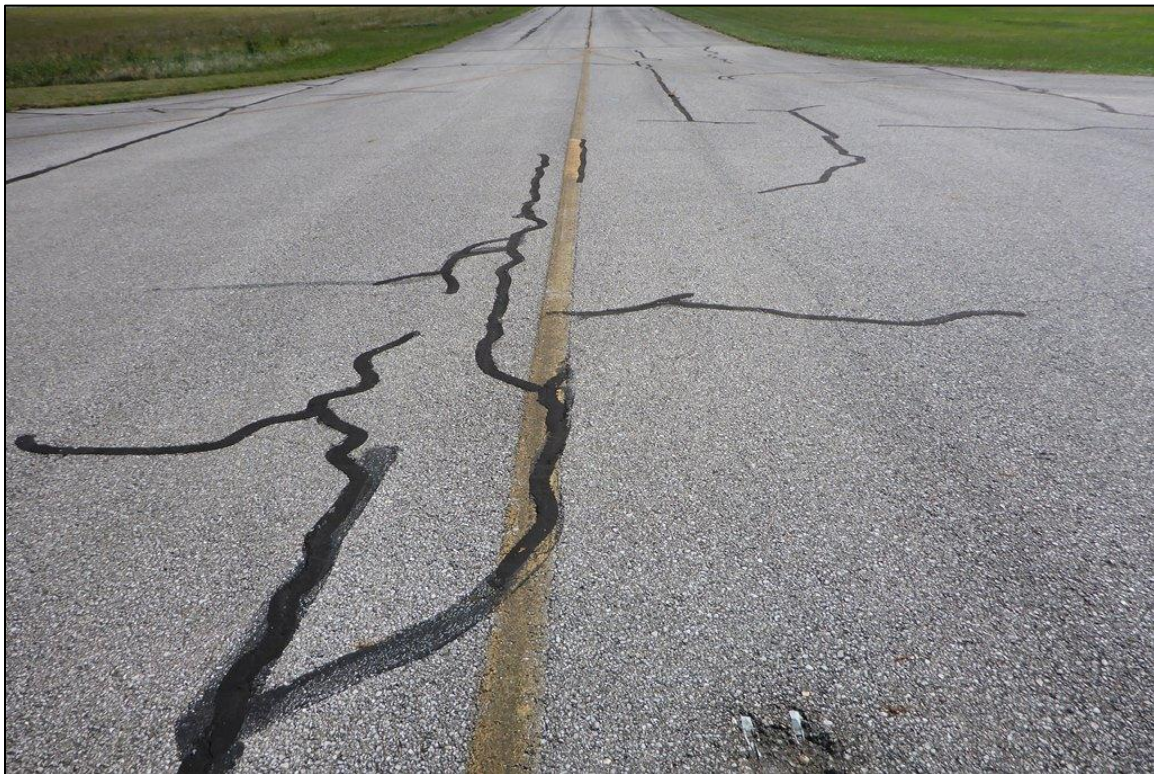
Figure 2-5. Typical AC Pavement in Fair Condition (Feature 120)
