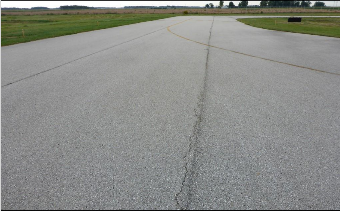
Figure 2-4. Typical AC Pavement in Good Condition (Feature 170)
