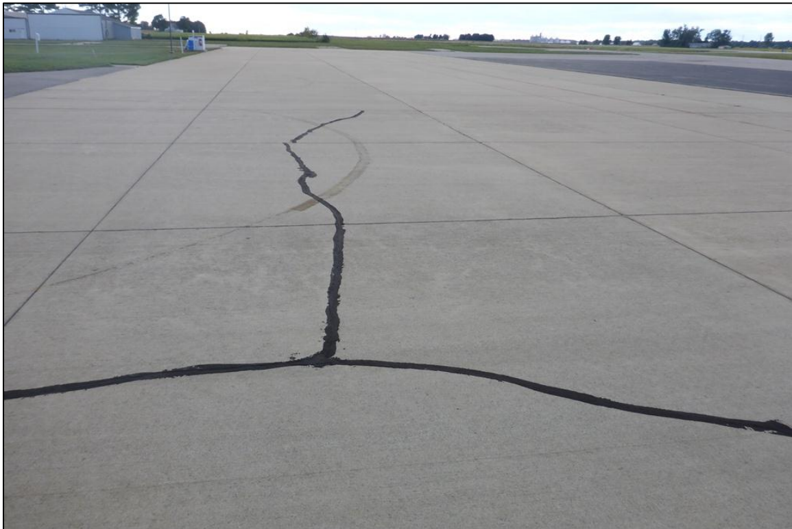
Figure 2-3. Typical PCC Pavement in Good Condition (Feature 3015)
