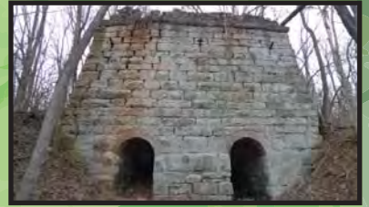
Local example of a continuous-burning vertical shaft type kiln.
