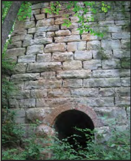
Chamber opening and limestone wall of a continuous-burning vertical kiln.
