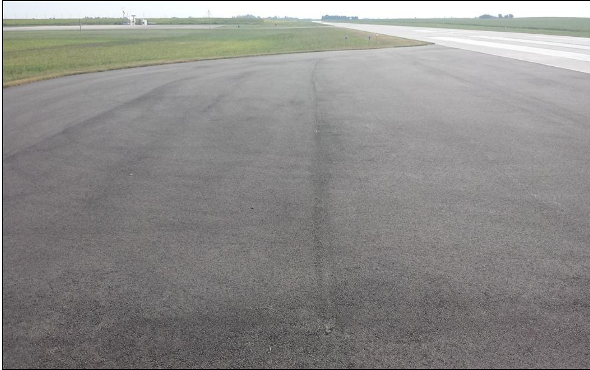
Figure 2-4. Typical AC Pavement in Good Condition (Feature 4105)
