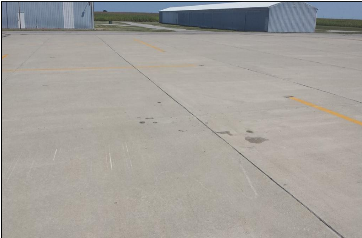
Figure 2-3. Typical PCC Pavement in Good Condition (Feature 3015)
