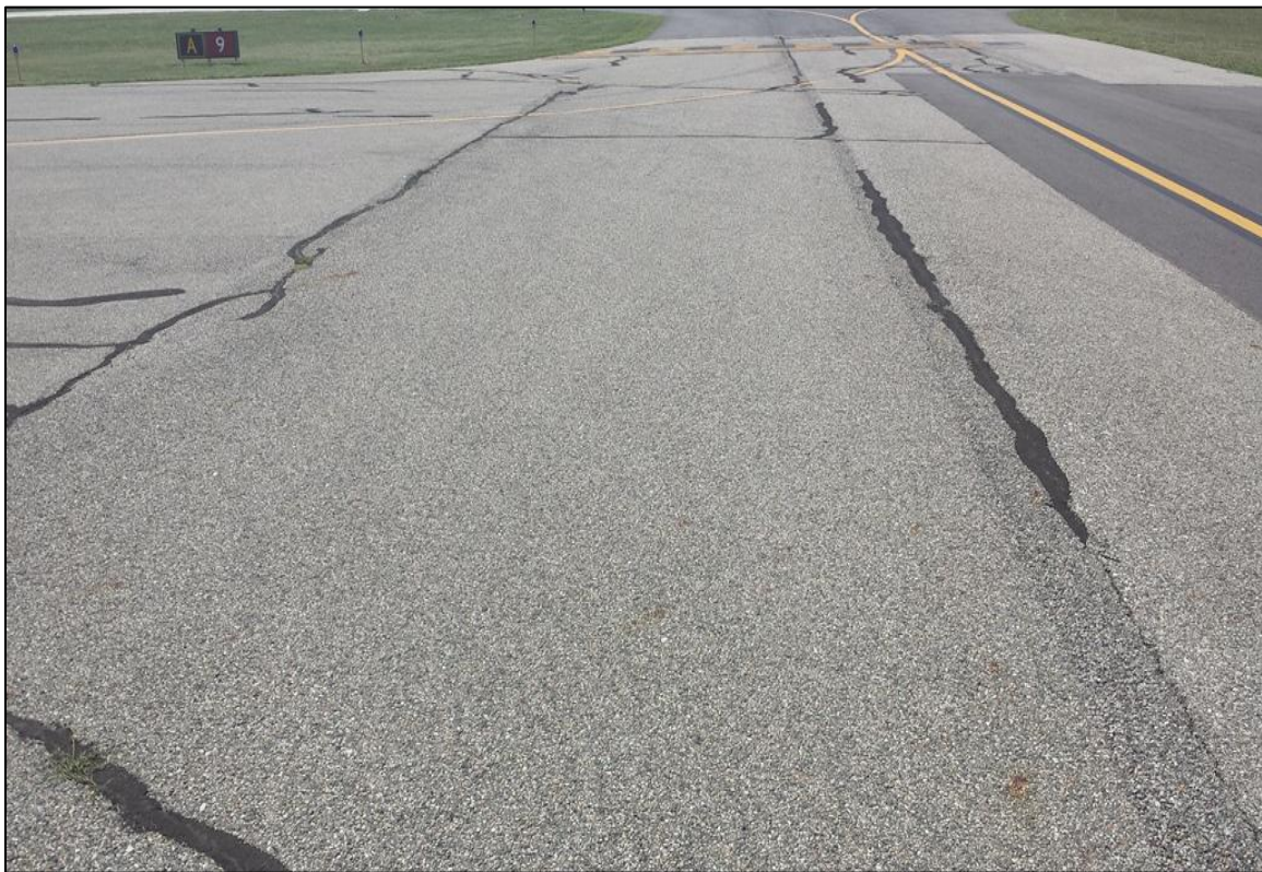
Figure 2-5. Typical AC Pavement in Fair Condition (Feature 105)
