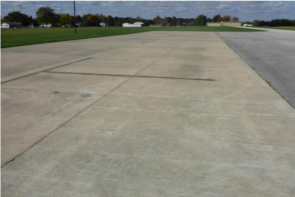
Figure 2-3. Typical PCC Pavement in Good Condition (Feature 3010)
