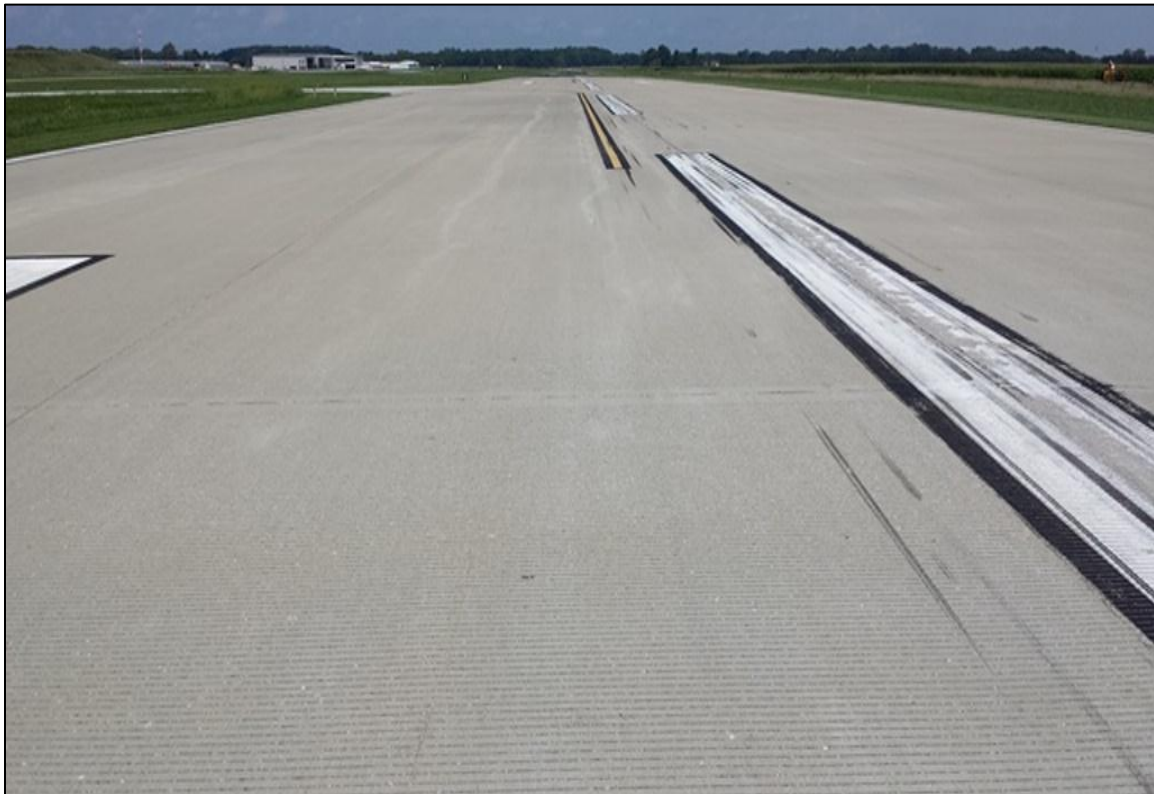
Figure 2-3. Typical PCC Pavement in Good Condition (Feature 6105)
