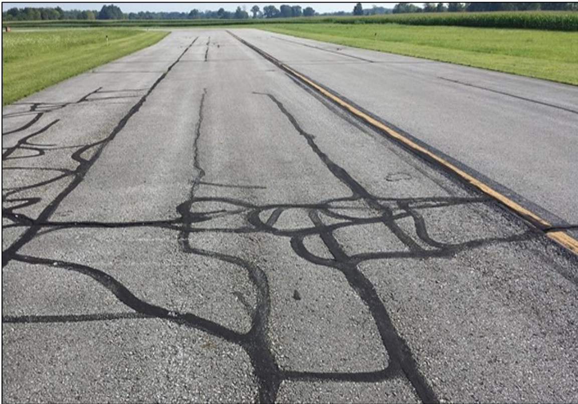
Figure 2-5. Typical AC Pavement in Fair Condition (Feature 115)
