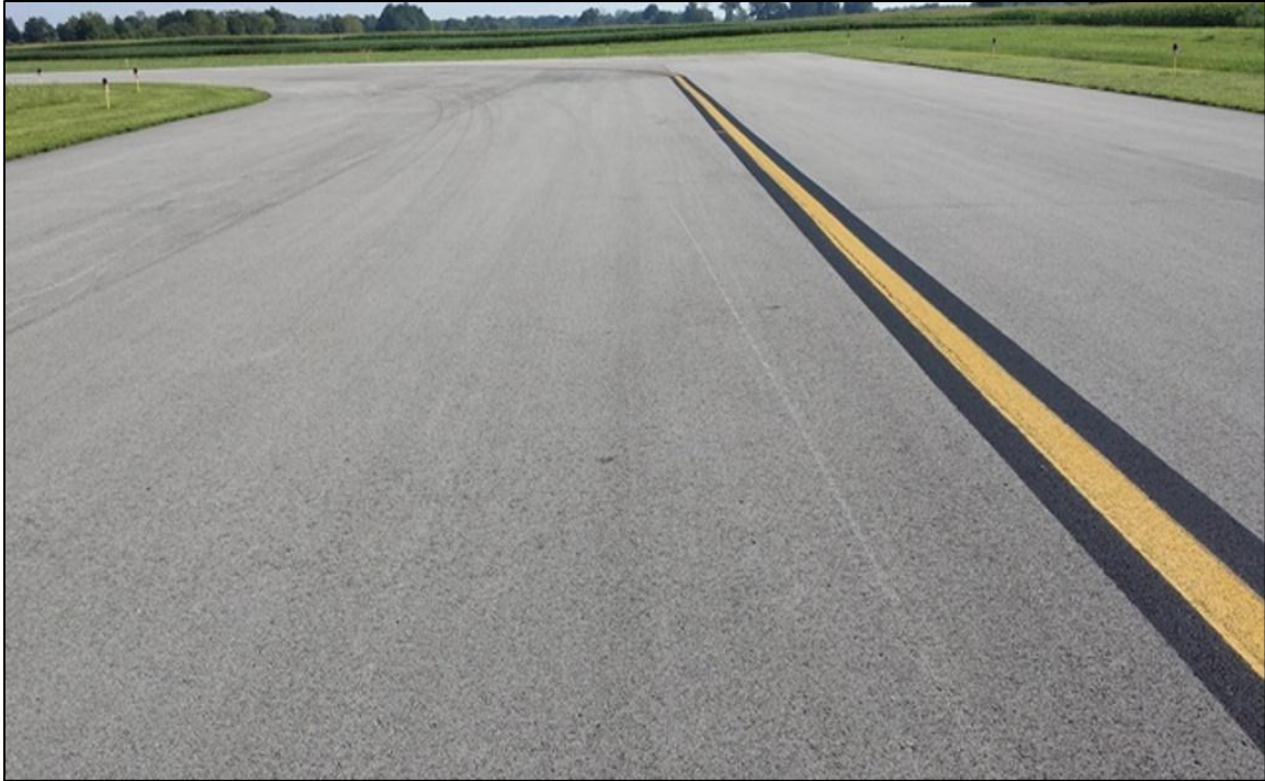
Figure 2-4. Typical AC Pavement in Good Condition (Feature 117)
