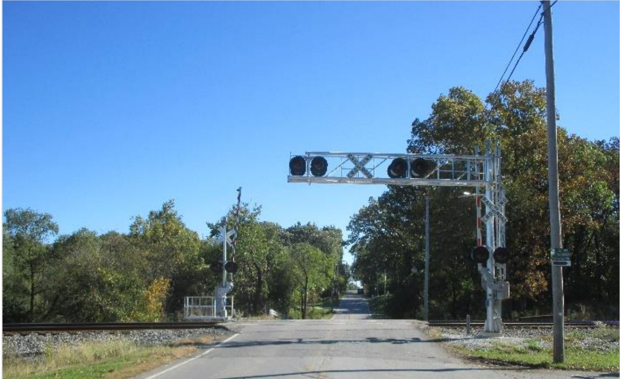
Photo 7: Typical Section 130 Project
