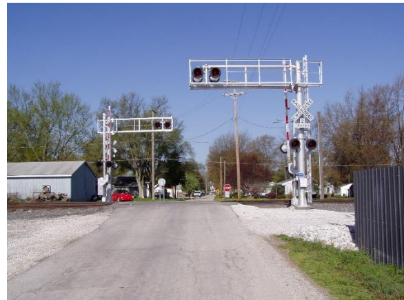
Photo 6: Typical Section 130 Project
