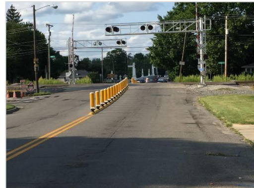
Photo 6: Median Barrier, South Bend
