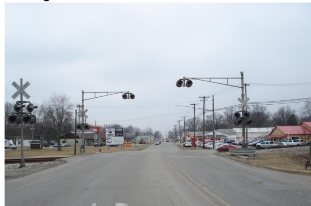
Photo 3: Typical Flashing Lights Only Installation in Need of Upgrade
