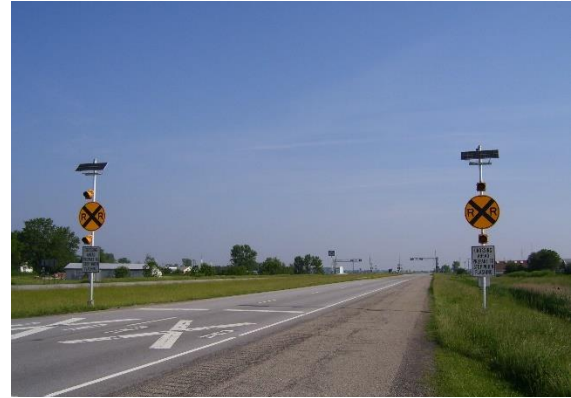
Photo 8: Advance Warning Signs
