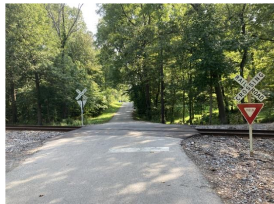
Photo 4: Typical Rural Railroad Crossing
