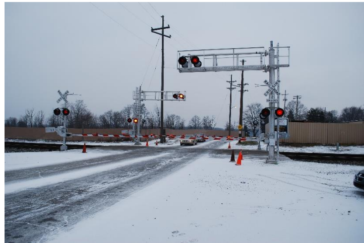
Photo 7: Four-Quadrant Gate, Tipton
