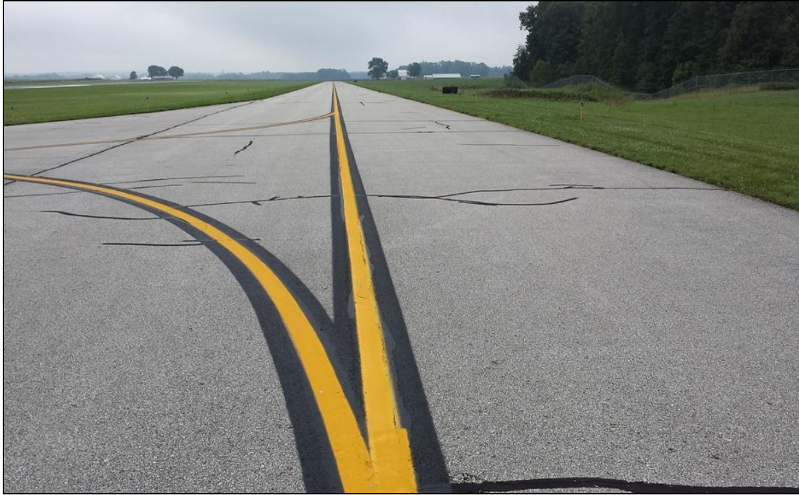
Figure 2-4. Typical AC Pavement in Good Condition (Feature 115)
