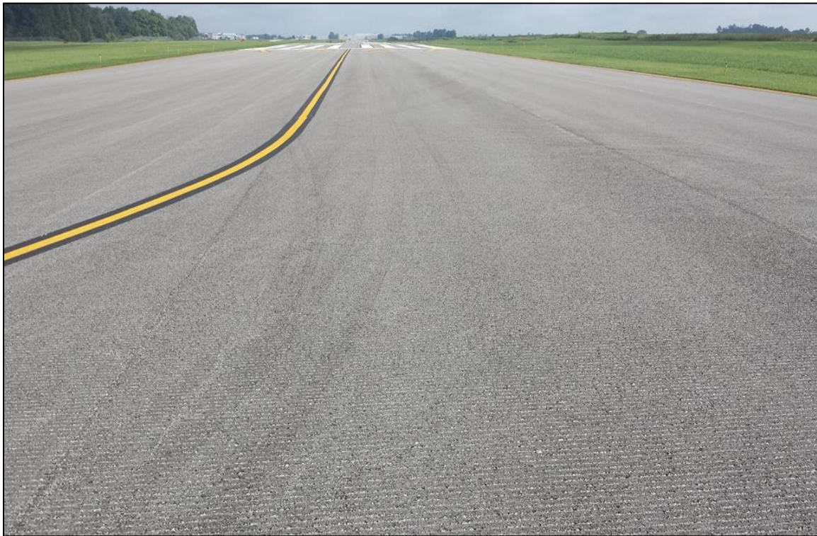
Figure 2-3. Typical AC Pavement in Good Condition (Feature 6105)
