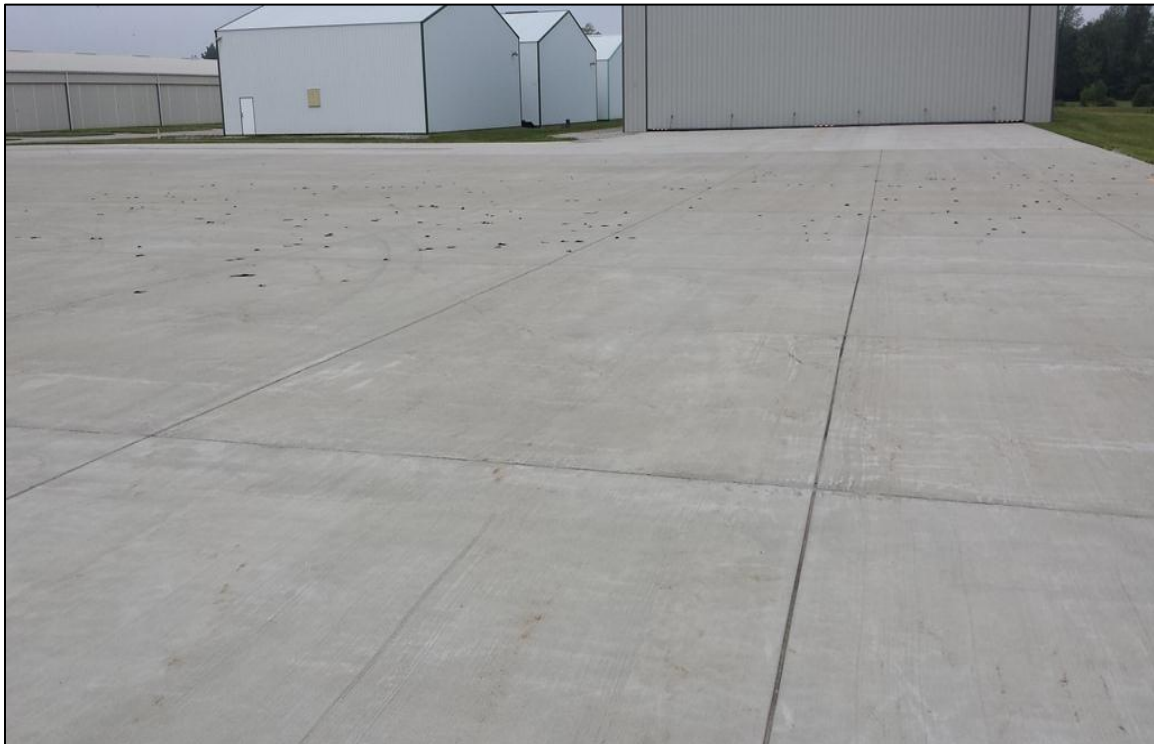
Figure 2-5. Typical PCC Pavement in Good Condition (Feature 3120)
