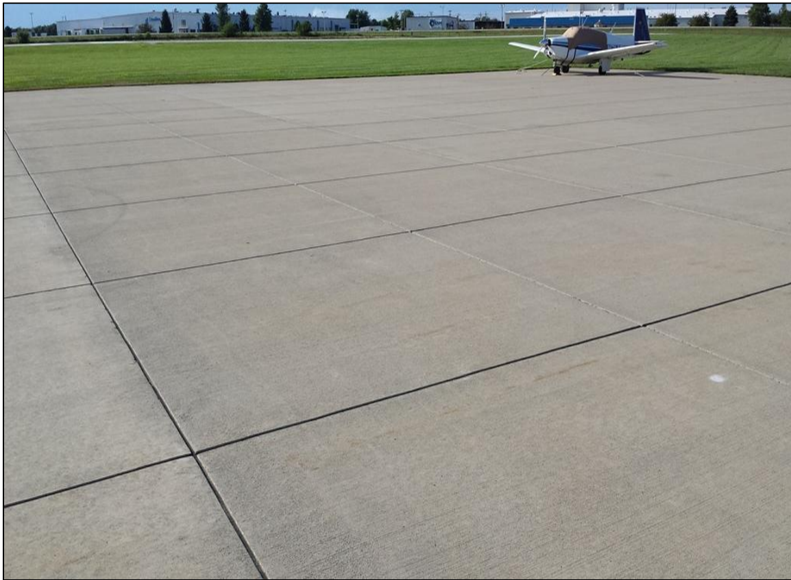
Figure 2-3. Typical PCC Pavement in Good Condition (Feature 3015)
