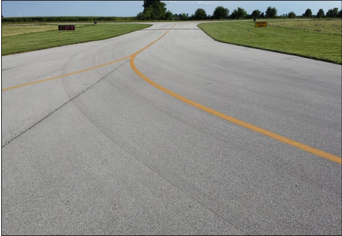
Figure 2-4. Typical AC Pavement in Good Condition (Feature 130)
