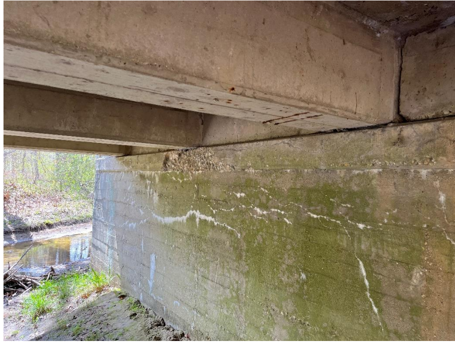
Photo: 13 Vantage Point: Under Span A Direction: Looking southwest Description: Abutment 1
