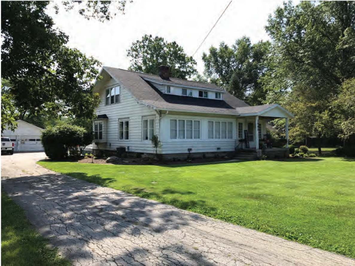
17. Looking SE at Lochmueller #9, Contributing, 1331 S. Meridian Street
