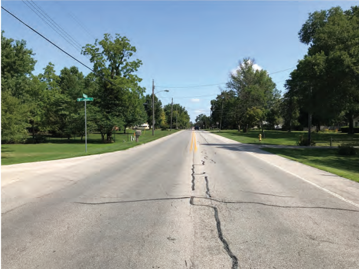
5. Looking N at the S end of the project limits on US 27 (Meridian Street)
