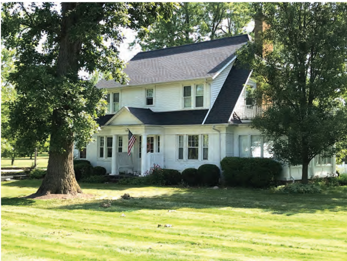
24. Looking NE at Lochmueller #12, Contributing, 1303 S. Meridian Street
