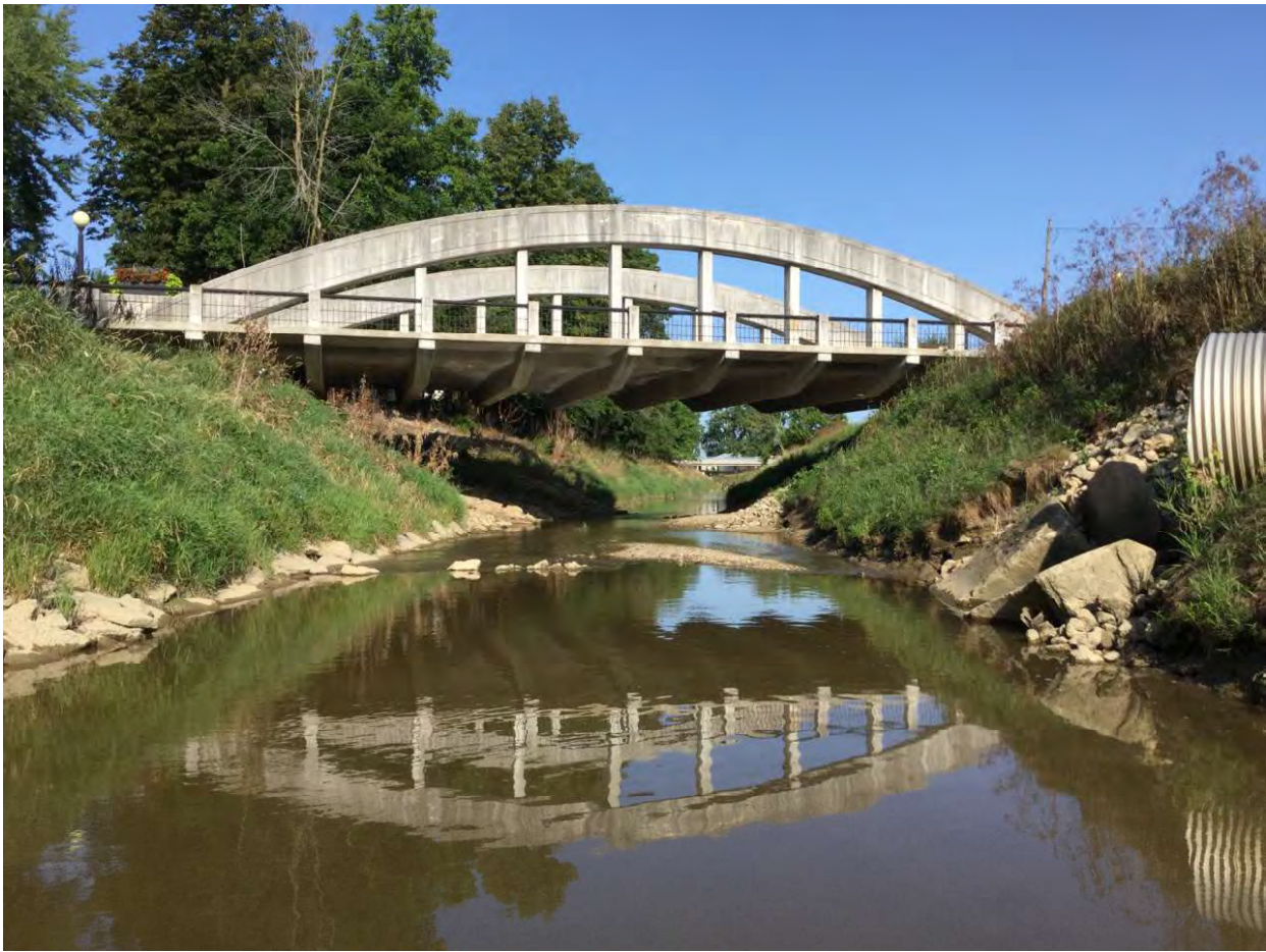
3. Looking west (downstream) towards bridge over the Salamonie River.
