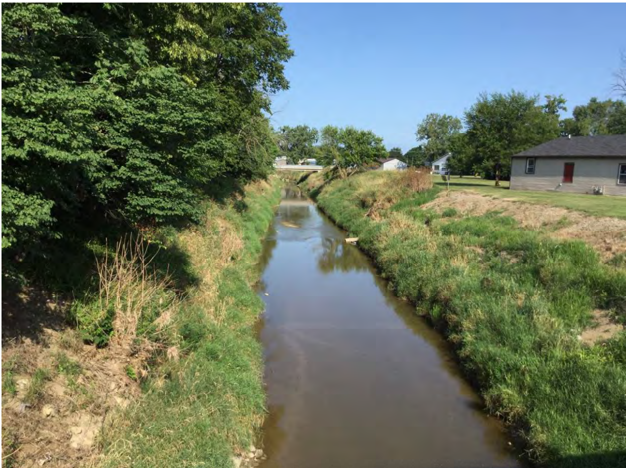
8. Looking west (downstream) from the bridge along the Salamonie River.
