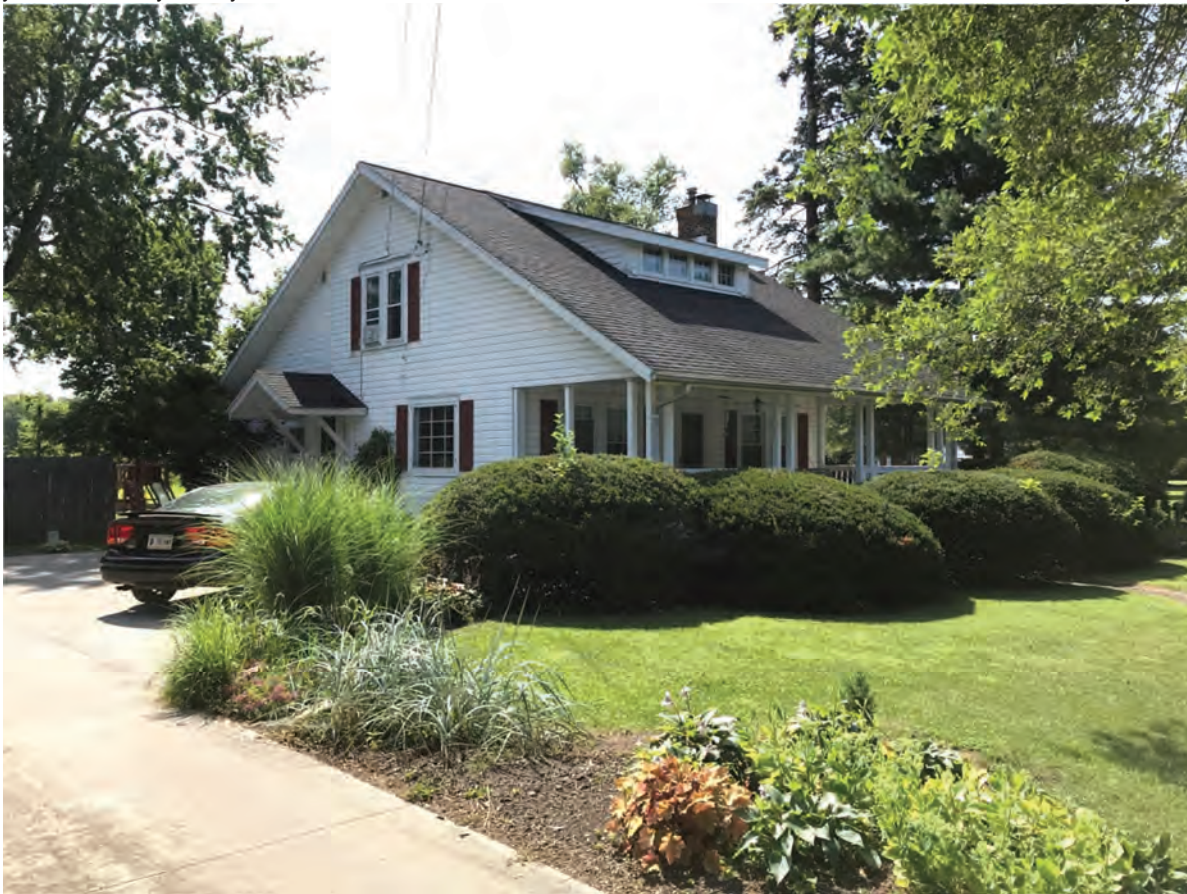
11. Looking SE at IHSSI #075-521-33099, Contributing, 1345 S. Meridian Street
