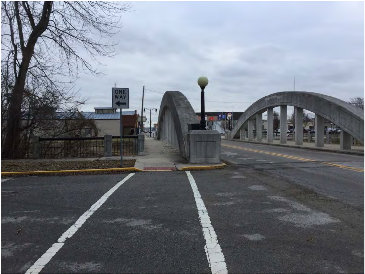
9. Looking north toward bridge over Salamonie River
