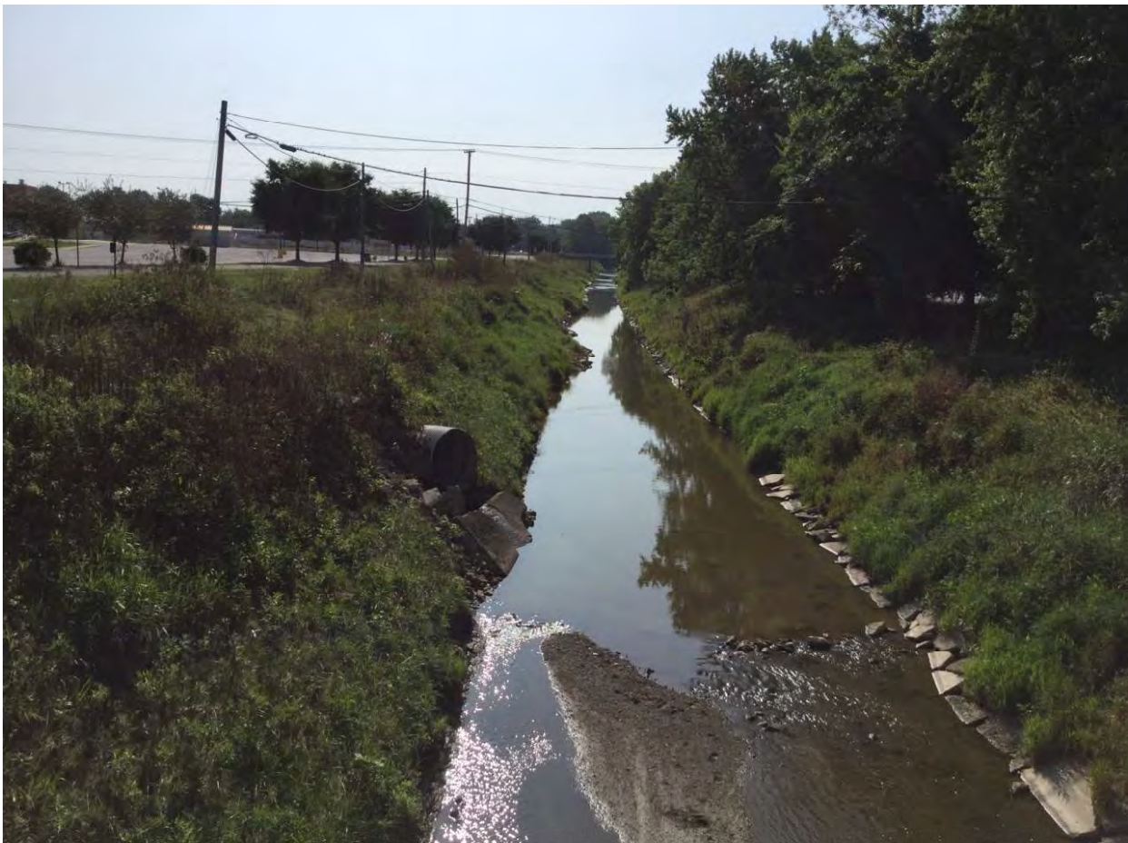
6. Looking east (upstream) from the bridge along the Salamonie River.
