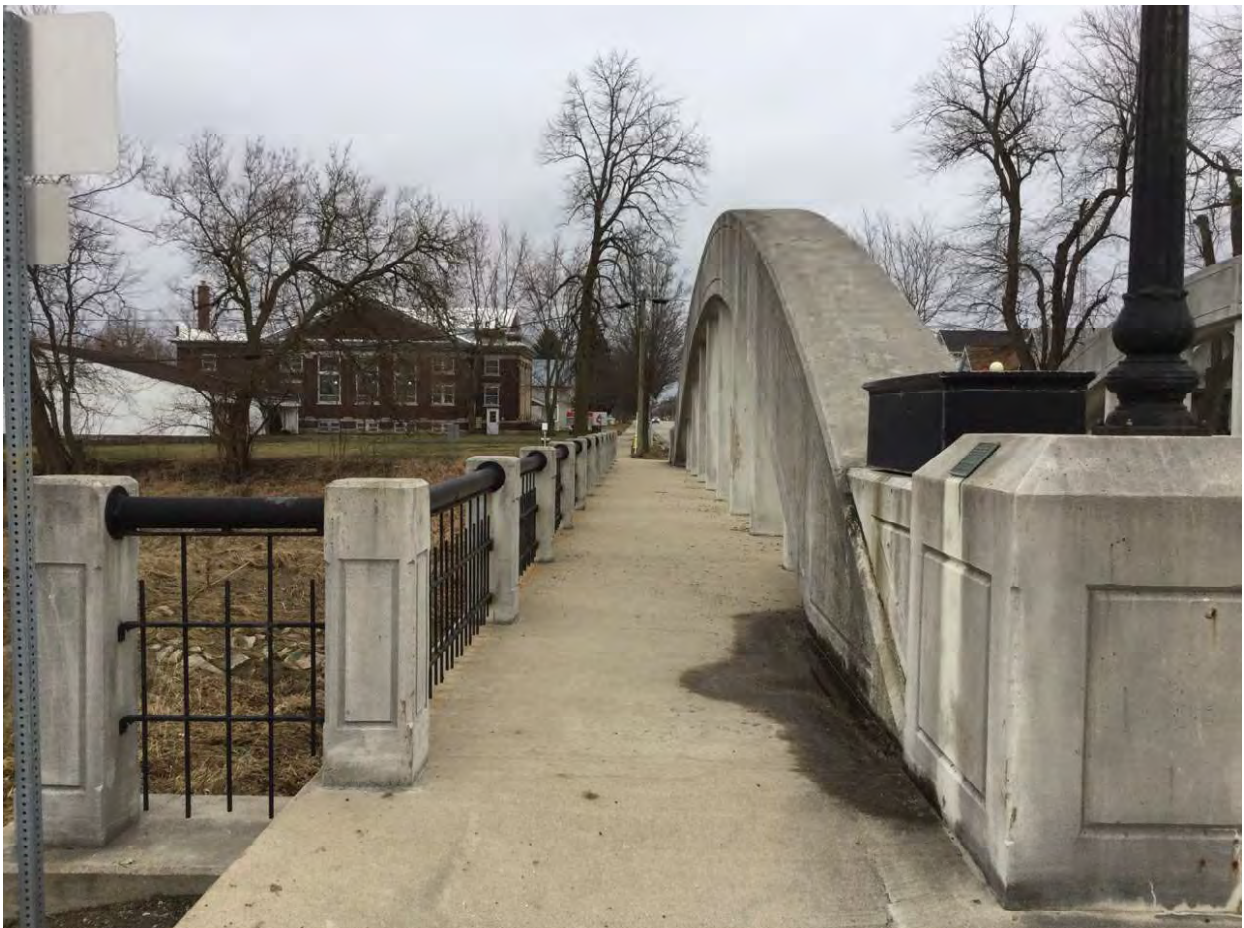
10. Looking south along east side of bridge structure
