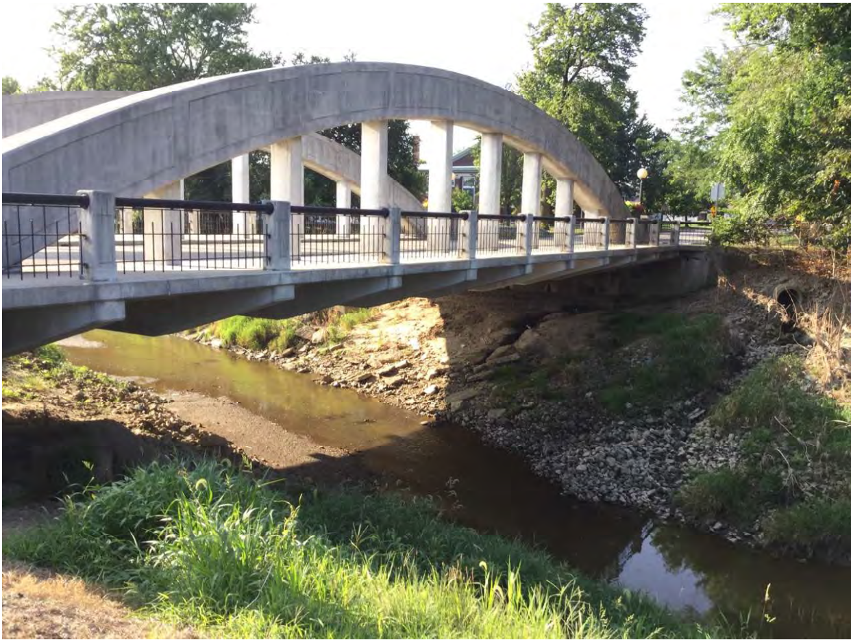
1. Looking southeast towards bridge over the Salamonie River.
