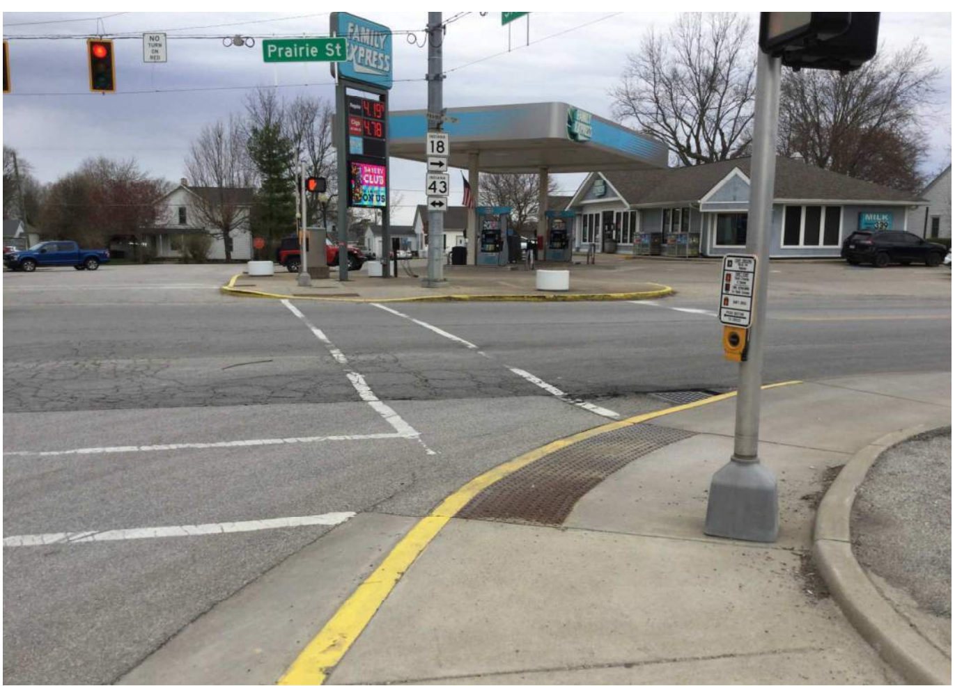
19. Looking west / northwest from the SR 18 South Junction / SR 43 Intersection at existing pedestrian facilities. Note: SR 18 is known locally as West 3 rd Street.
