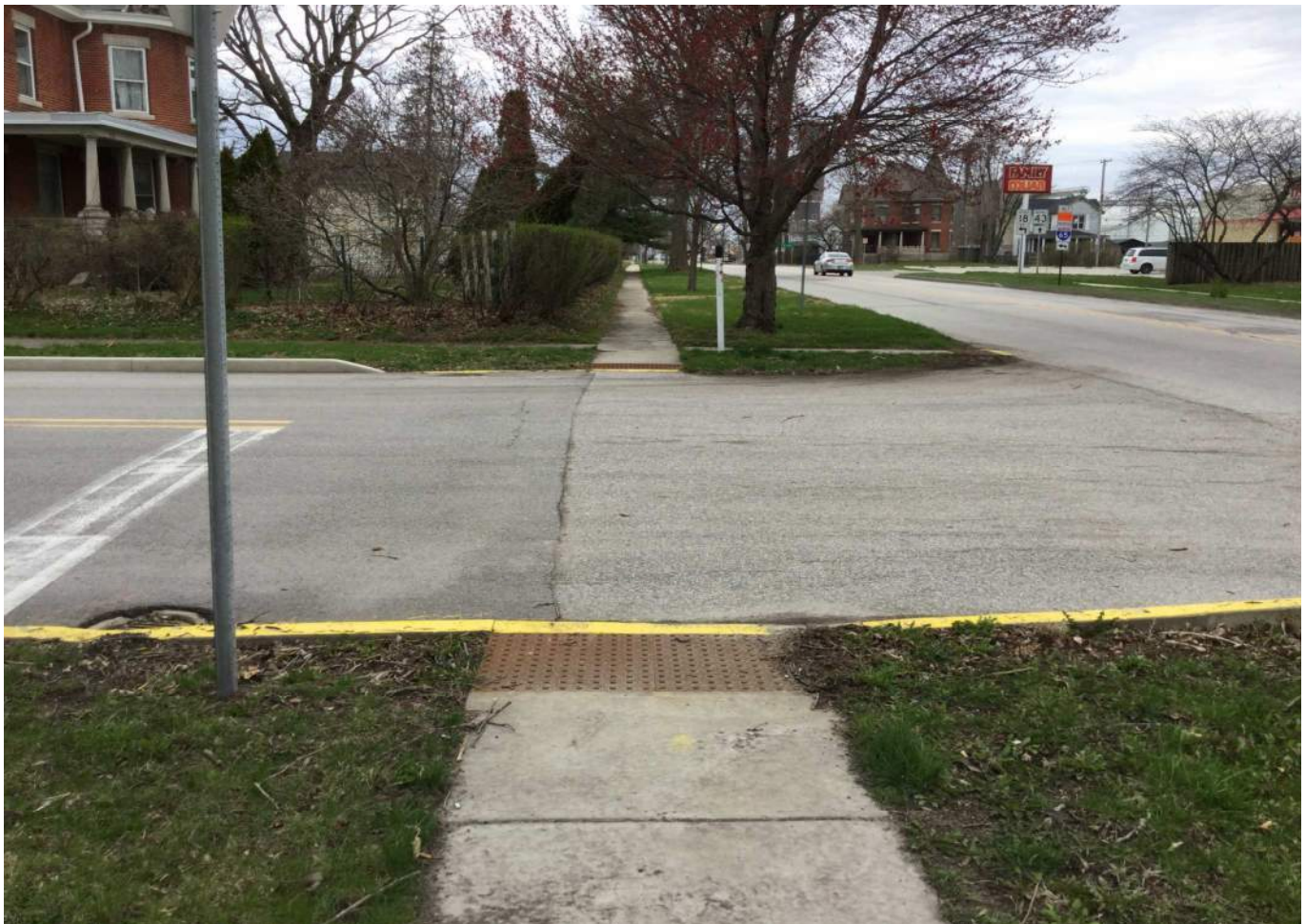
18. Looking north from the SR 18 / West 2 nd Street Intersection at existing sidewalk and curb ramps along the west side of SR 18.
