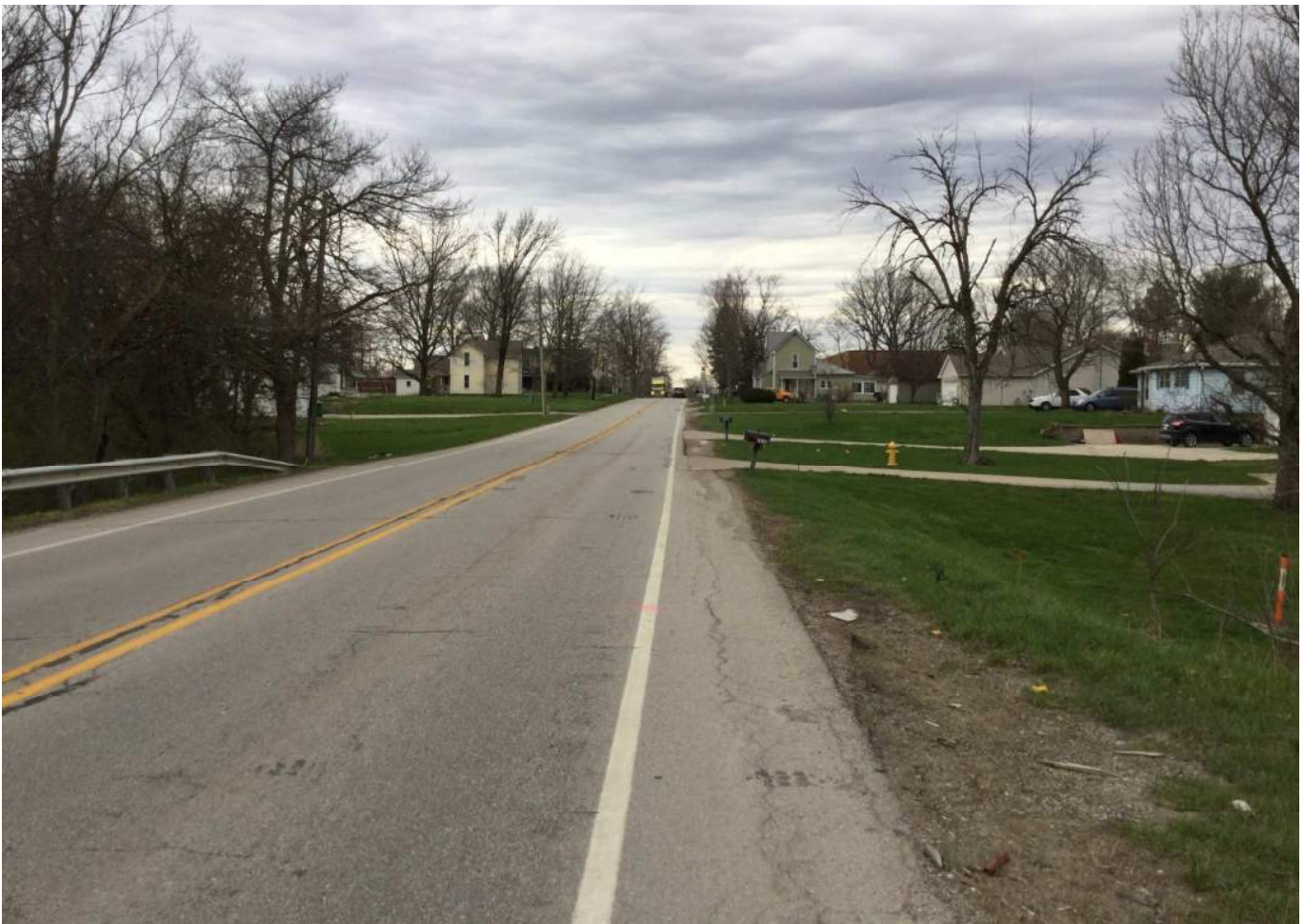
42. Looking north from the southern project terminus at roadway and adjacent landscape.
