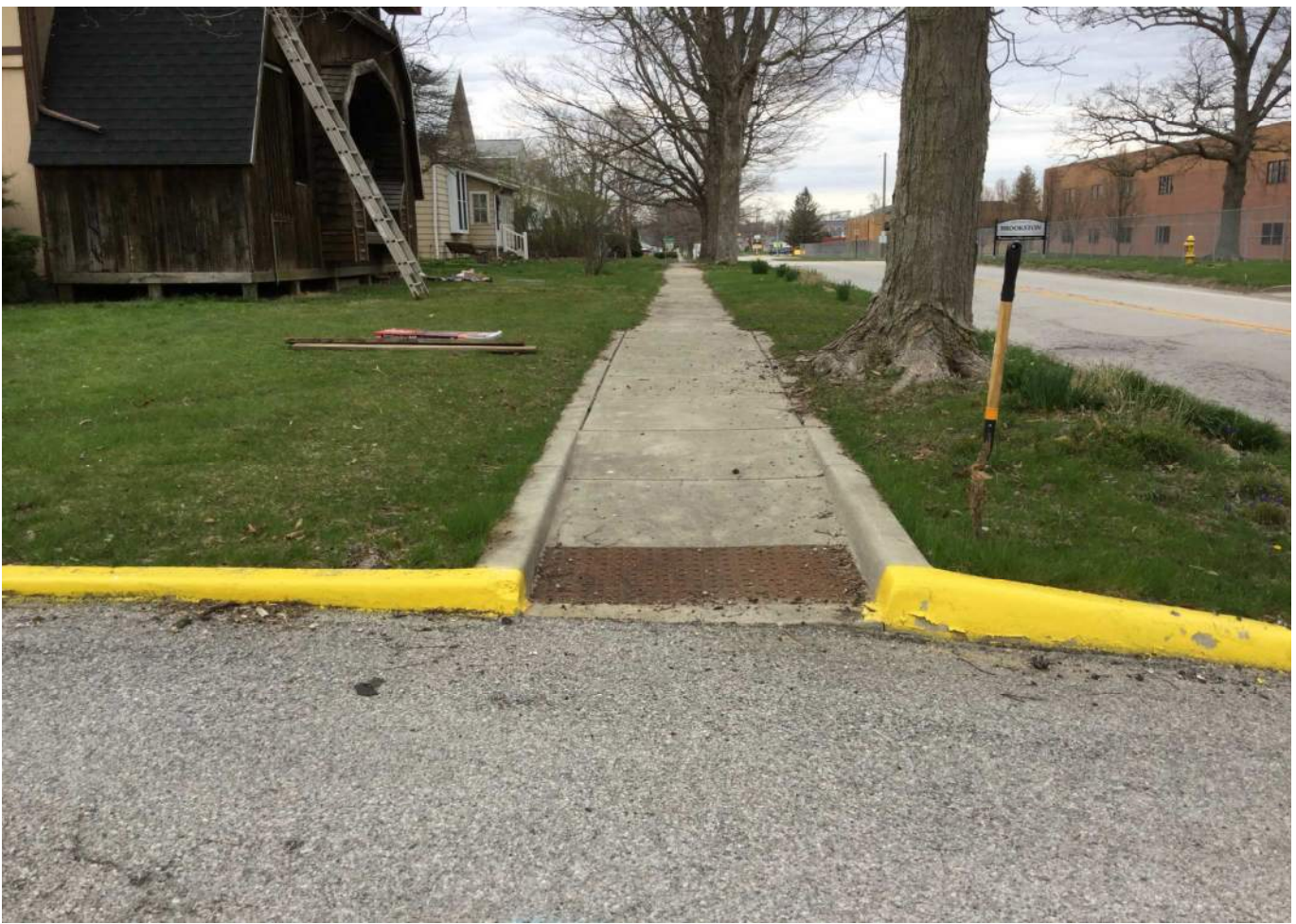
37. Looking north from the SR 43 / West 10 th Street Intersection at existing sidewalk and curb ramp along the west side of SR 43.
