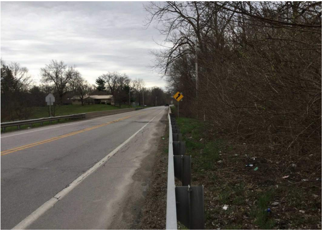
43. Looking south from the southern project terminus at the Moots Creek Bridge approach demarcating the southern project terminus.
