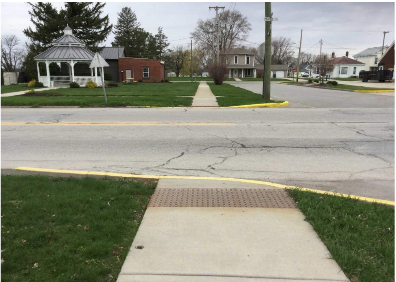
15. Looking west from the SR 18 / West 1 st Street Intersection at existing sidewalk, curb ramps, and Jaunita Park.
