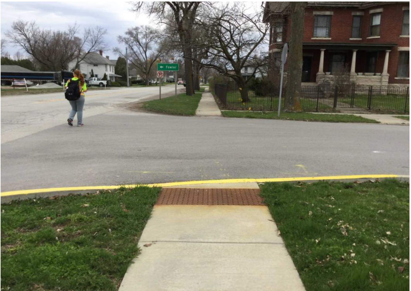
14. Looking north from the SR 18 / West 1 st Street Intersection at existing sidewalk and curb ramps along the east side of SR 18.
