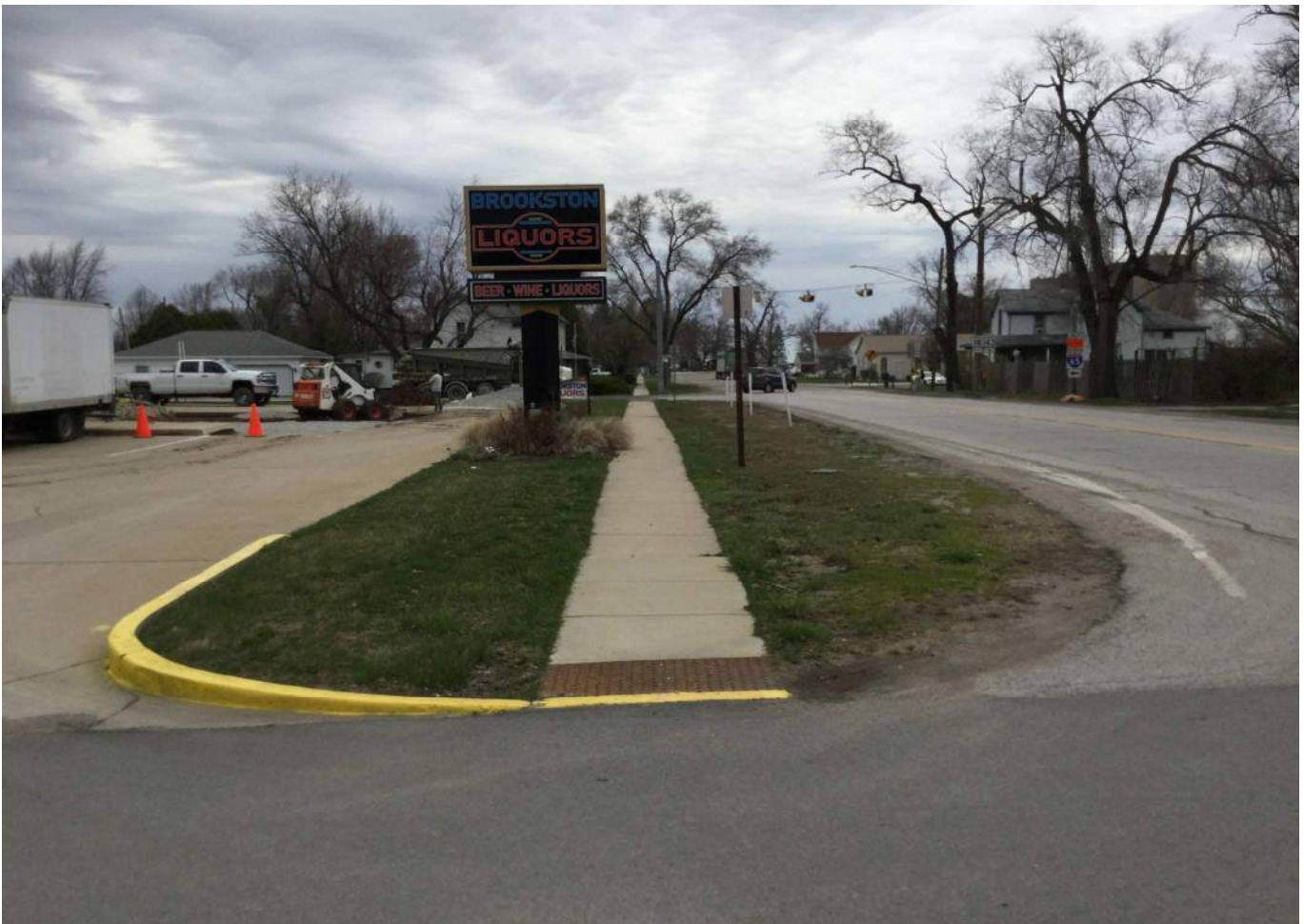
12. Looking north from the SR 18 / West 1 st Street Intersection at existing sidewalk and curb ramp along the west side of SR 18.
