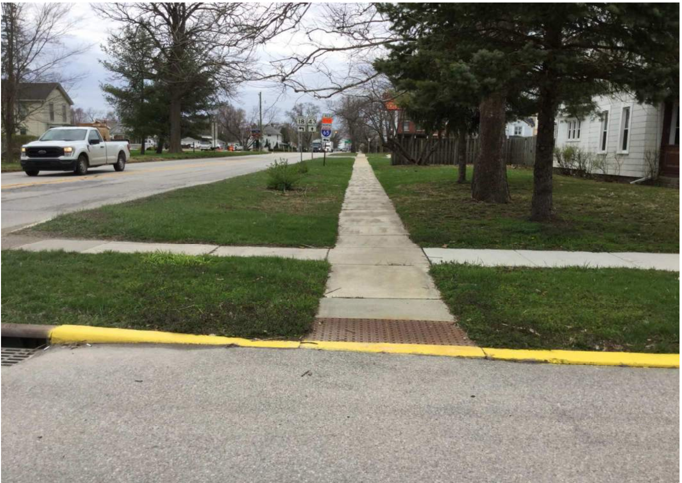
16. Looking north from the SR 18 / West 2 nd Street Intersection at existing sidewalk and curb ramp along the east side of SR 18.
