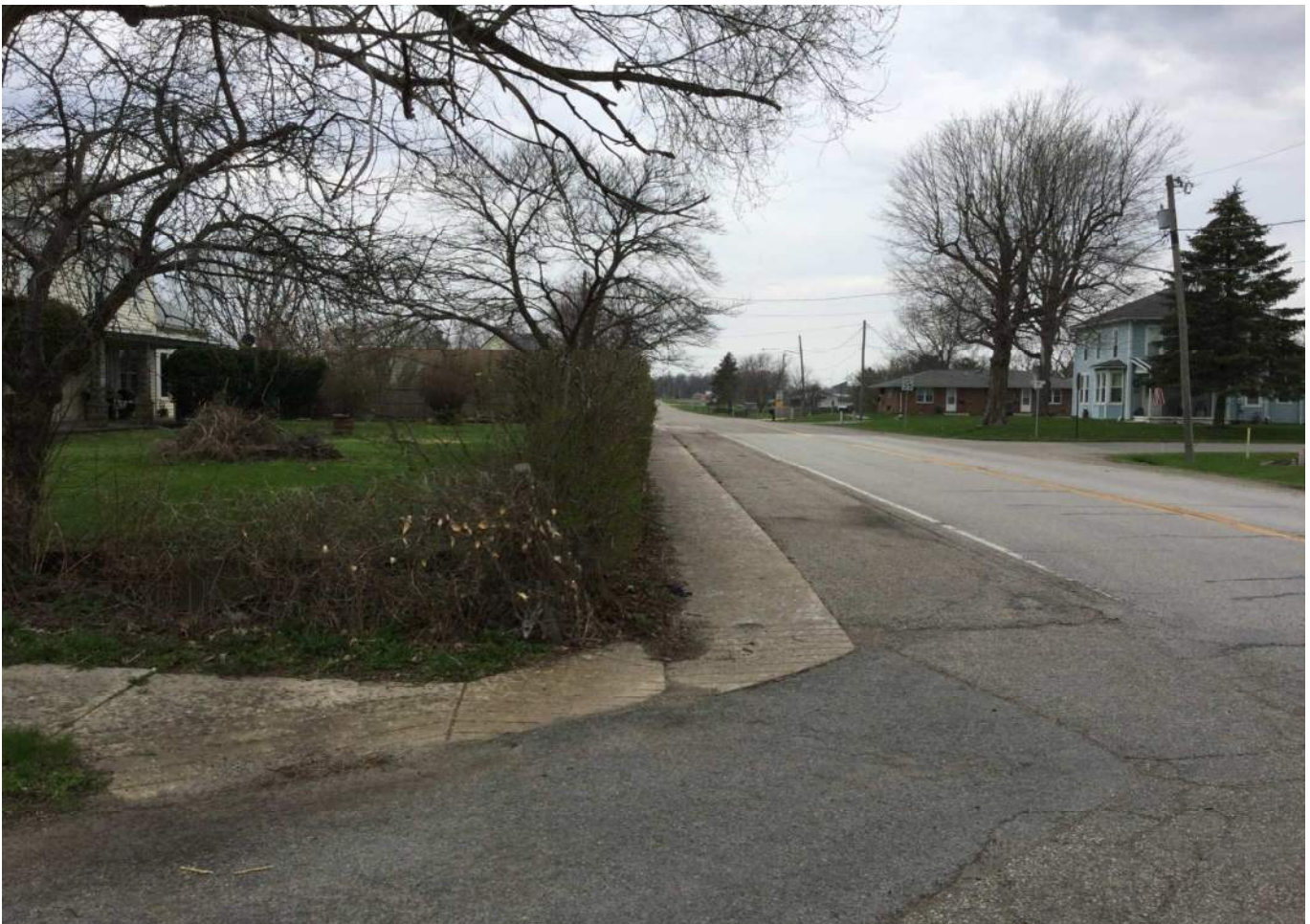
8. Looking west from the SR 18 / Ripley Street Intersection at existing sidewalk and curb ramp along the south side of Ripley Street.
