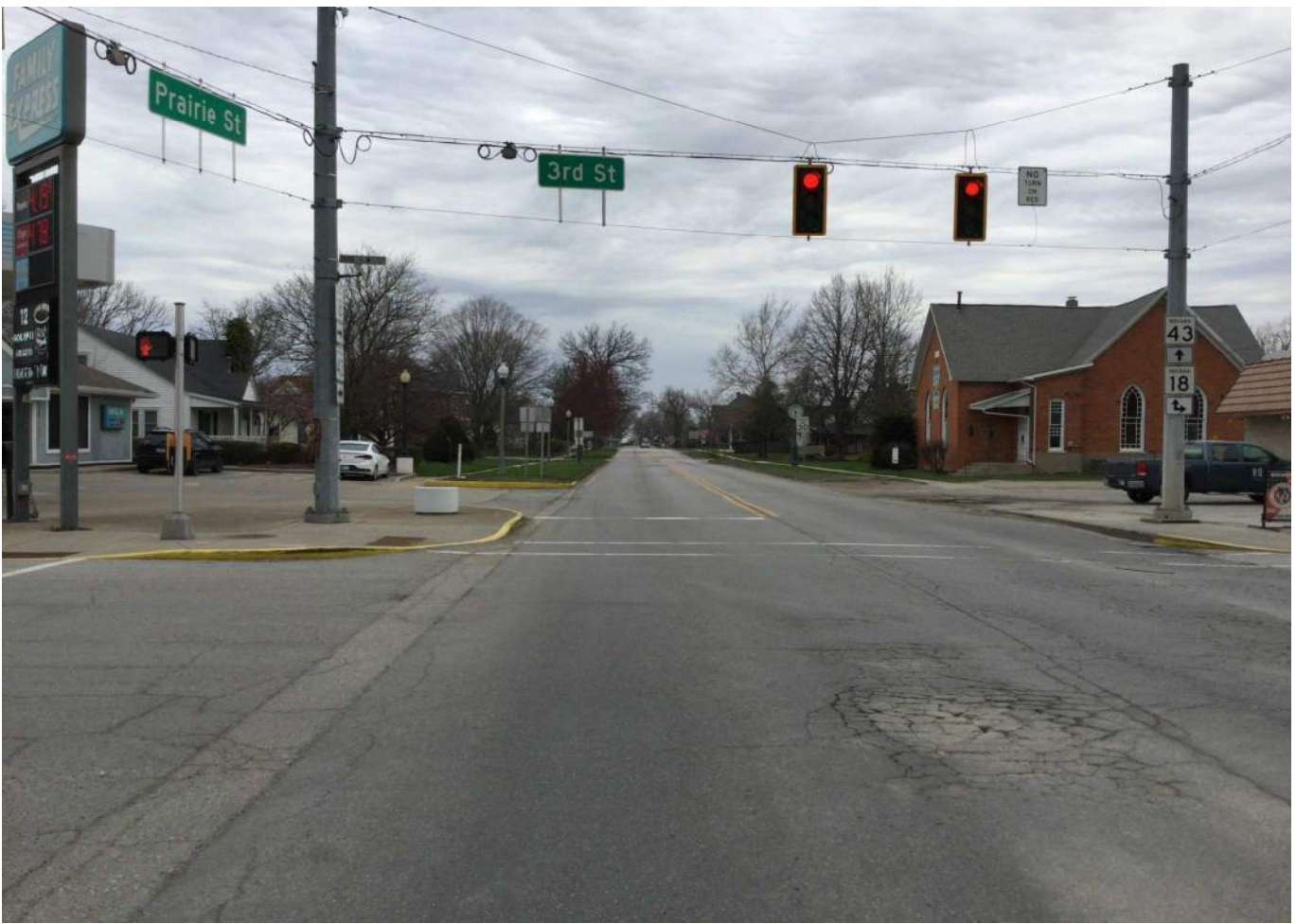
21. Looking north from the SR 18 South Junction / SR 43 Intersection at roadway and adjacent landscape.
