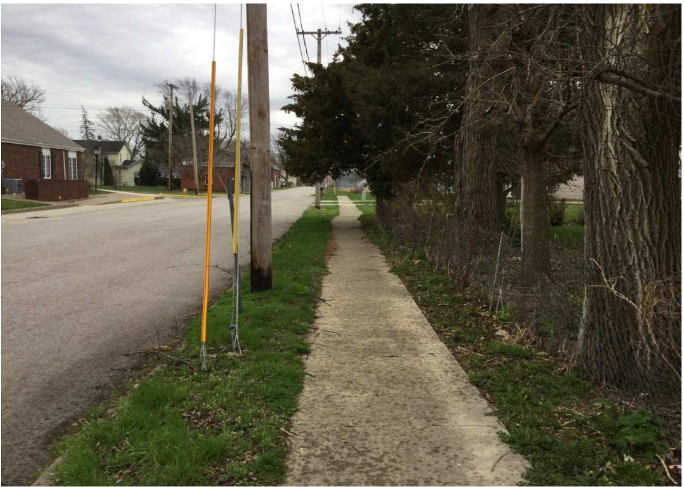
7. Looking south from the SR 18 / Ripley Street Intersection at existing sidewalk along the west side of Ripley Street.
