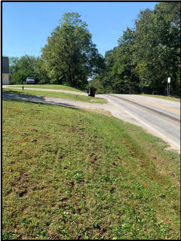
13. View of mowed ROW and driveway entrances along the south side of SR 258, looking west. 9/28/2021
