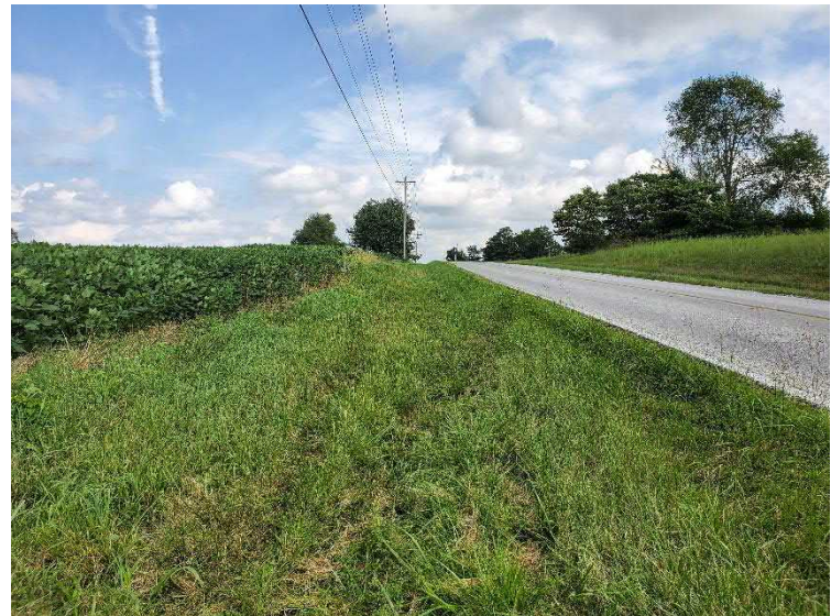
Photo 16: RSD 3 facing east
