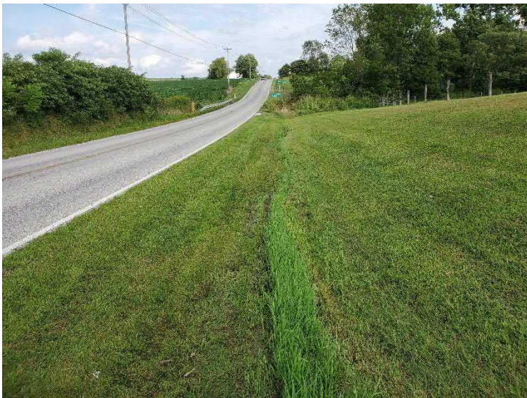
Photo 3: RSD 1 facing east
