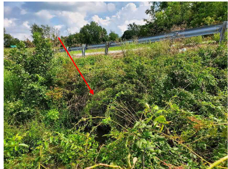
Photo 8: Culvert carrying UNT 1 north of SR 250 facing southeast
