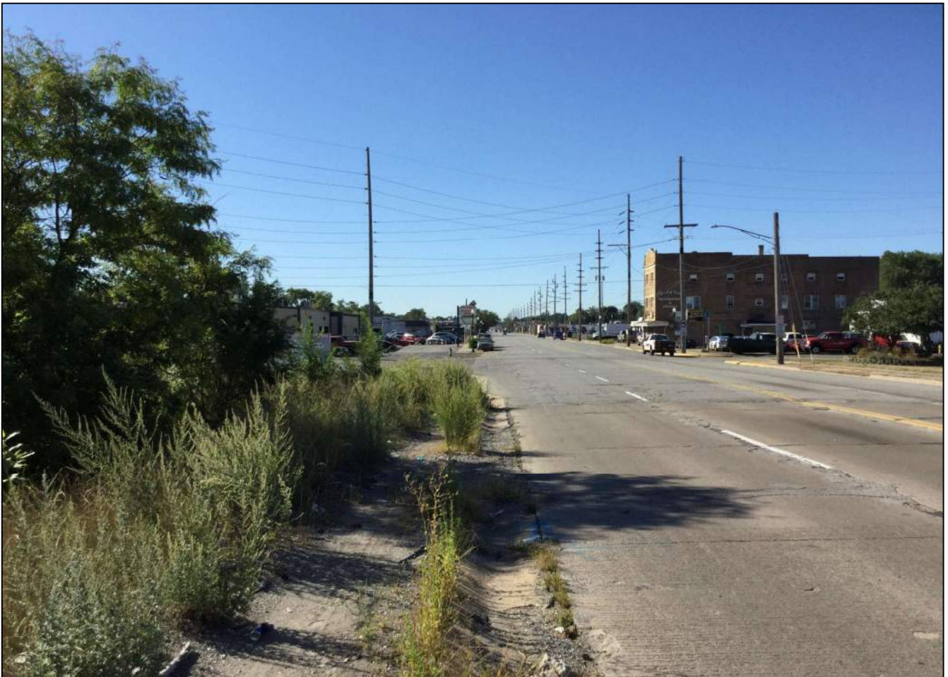
33. Looking south along the east side of Kennedy Ave. at the V gutter present and gravel shoulder.
