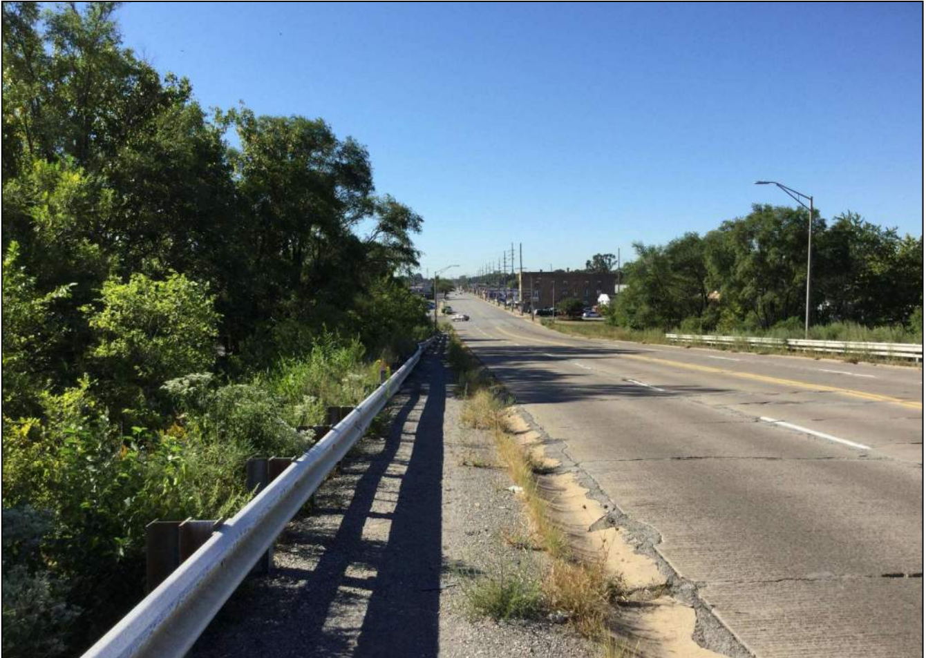
38. Looking south along the east side of Kennedy Ave. just south of County Bridge exempted from the project.
