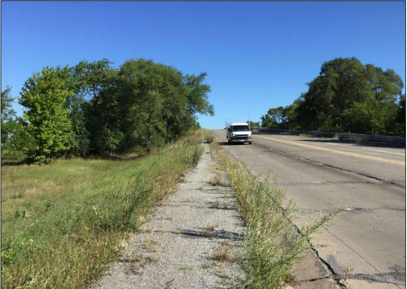
36. Looking north along the west side of Kennedy Ave. at the V gutter present and gravel shoulder.
