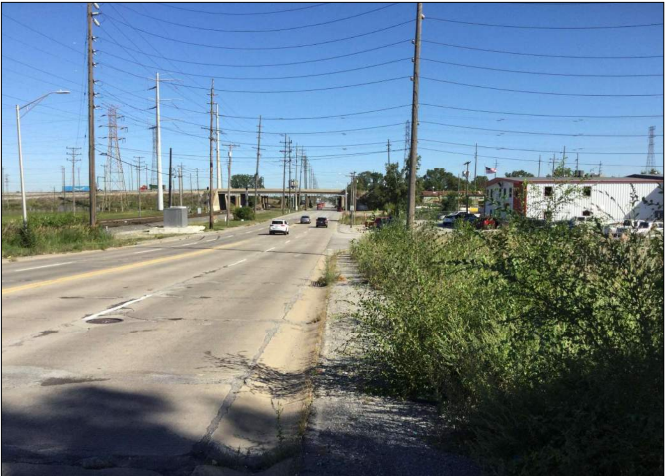
41. Looking north along the east side of Kennedy Ave.
