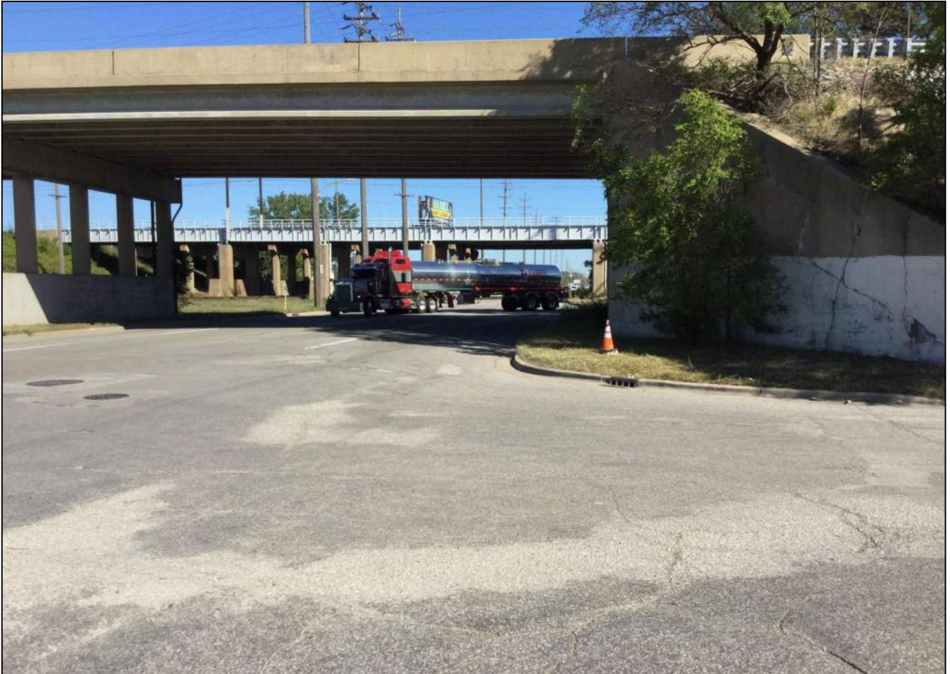
48. Looking northwest from the intersection of the south access road for US 20/Michigan St. at the northern end of the project.
