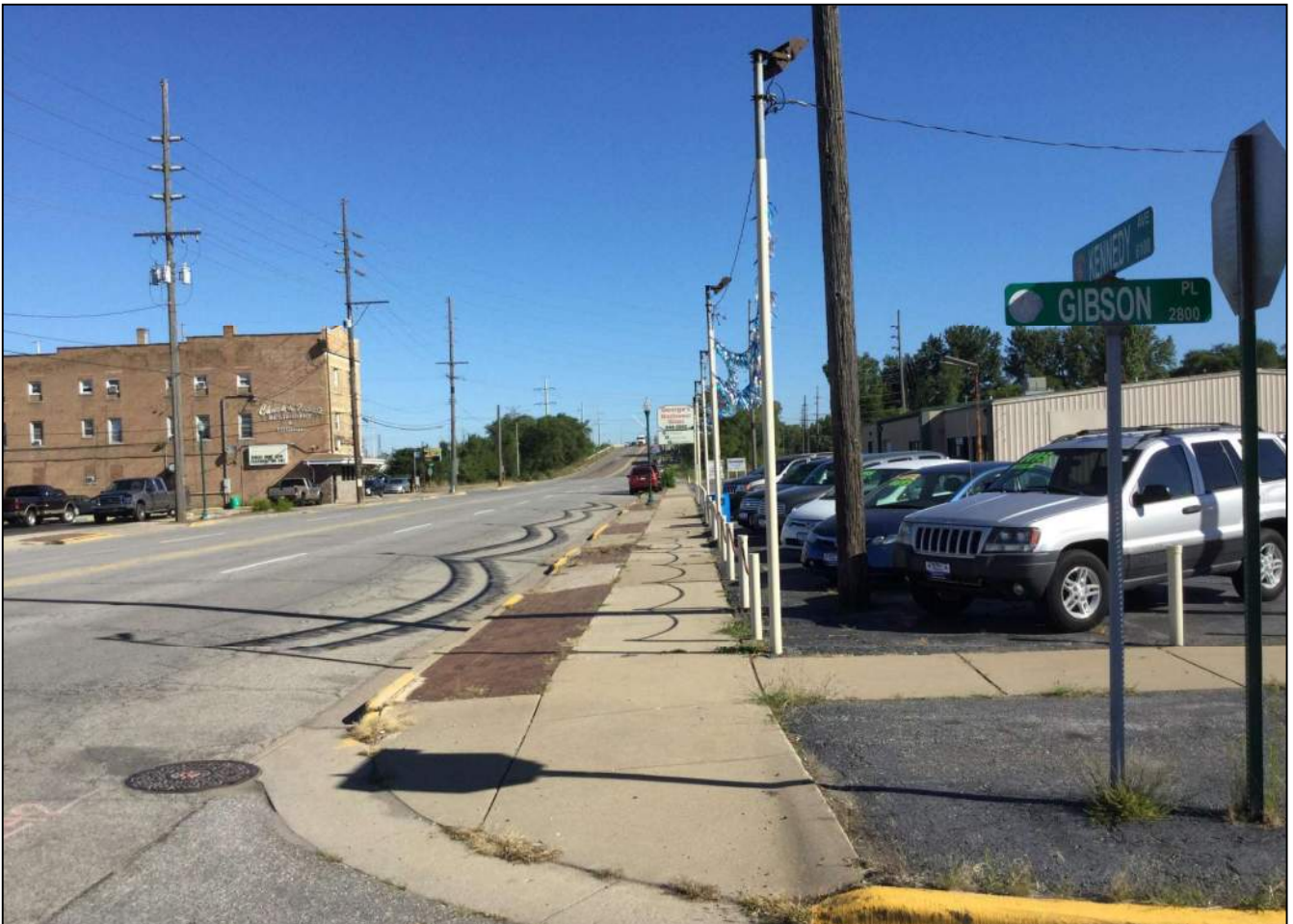
25. Looking north along the east side of Kennedy Ave. and sidewalk from the Gibson Pl. and Kennedy Ave. intersection.
