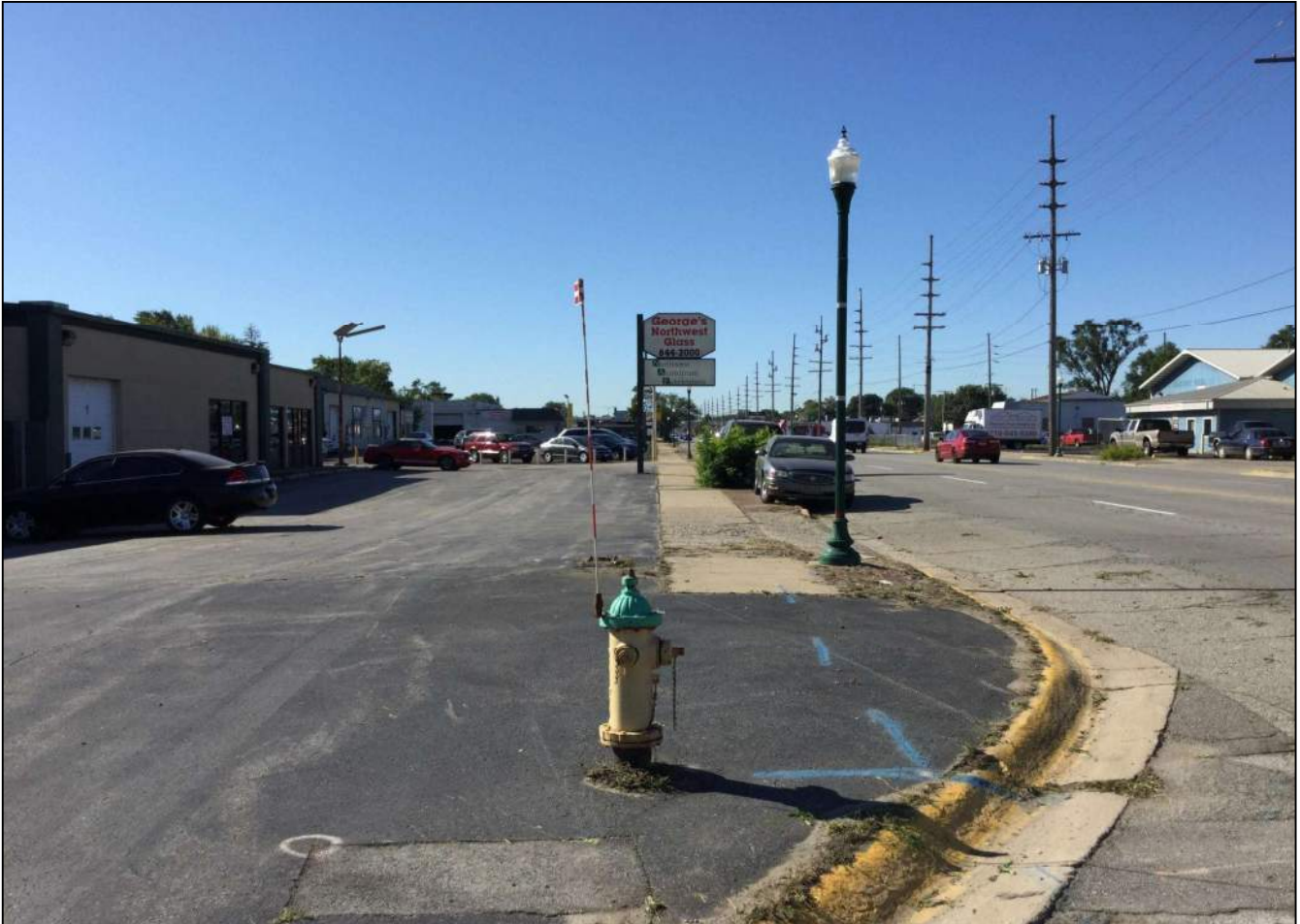
28. Looking south along the east side of Kennedy Ave. and partial sidewalk from the Gibson Transfer Rd. and Kennedy Ave. intersection.
