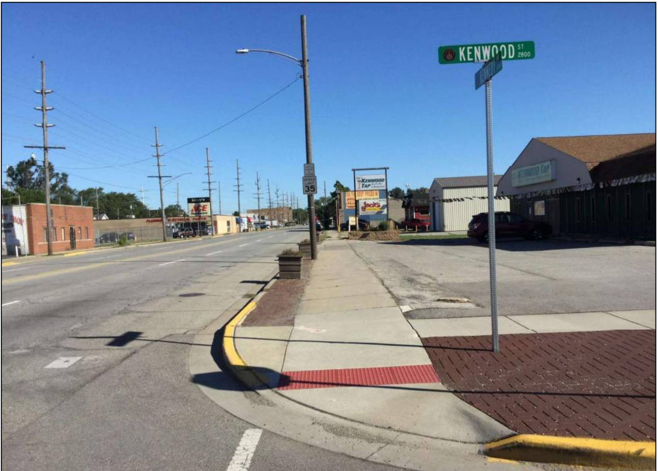
15. Looking north along the east side of Kennedy Ave. and sidewalk from the Kenwood St. and Kennedy Ave. intersection.
