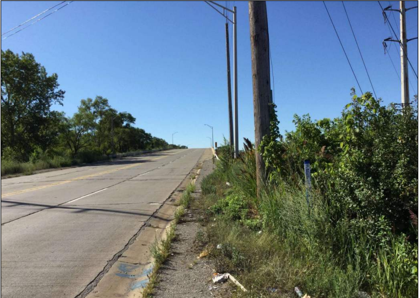
42. Looking south along the west side of Kennedy Ave.
