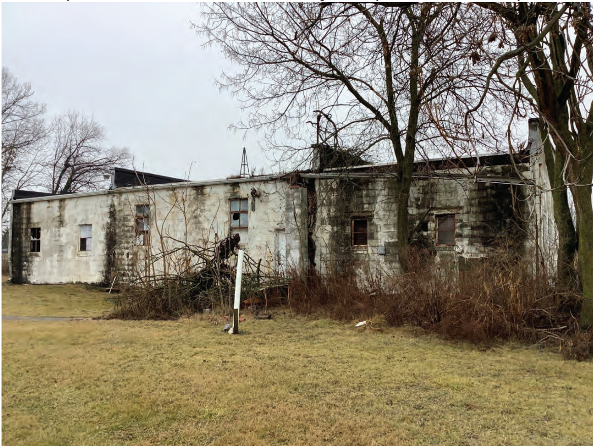
3. Looking NW at Lochmueller #1 (Contributing, 2904 S 1050 E)
