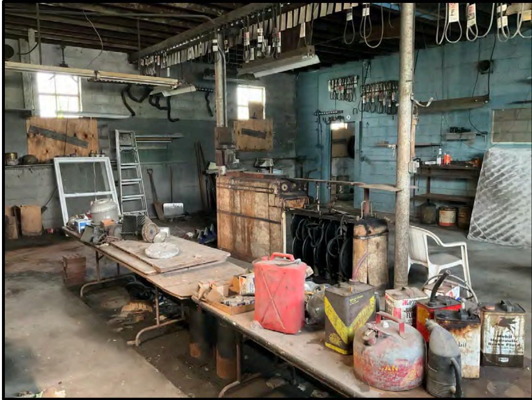
Figure 8: Looking SW inside Lochmueller #1 in center service bay
