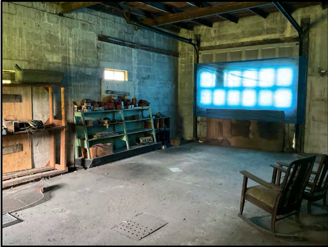
Figure 6: Looking NW inside Lochmueller #1 in W service bay
