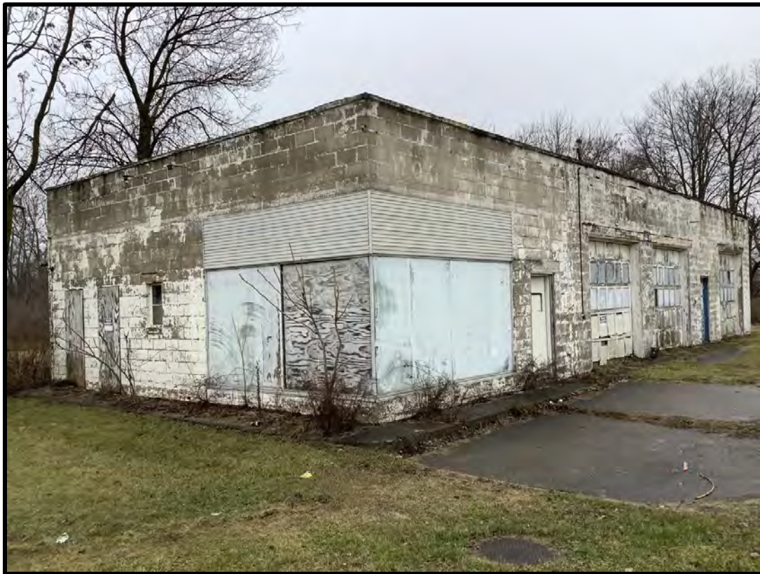
Figure 4: Looking SW at facade and E elevation of building.
