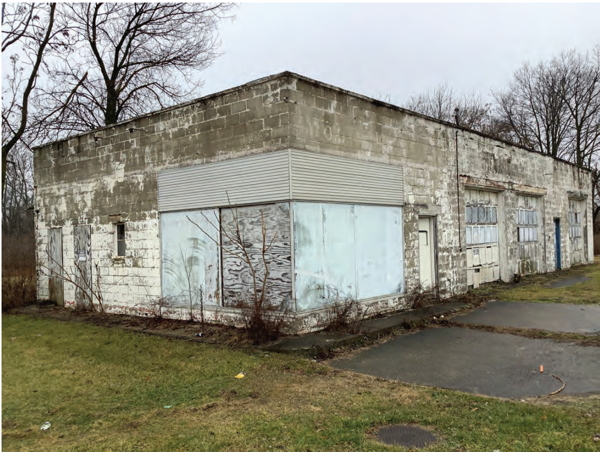
2. Looking SW at Lochmueller #1 (Contributing, 2904 S 1050 E)
