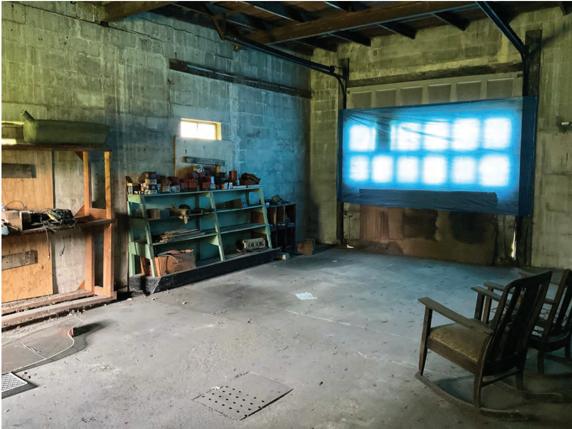
5. Looking NW in W service bay in Lochmueller #1 (Contributing, 2904 S 1050 E)
