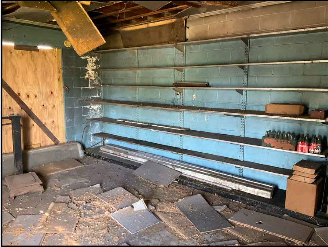
Figure 12: Looking SE inside Lochmueller #1 in service counter area, (E bay)
