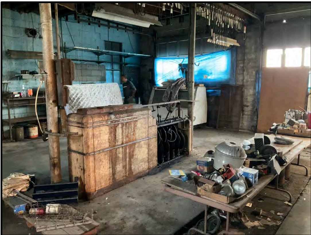
Figure 7: Looking NW inside Lochmueller #1 in center service bay
