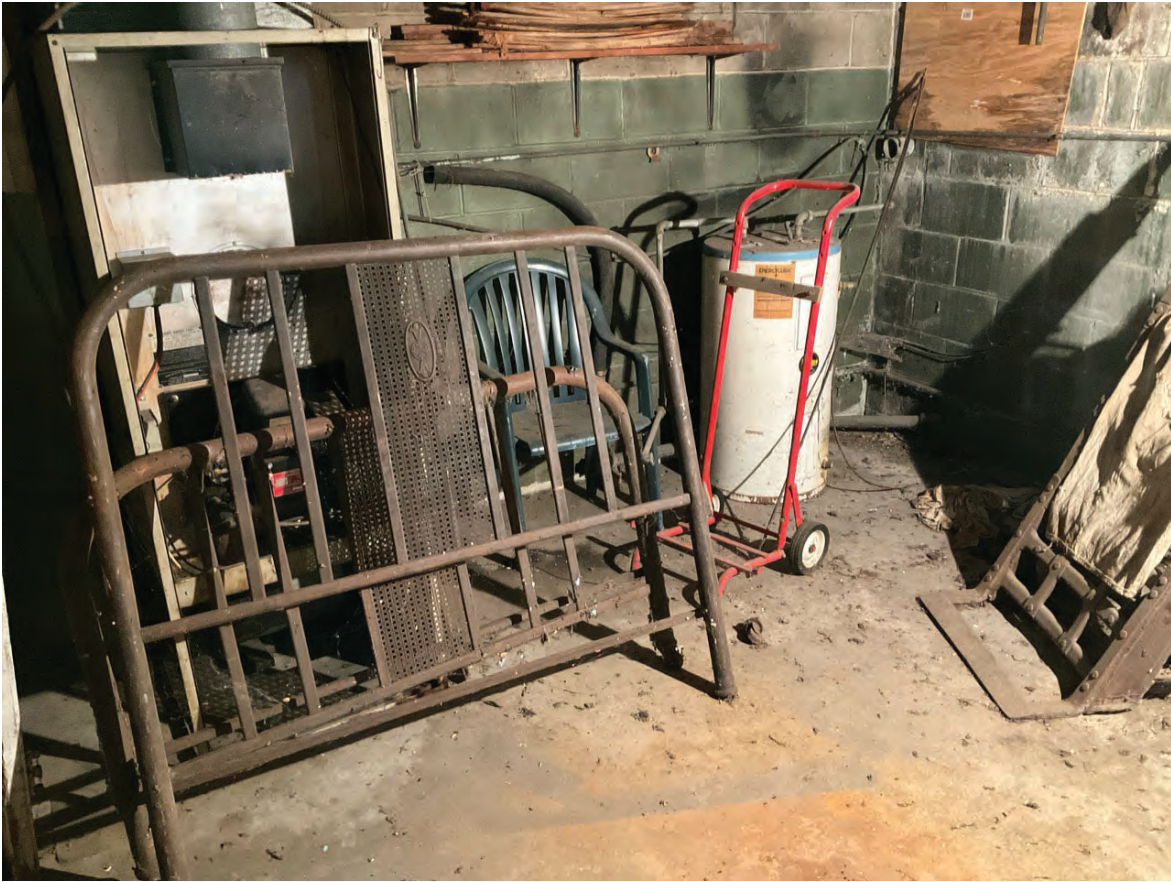
11. Looking SE in SE corner office in Lochmueller #1 (Contributing, 2904 S 1050 E)
