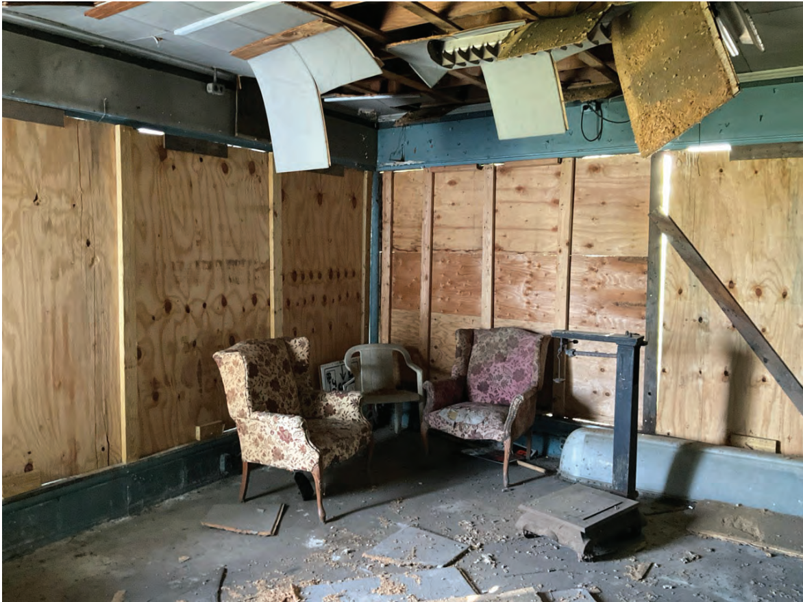
13. Looking NE in service counter area in Lochmueller #1 (Contributing, 2904 S 1050 E)
