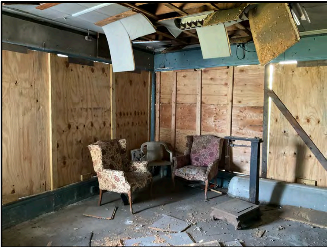
Figure 11: Looking NE inside Lochmueller #1 in service counter area
