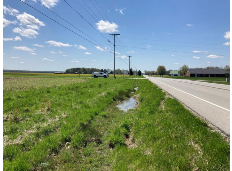
Photo 2: Looking westerly along US 50 east of intersection.
