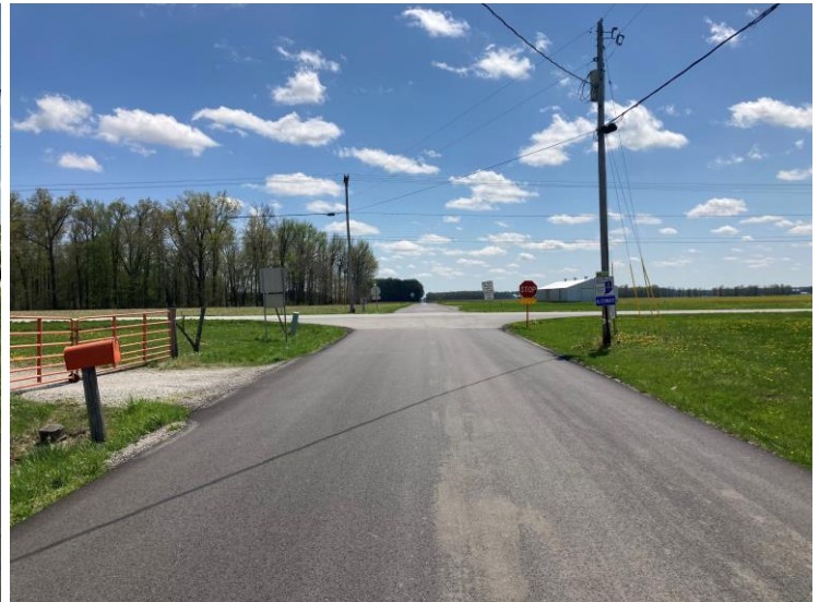
Photo 4: Looking southerly along Old Michigan Road north of intersection.
