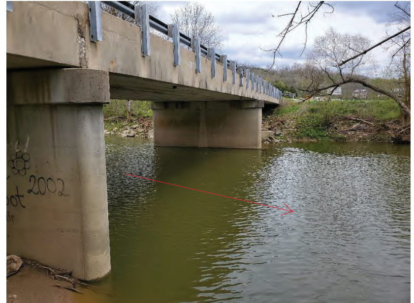
Photo 12: Laughery Creek Facing Northeast from South Side of Structure
