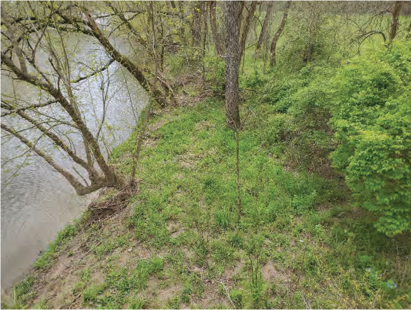
Photo 25: ROW of Structure On Southside Facing South
