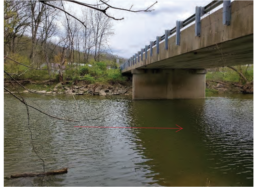
Photo 10: Laughery Creek Facing Southeast from Northside of Structure
