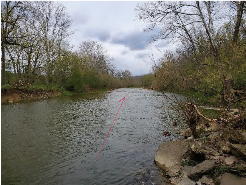
Photo 11: Laughery Creek Facing Southeast from South Side of Structure
