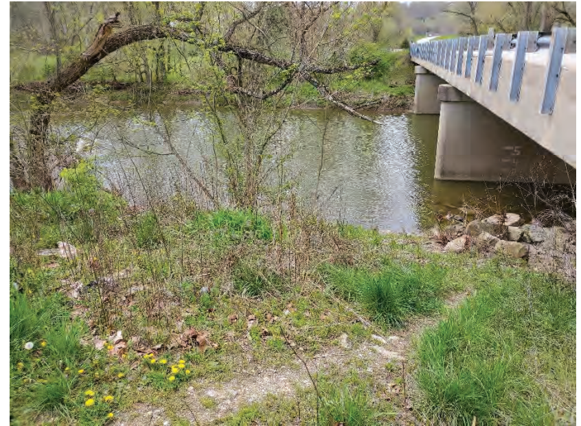
Photo 26: ROW of Structure On Northside Facing East
