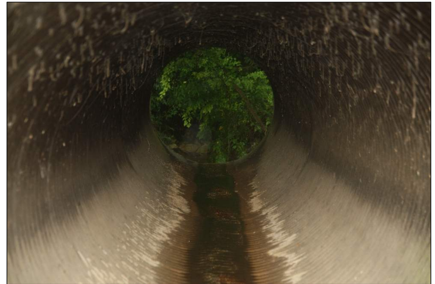
Photograph 4. View of inside of the structure.
