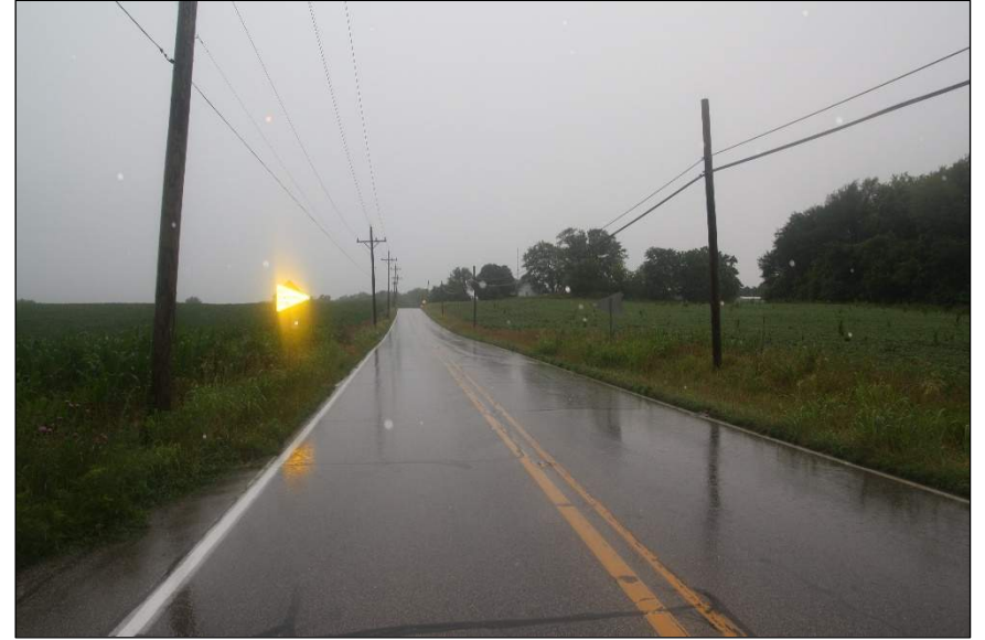
Photograph 6. View of existing roadway. Photo taken on western edge of project limits along SR 58, facing west.
