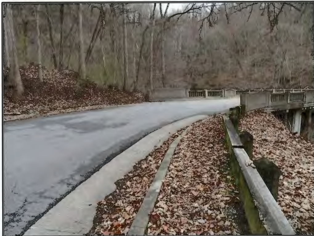
Figure 4. Overview of project area along Park Road/Canyon Road, facing northeast.
