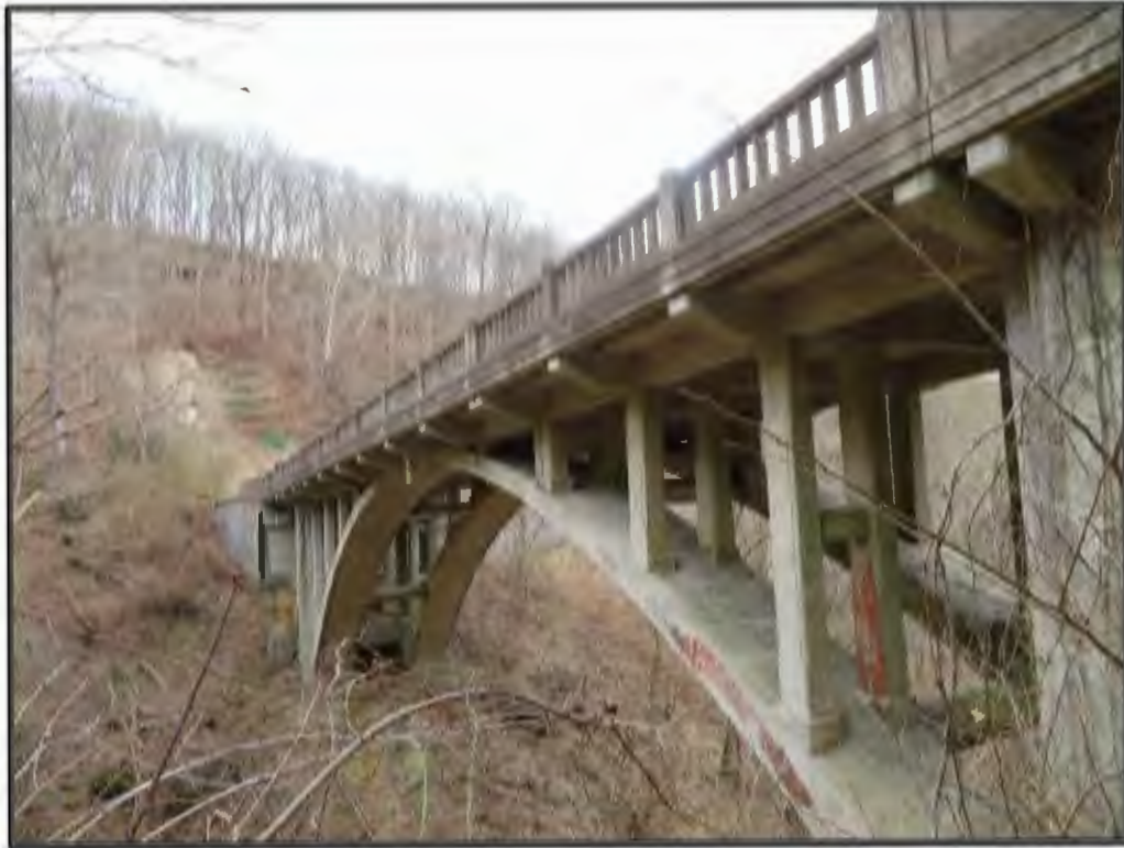
Figure 3. Overview of project area along Park Road/Canyon Road, facing southeast.
