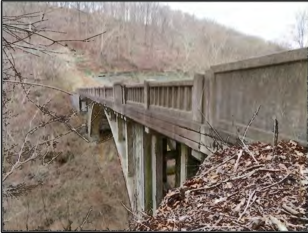
Figure 6. North elevation of the bridge (P000-39-06876B; NBI No. 60290), looking southeast.
