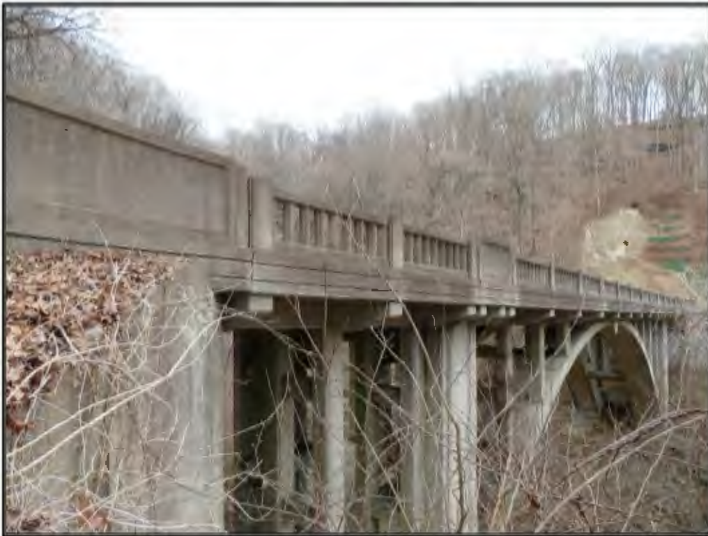
Figure 7. South elevation of the bridge (P000-39-06876B; NBI No. 60290), looking northeast.
