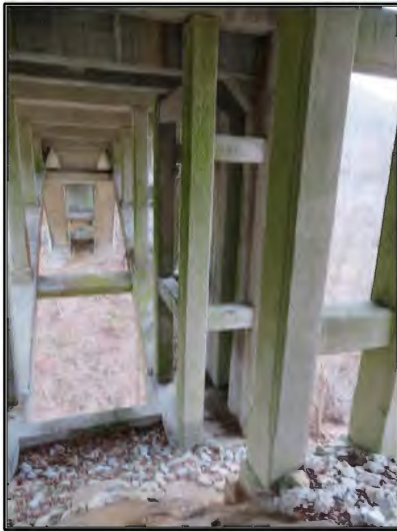
Figure 8. Substructure of the bridge (P000-39-06876B; NBI No. 60290), looking southeast.
