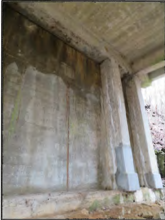
Figure 10. West concrete abutment of the bridge (P000-39-06876B; NBI No. 60290), looking northwest.
