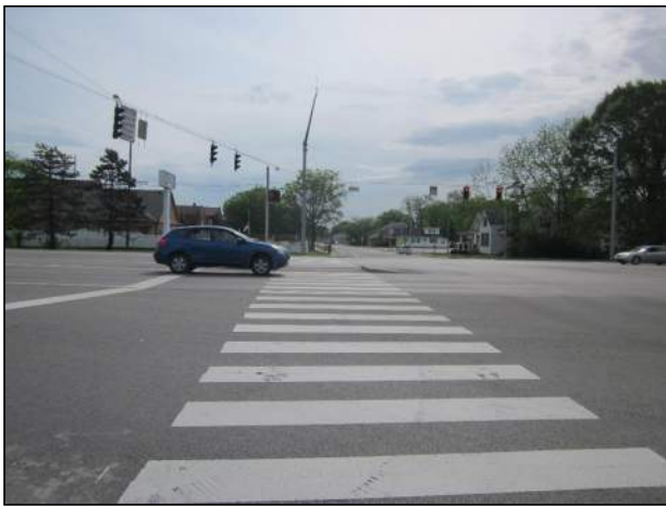
North Leg Crosswalk Looking East
