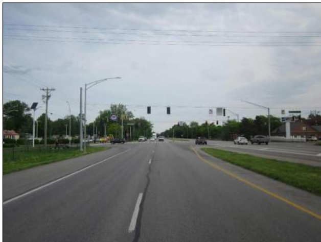
Southbound US 41 Looking North, South of Washington Ave
