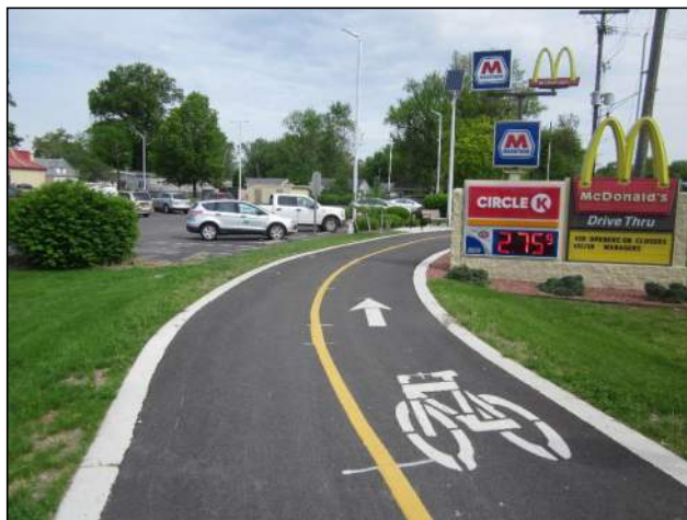
Multi-Use Path Along the West Side of US 41, Looking North
