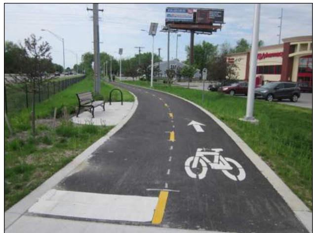
Multi-Use Path Along the West Side of US 41, Looking South
