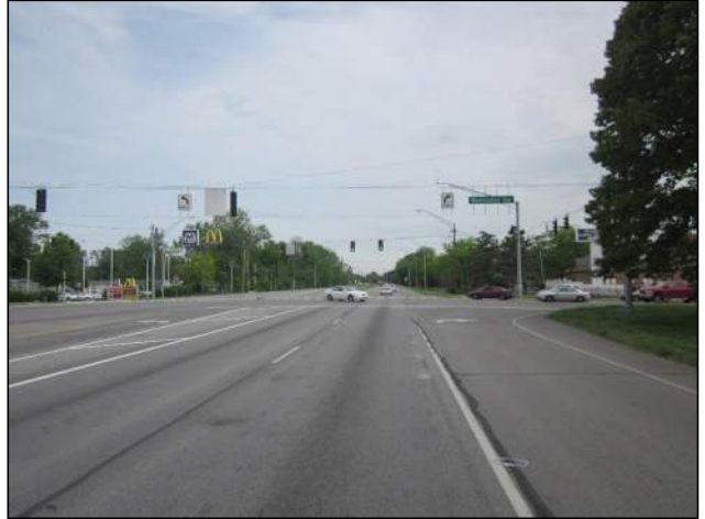
Northbound US 41 Looking North, South of Washington Ave
