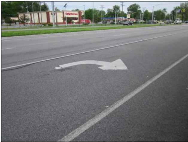
Pavement Markings in Northbound Right-Turn Lane
