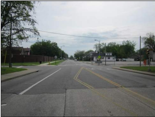
Washington Ave Looking East, East of US 41
