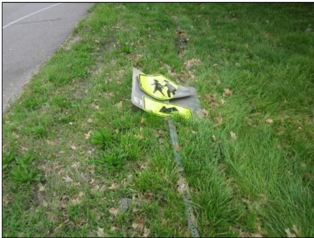
Fallen Pedestrian Crossing Sign on the SE Corner
