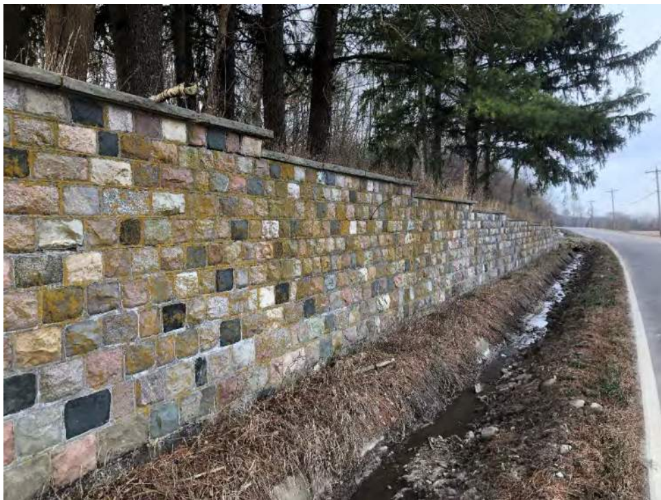
Figure 17. Detail of stone wall.
