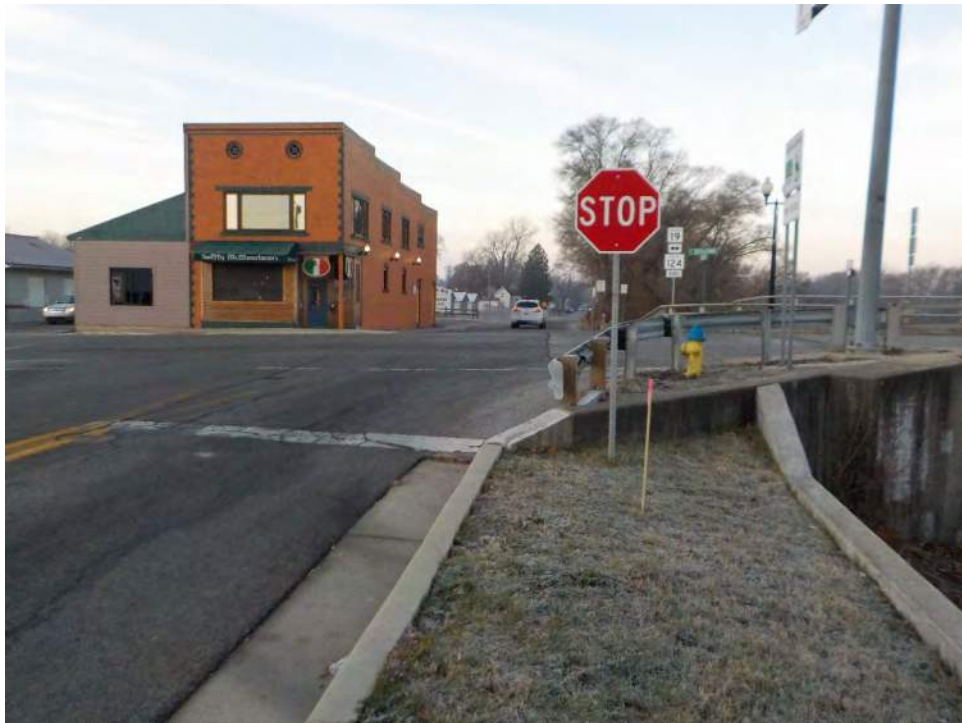
Figure 6. Intersection of SR 19 and SR 124, facing west.
