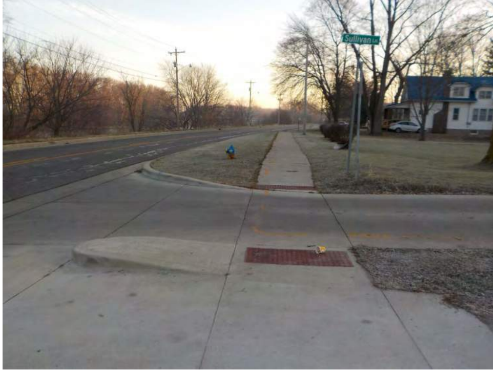
Figure 8. Intersection of SR 124 and Sullivan Lane, facing east.
