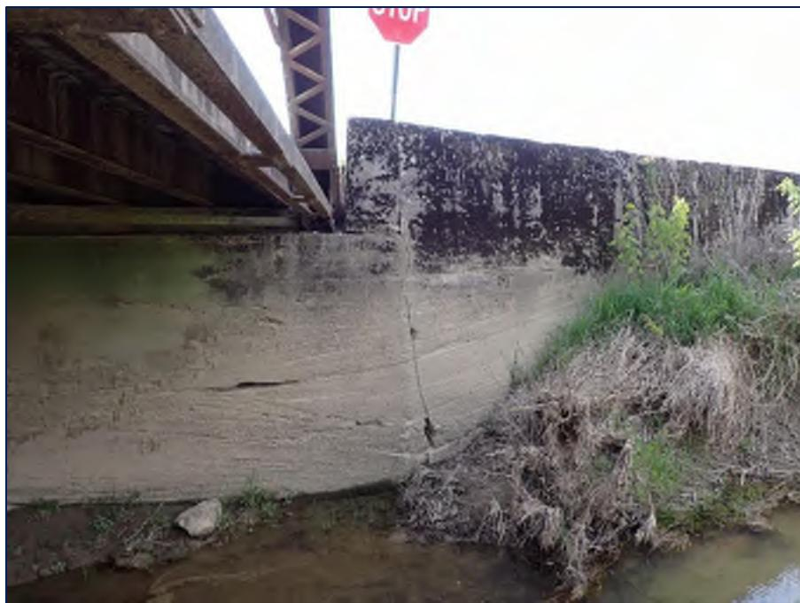
Photo 5. View of Crack in Northwest Wingwall
