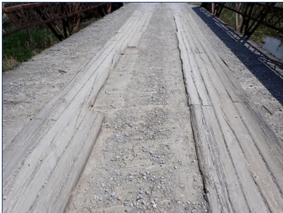
Photo 4. View of Jackson County Bridge No. 197 Wearing Surface (Bridge Deck)
