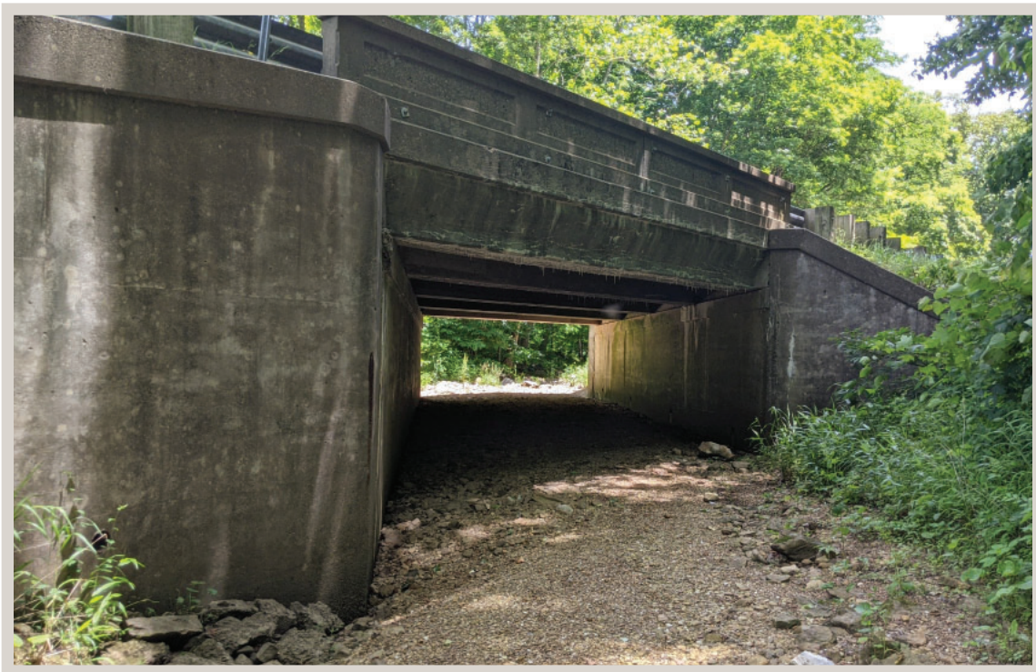
Photo 4: Looking northeast (downstream) of Bridge # (158)58-47-03027.
