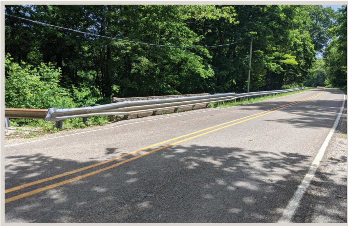
Photo 1: Looking southeast at Private Drive along Bridge # (158)58-47-03027.
