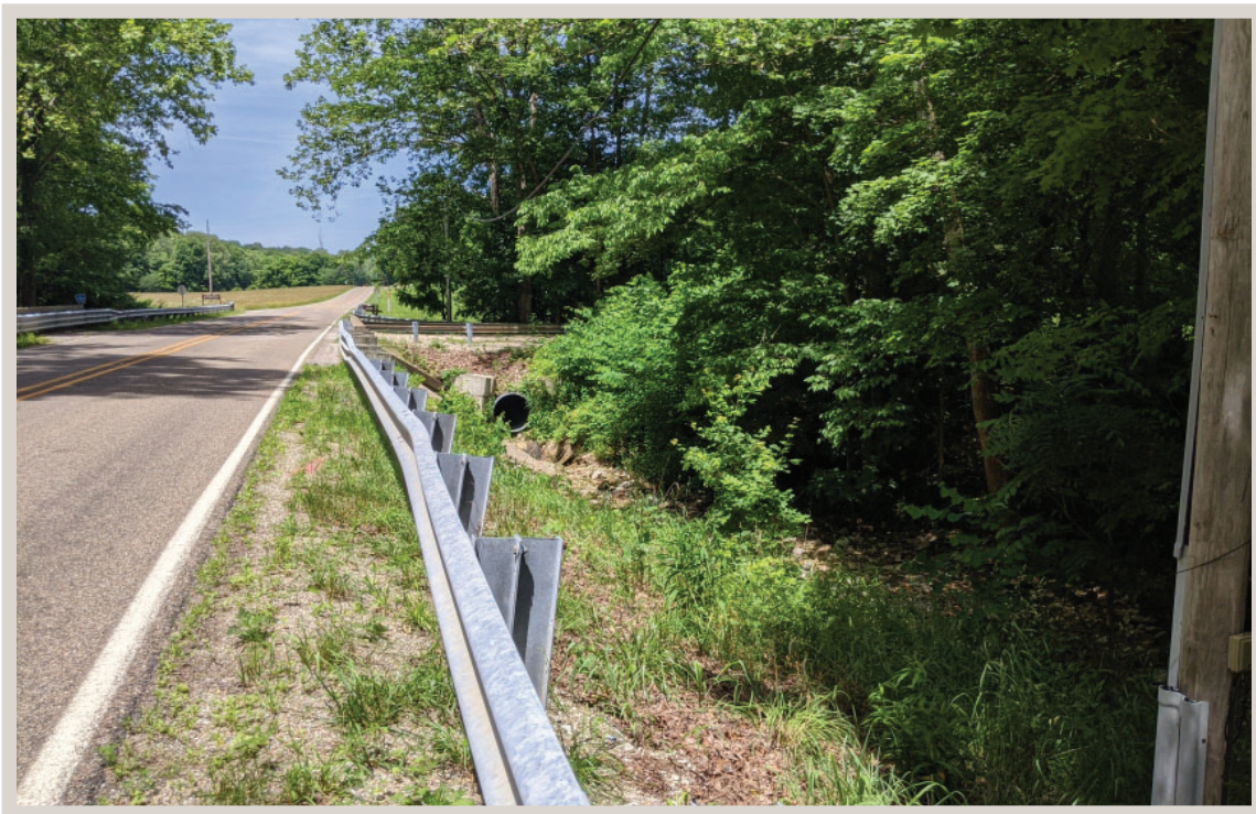
Photo 2: Looking northwest at CMP underneath north side of Private Drive.
