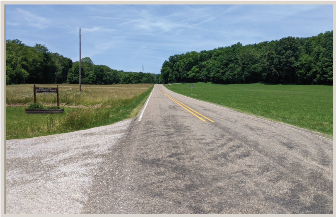
Photo 5: Looking northwest along SR 158 away from Bridge # (158)58-47-03027 near Graded Road.
