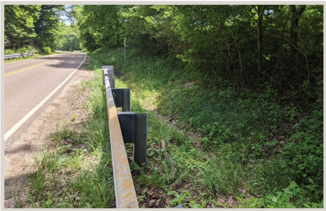
Photo 6: Looking southeast towards SR 158 along Bridge # (158)58-47-03027.
