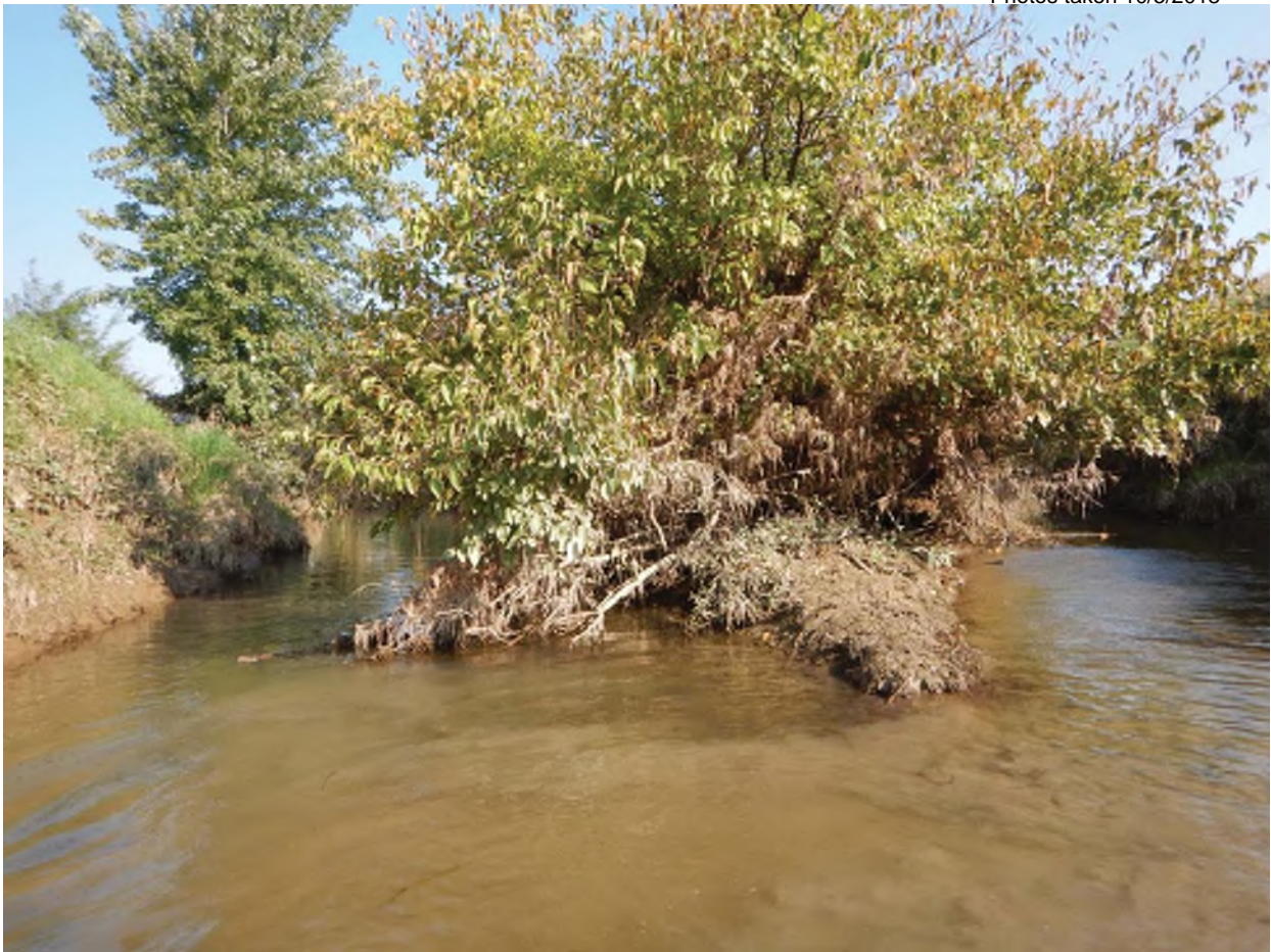
11. Facing north towards fork in Pollard Ditch downstream from bridges
