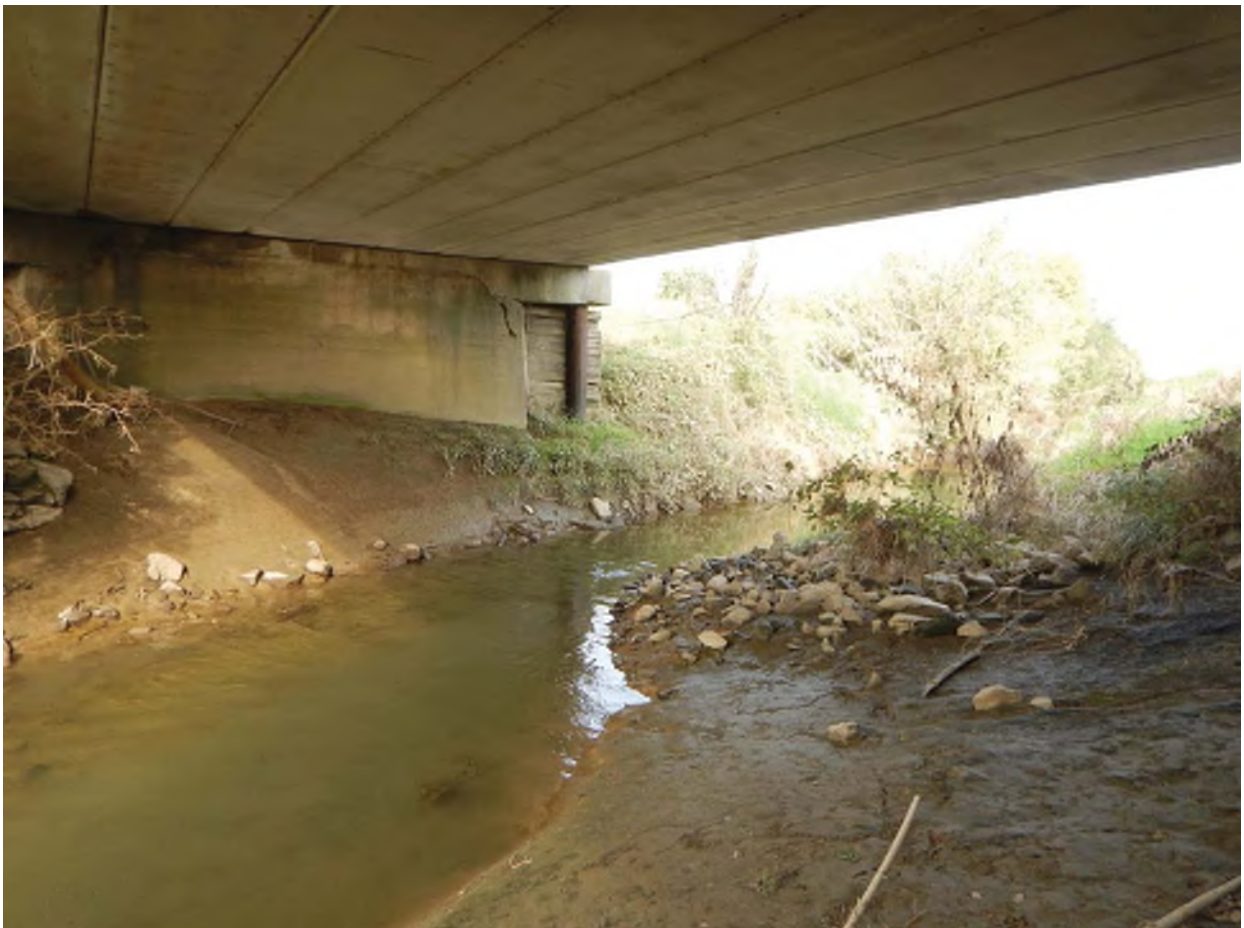
6. Facing northwest under bridge over Pollard Ditch
