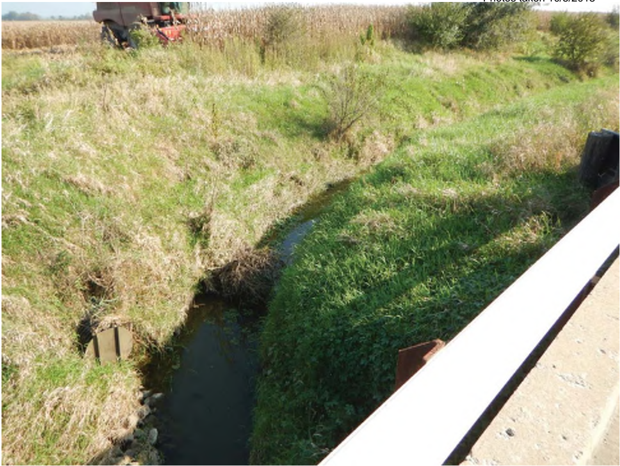
15. Facing northeast towards UNT to Pollard Ditch from bridge
