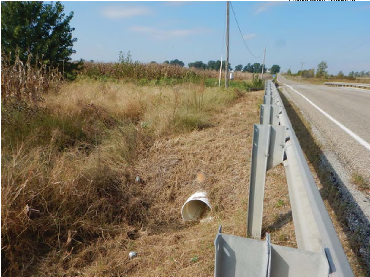
23. Facing west towards SR 58 and drive culvert
