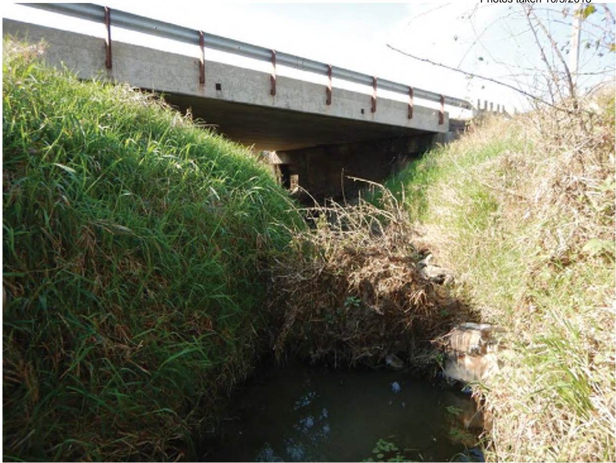
19. Facing southwest towards bridge over UNT to Pollard Ditch east
