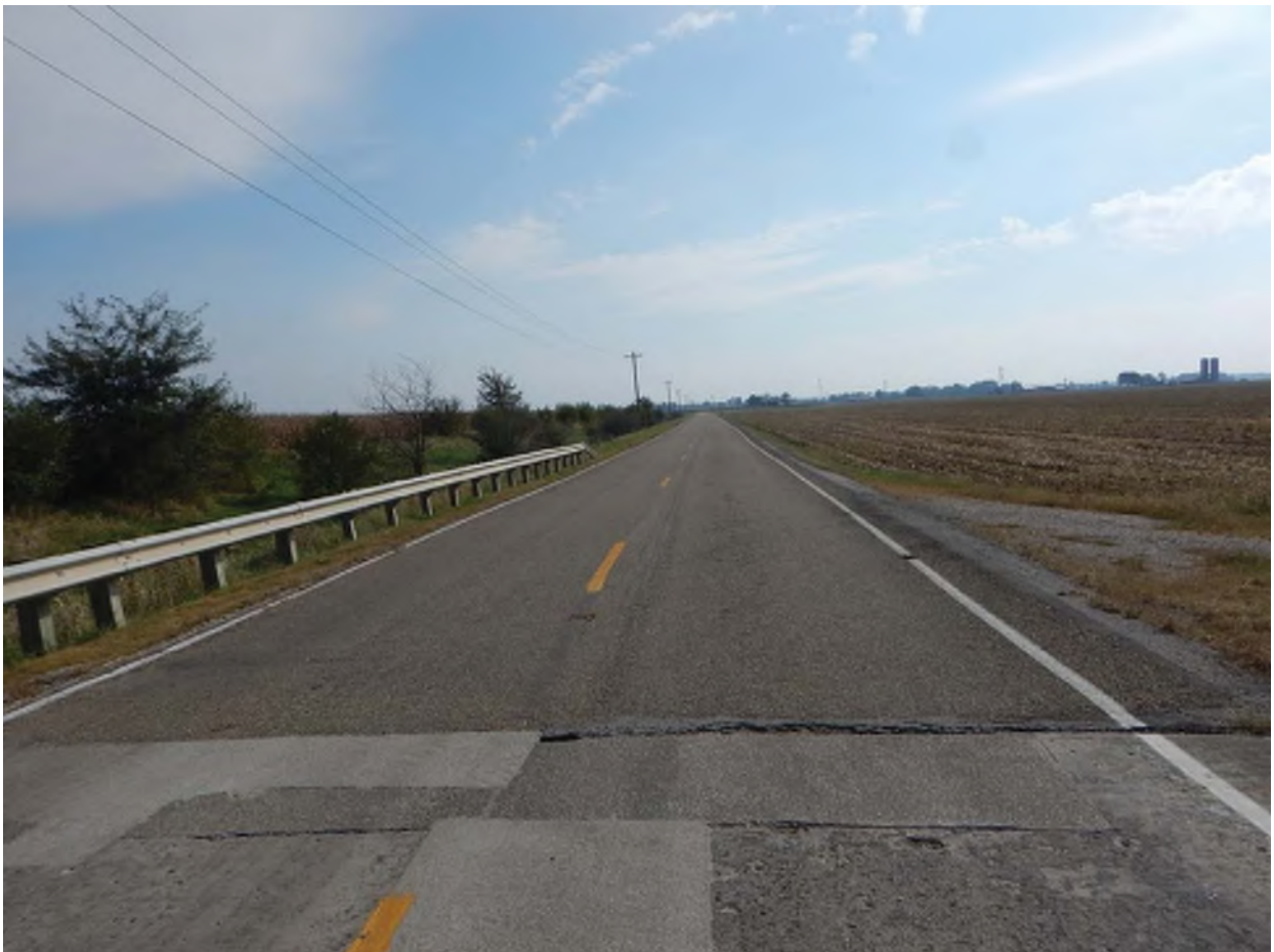
22. Facing east towards SR 58 from bridge
