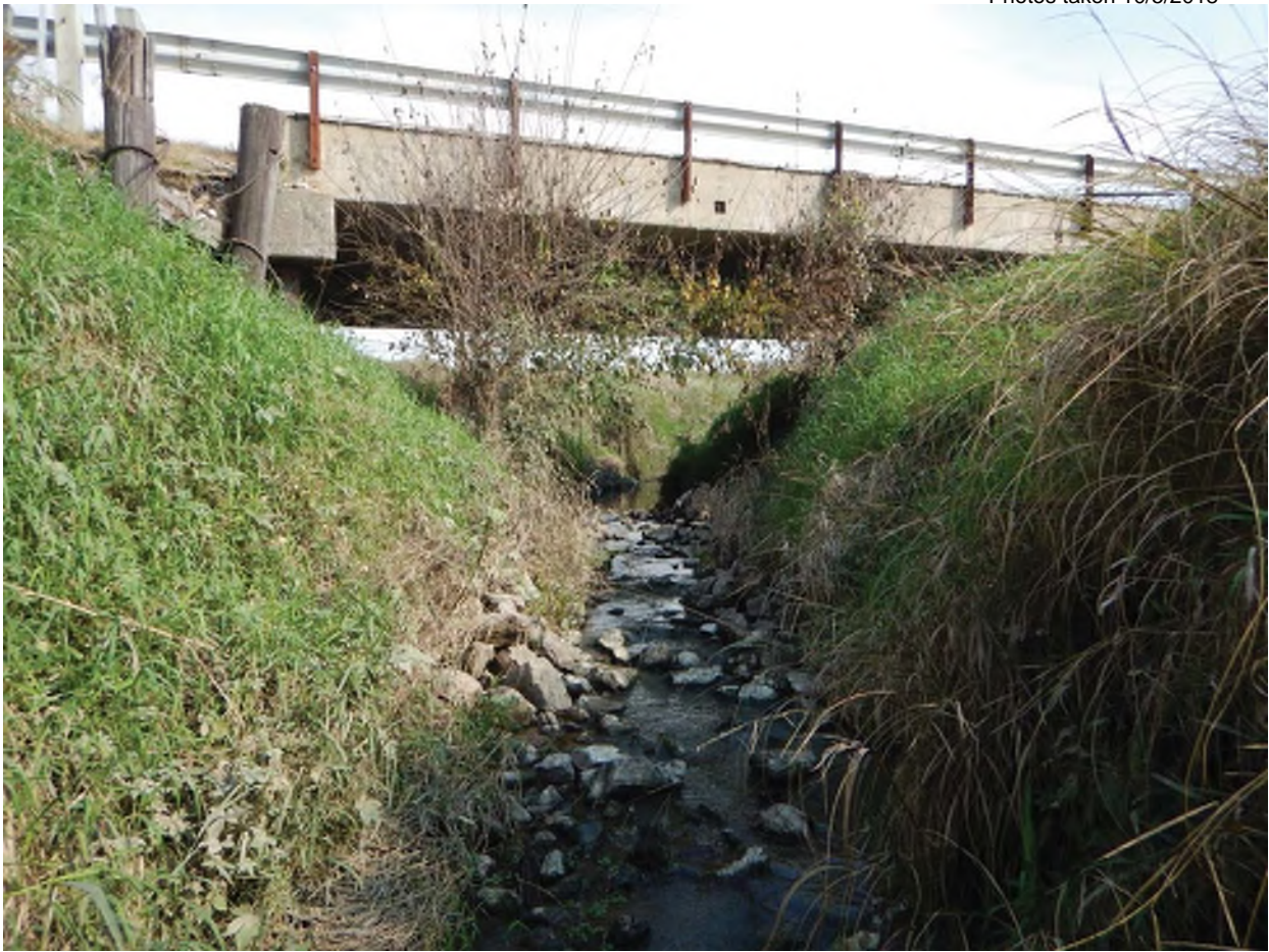
21. Facing northeast towards bridge over UNT to Pollard Ditch downstream
