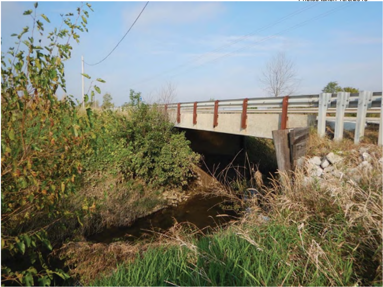
7. Facing northwest towards bridge over Pollard ditch
