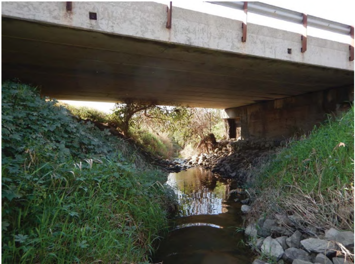
20. Facing southwest under bridge over UNT to Pollard Ditch east
