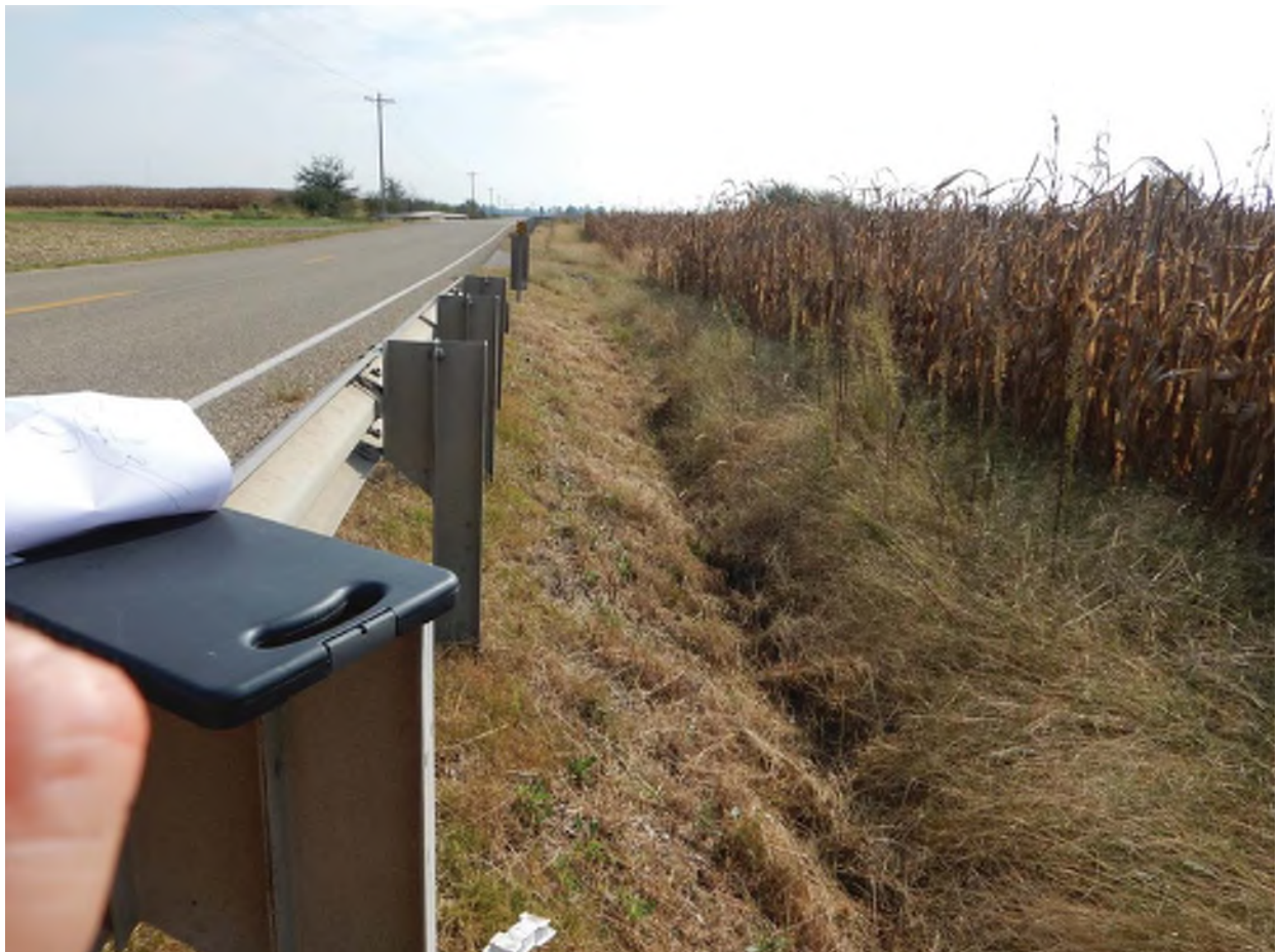
24. Facing east towards SR 58 and bridge structure
