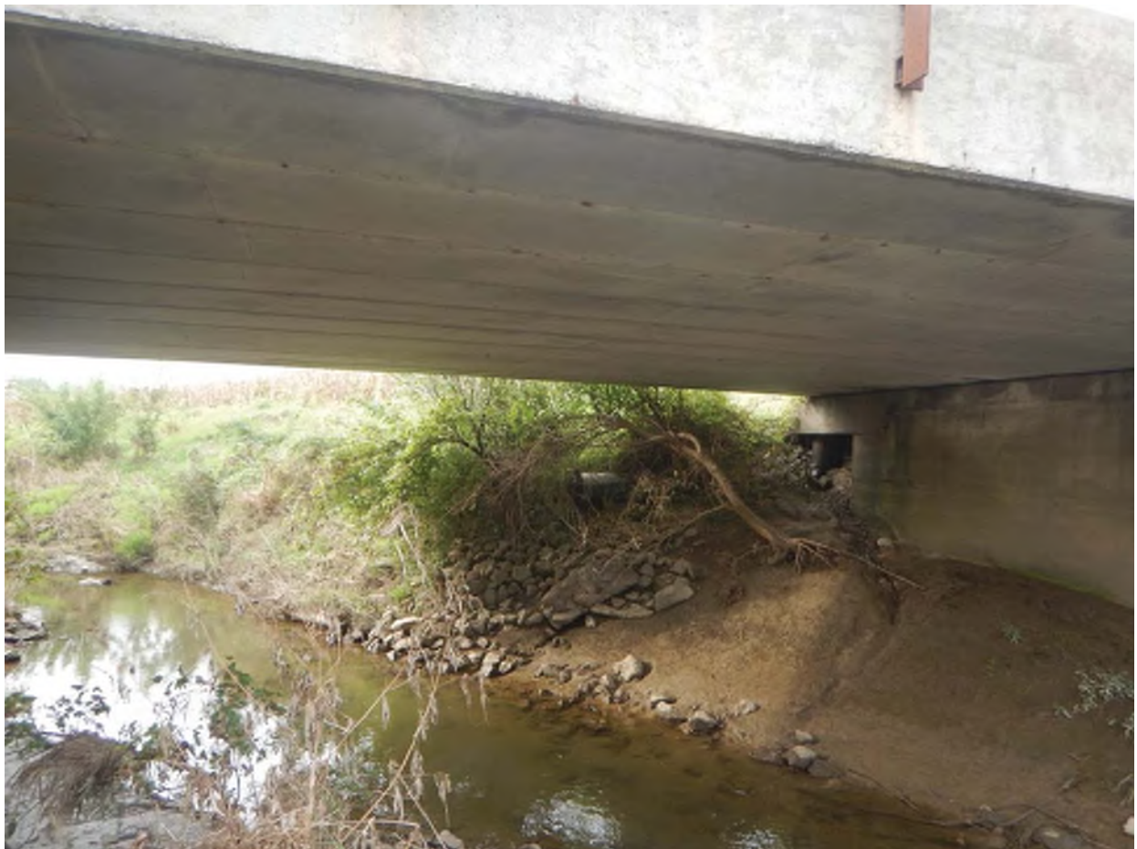
2. Facing southeast beneath bridge over Pollard Ditch
