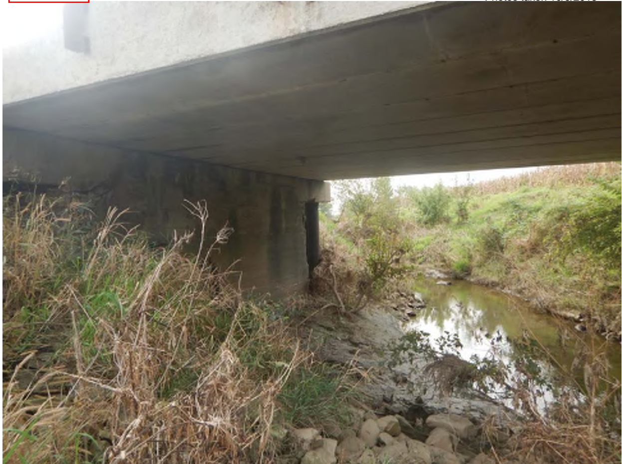
1. Facing southeast beneath bridge over Pollard Ditch
