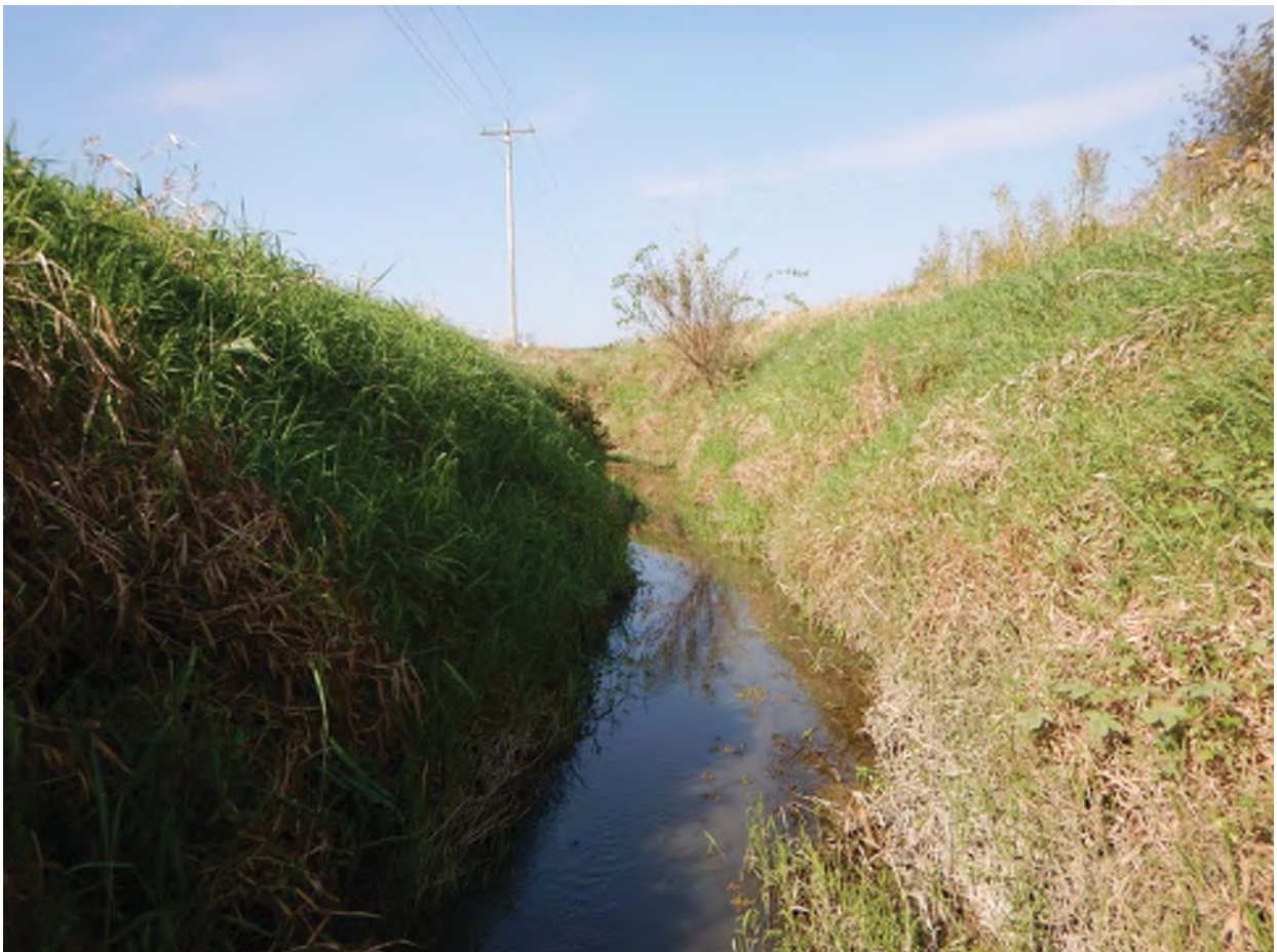
18. Facing west towards UNT to Pollard Ditch upstream from bridge
